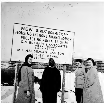
Future residents inspect progress on the new dorm.
