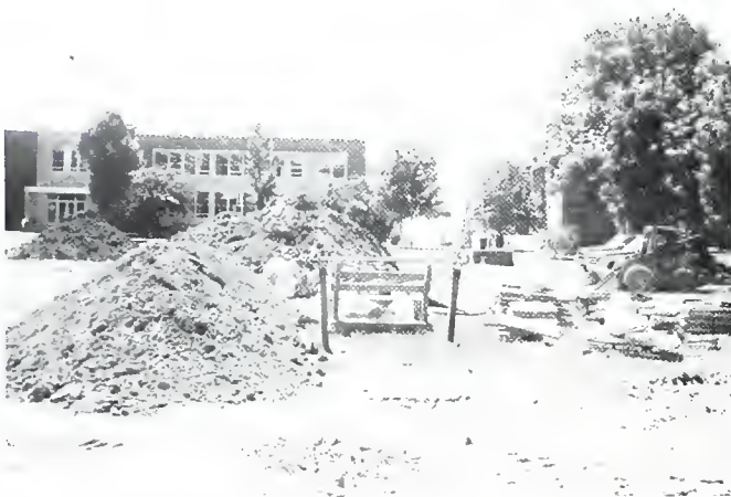
A number of renovations occurred over the past few years.
