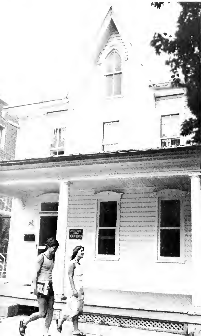
The old Health Center was demolished in 1989.
