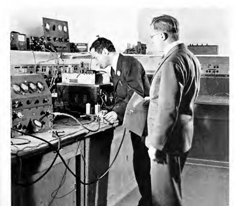
A DEVELOPMENTAL ULTRA-HIGH FRE-QUENCY TUBE IS TESTED BY RESEARCH SCIENTISTS IN AN ALL-COPPER SHIELDED ROOM AT RCA LABORATORIES.
