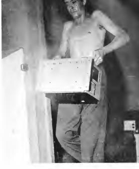
SHIPBOARD INTERCOMMUNICATION UNIT BEING BROUGHT FROM "TORTURE CHAM-BER'S" WEATHER ROOM, WHERE IT OPER-ATED IN 140-DEGREE HEAT.
