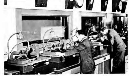
SOUND RECORDING EQUIPMENT WAS INSTALLED BY REA IN THE NEW YORK OFFICES OF OWI FOR USE IN OVERSEAS BROADCAST TRANSMISSIONS.
