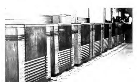
PRE-WAR TELEVISION RECEIVERS ROLLING OFF THE FINAL ASSEMBLY LINE AT THE CAMDEN, N. J., PLANT OF THE RCA VICTOR DIVISION. THEY WERE THE LARGEST MODELS TRK-12, BUILT BY RCA.
