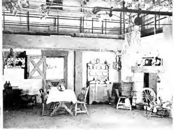
THESE STAGE SETS ILLUSTRATE THE VERSATILITY OF THE NEW UNIT STRUCTURE IN BUILDING WALLS, GOTHIC WINDOWS, DUTCH DOORS AND FIREPLACE OPENINGS. THE SAME UNITS ARE APPLIED IN VARIOUS WAYS ACCORDING TO THE DESIGN.
