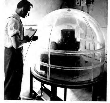
TECHNICIAN RECORDS OPERATING DATA FROM THE COMMUNICATIONS UNIT BEING TESTED IN THIS RECENTLY DEVELOPED ALTITUDE CHAMBER.
