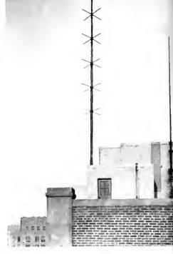
"TURNSTILE" ANTENNA USED WITH THE FM TRANSMITTER OF STATION WCAU, IN PHILAPELPHIA.
