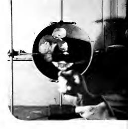
aspherical system, for projecting television images from cathode-ray tubes onto a viewing screen, was ready; special tubes were built for it, and the first demonstration was given at the Camden laboratory.
