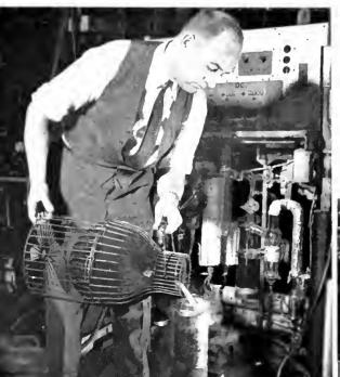
LIQUID AIR, TEMPERATURE 313 DEGREES BELOW ZERO, FAHRENHEIT, IS USED BY J. BURNETT TO IMPROVE THE VACUUM IN A TUBE WHEN IT IS COMPLETED. BELOW, II. A. FINKE TAKES PERFORMANCE DATA ON A RESEARCH TUBE AS IT IS PUT THROUGH ITS PACES IN AN ELABORATE SERIES OF ELECTRICAL TESTS.
