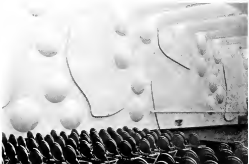
VIEWS OF NEW NBC STUDIO IN RADIO CITY SHOWING UNUSUAL FORMS OF WALL AND CEILING TREATMENT TO DIFFUSE SOUNDS AND PREVENT TONE-DESTROYING ECHOES. THE PATTERN OF ROUNDED SURFACES AND EMBOSSED PATCHES IS DIFFERENT FOR EACH WALL.
