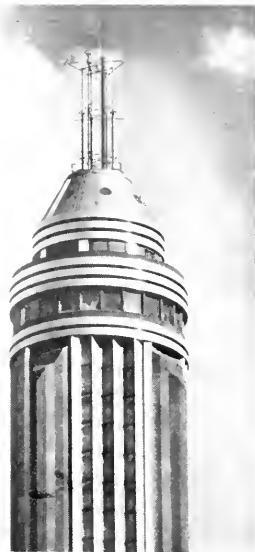
EARLIEST TYPE OF TELEVISION ANTENNA ERECTED ON THE EMPIRE STATE TOWER, BY RCA-NBC IN 1931.
