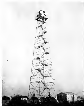
AUTOMATIC, UNATTENDED RADIO RELAY TOWERS, LIKE THE ONE ABOVE, MAY ULTIMATELY REPLACE THOUSANDS OF MILES OF TELEGRAPH AND TELEPHONE LINES IN THE UNITED STATES.
