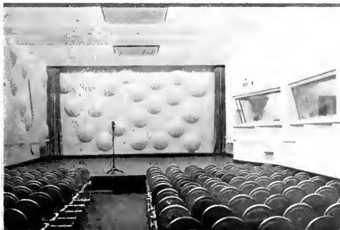
VIEWS OF NEW NBC STUDIO IN RADIO CITY SHOWING UNUSUAL FORMS OF WALL AND CEILING TREATMENT TO DIFFUSE SOUNDS AND PREVENT TONE-DESTROYING ECHOES. THE PATTERN OF ROUNDED SURFACES AND EMBOSSED PATCHES IS DIFFERENT FOR EACH WALL.
