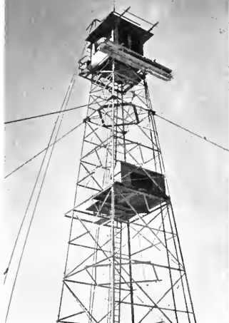
TOWERS SIMILAR TO THE ONE ABOVE SUPPORTED TELEVISION CAMERAS AND TRANSMITTERS ON BIKINI. AT RIGHT: "DRONE" PLANE CARRYING A TELEVISION CAMERA, COMES IN FOR A LANDING. OPERATOR IN FOREGROUND HAS TAKEN OVER CONTROL FROM THE "MOTHER" PLANE IN THE DISTANCE.
