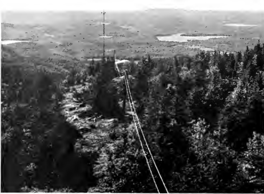
Coaxial transmission lines lead from central television receiving antenna on Mt. Belknap to Laconia, six miles away. At right: Close-up of Antenaplex tower on 2,400-foot mountain.
