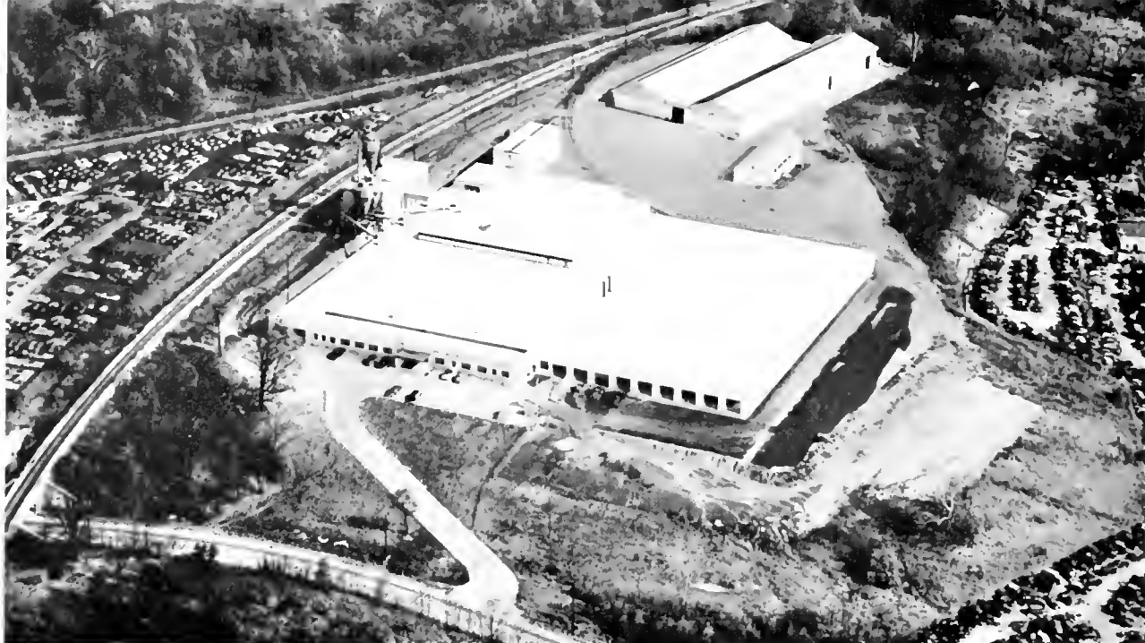
The new Cincinnati plant provides more than 135,000 square feet of floor space for the manufacture of miniature and sub-miniature electron tubes.
