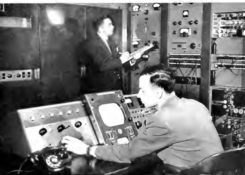
FROM THIS TOWER NEAR BRIDGEPORT, CONN., RCA-NBC HAVE BEEN CONDUCTING EXTENSIVE FIELD TESTS OF TELEVISION PROGRAMS TRANSMITTED ON ULTRA-HIGH FREQUENCIES. BELOW: CONTROL CONSOLE AND TRANSMITTER SWITCHBOARD AT BRIDGEPORT STATION.
