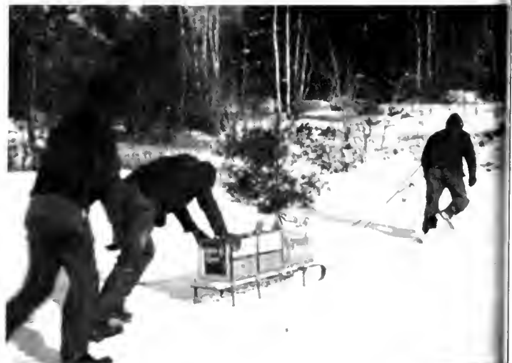
10 RADIO AGE Workmen drew hundreds of pounds of TV equipment up last half-mile of roadless, snow-covered mountain.
