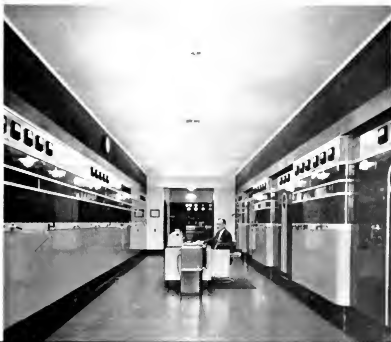
Three RCA transmitters line the walls of the main floor of NBC's International station.
