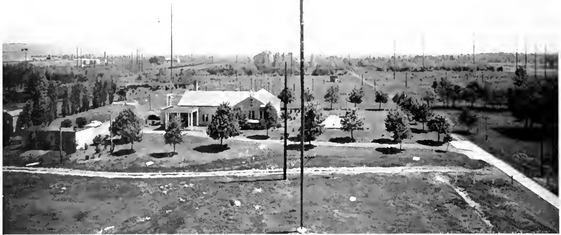
NBC's East Coast transmitter building at Bound Brook, N. J., is surrounded by a forest of poles supporting the station's array of shortwave antennas.
