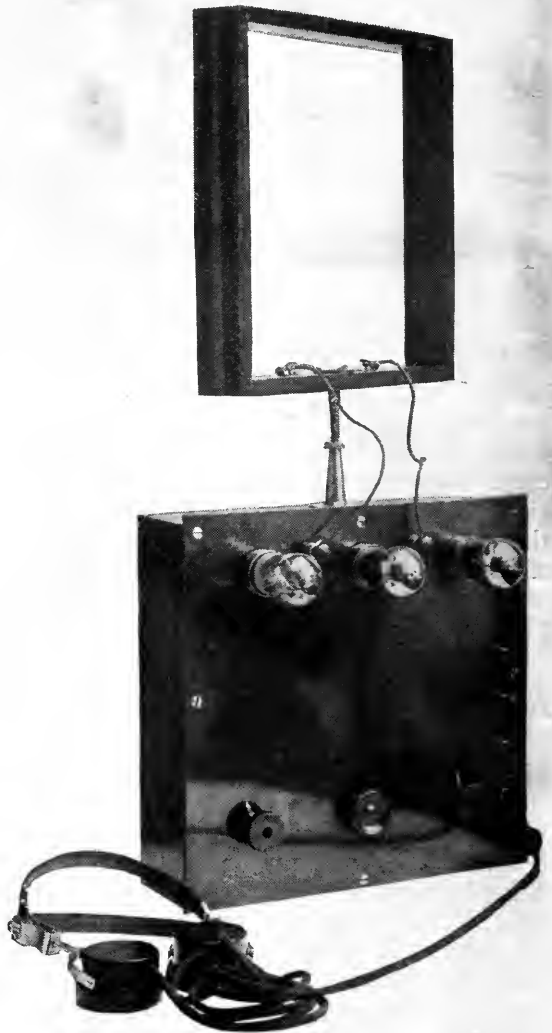
THE COMPLETE "INVERSE DUPLEX" RECEIVER
