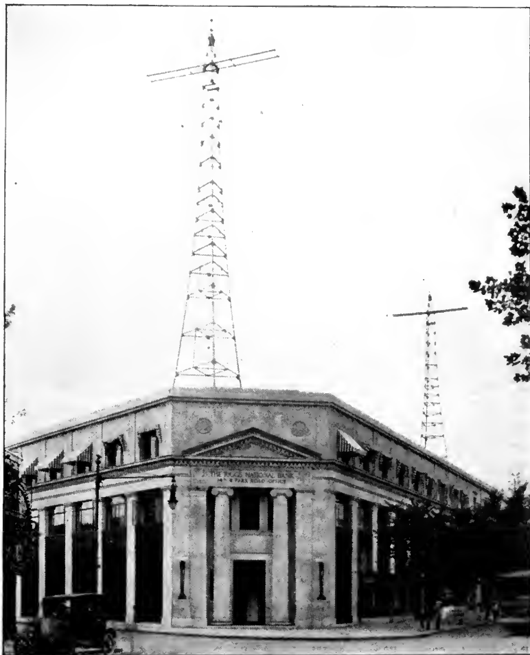
THE AERIAL WIRES ARE 150 FEET ABOVE THE STREET LEVEL
