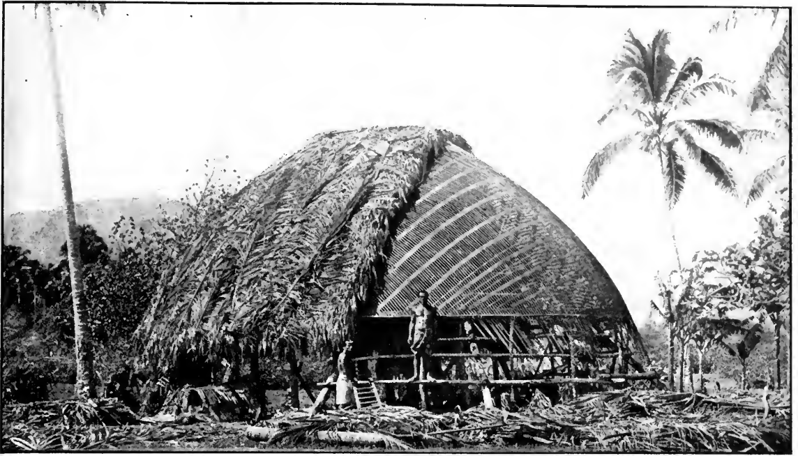
NATIVE SAMOANS PUTTING THE ROOF ON THEIR HOUSE
