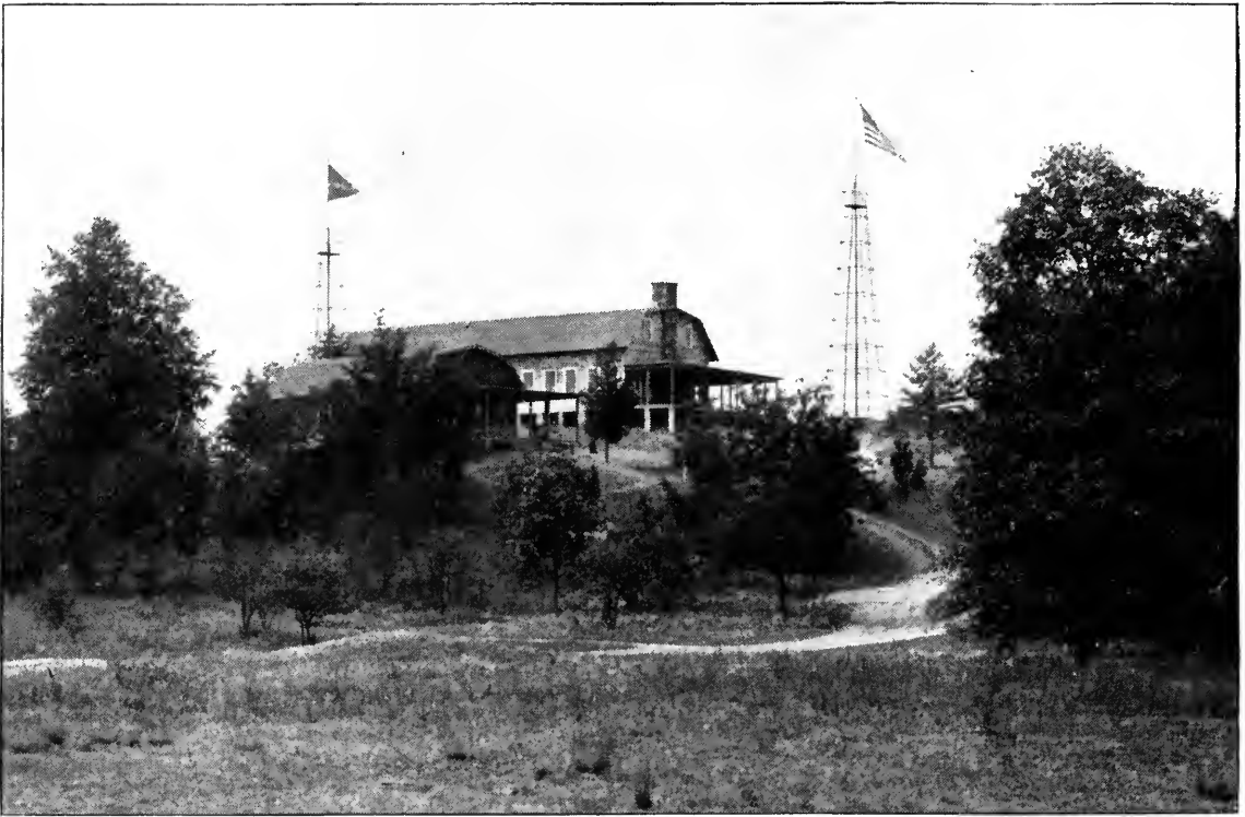
THE WIRELESS TOWERS AND RECREATION BUILDING AT CAMP WALKKILL, NEAR LAKE MOHAWK, N. Y.
