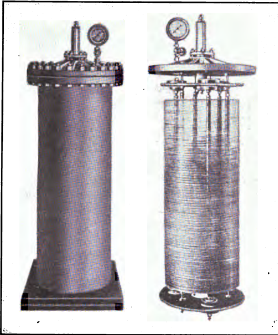
FIG. 88.—Compressed-air condenser.
