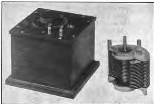
FIG. 87.—Variable air condenser.
