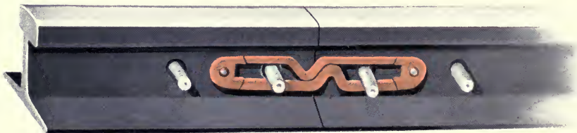
Showing a Type U. P.-01 United States Bond Installed on a Rail
