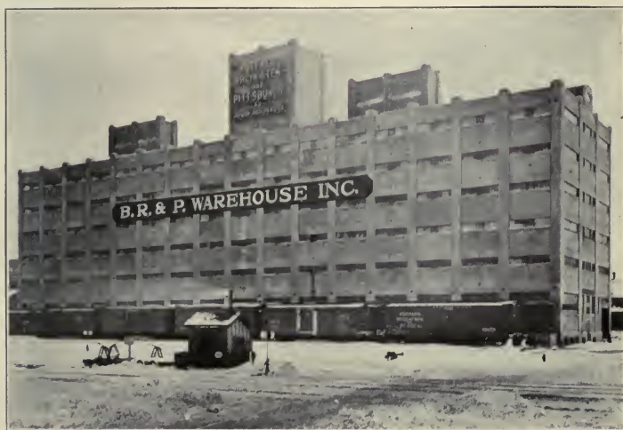
NEW FREIGHT TERMINAL WAREHOUSE AT ROCHESTER Built by the Buffalo, Rochester, & Pittsburgh Railway. A modern combination of freight house and storage warehouse.
