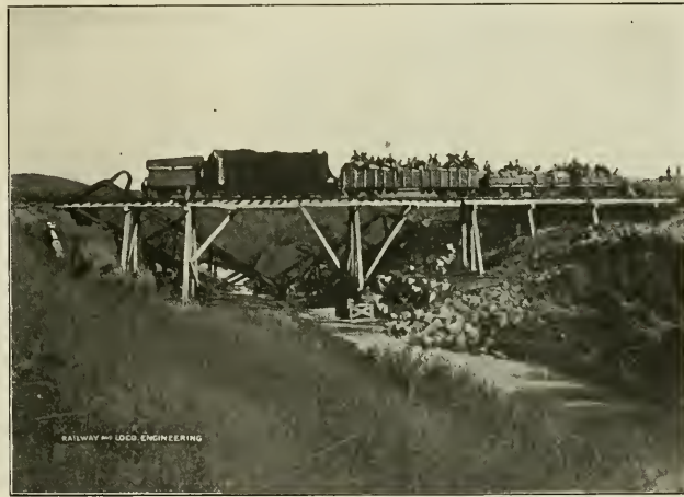
SOUTH AFRICA--ARMORED TRAIN ON TEMPORARY TRESTLE. WRECK OF STEEL BRIDGE SHOWING BEYOND.
