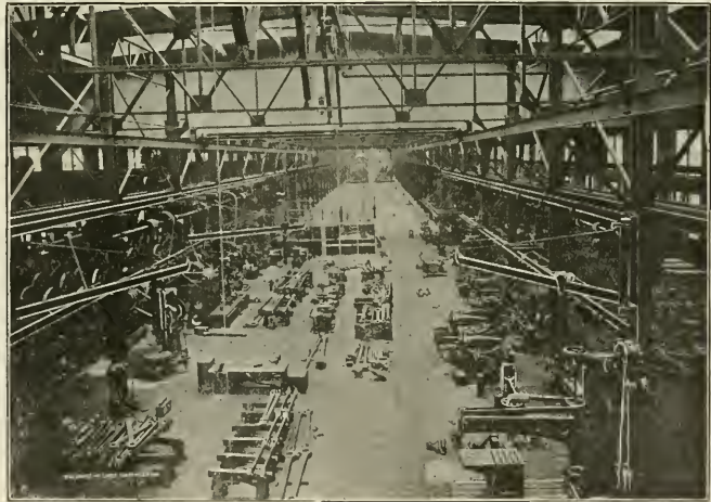
GENERAL VIEW OF THE MACHINE SHOP, CAN. PAC. RY., WINNIPEG, MAN.
