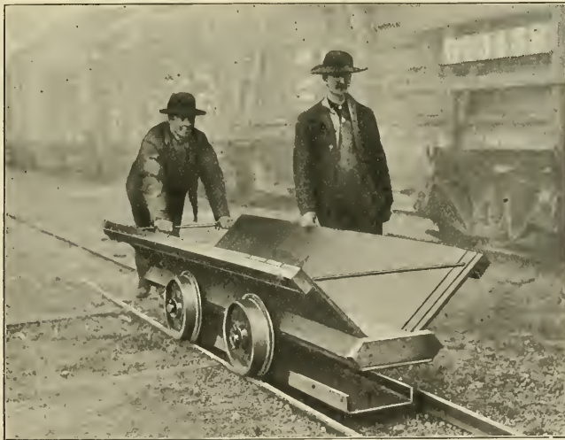
FIG 3. TRANSFORMED INTO A TRAVELING SCRAP RECEPTACLE
