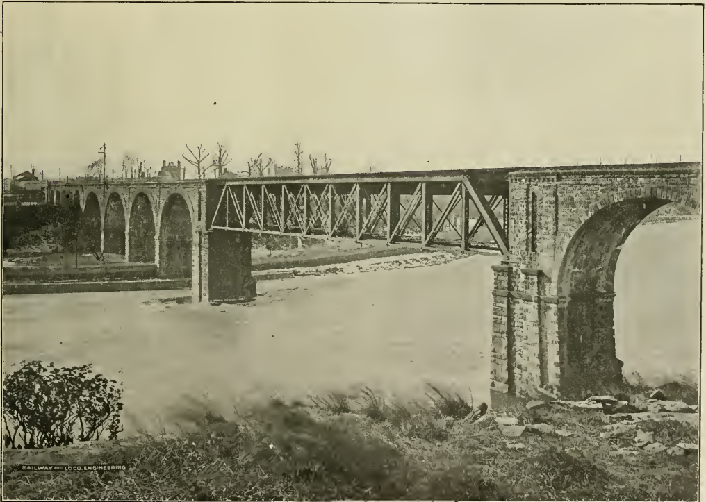
BRIDGE OVER THE SCHUYLKILL RIVER AT PHILADELPHIA ON THE PENNSYLVANIA RAILROAD.
