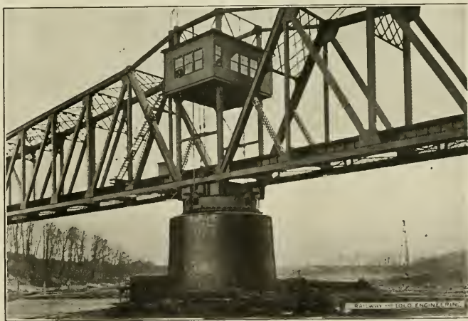
EXAMPLE OF SWING BRIDGE SHOWING TURNTABLE AND CENTER PIER. BRIDGE MUST OPEN FULLY FOR EVERY VESSEL
