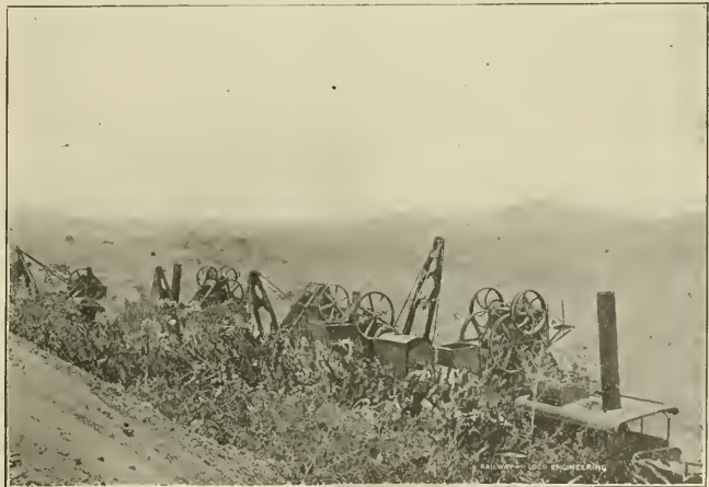
OLD FRENCH MACHINERY ABANDONED ALONG THE CANAL ROUTE.
