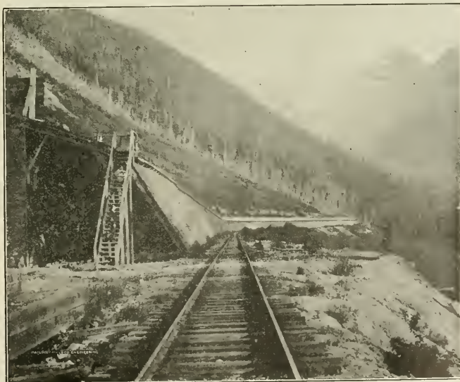
SNOW SHED, WITH SUMMER TRACK OUTSIDE, SHOWING PATH OF SNOW SLIDE WHERE TREES HAVE BEEN SWEEP AWAY.
