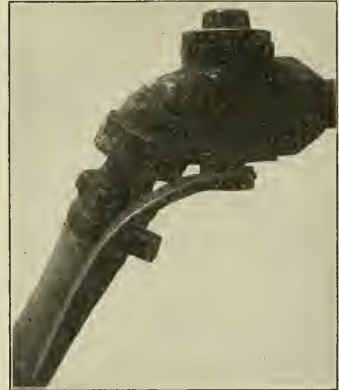
ANGLE VALVE—HOSE PROTECTING HANDLE.
