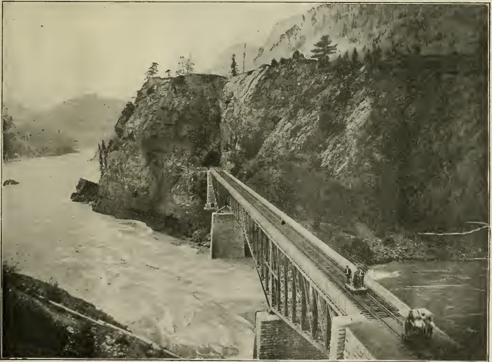
CANTILEVER BRIDGE OVER THE FRASER RIVER, C. P. R., BRITISH COLUMBIA.
