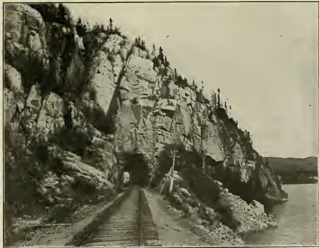
JACK FISH TUNNEL, NORTH SHORE OF LAKE SUPERIOR, ON THE CANADIAN PACIFIC RAILWAY.
