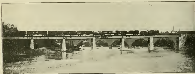
STEEL GIRDER AND BRICK ARCH RAILWAY BRIDGES
