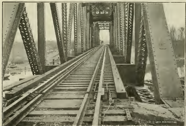
INTERIOR OF SWING SPAN, SHOWING CONTACT FOR ELECTRIC SIGNAL CIRCUIT.
