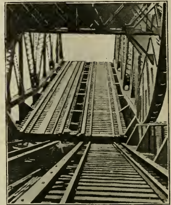
INTERIOR VIEW, BRIDGE PARTLY RAISED.
