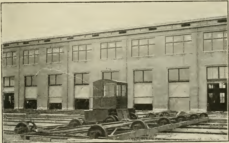
TRANSFER TABLE, MISSOURI PACIFIC SHOPS, SEDALIA, MO., SHOWING DOUBLE DROP DOORS AND WINDOW ARRANGEMENT. Courtesy of the New Southwest .
