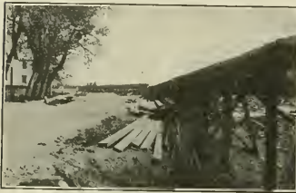
MAKING A FILL
