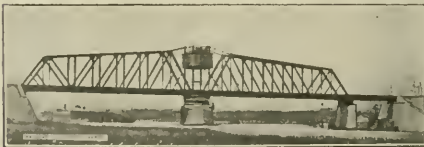
BLACK RIVER SWING, ON THE NICKEL PLATE. CANTILEVER FOR THE DEAD LOAD, CONTINUOUS GIRDER FOR THE LIVE LOAD.
