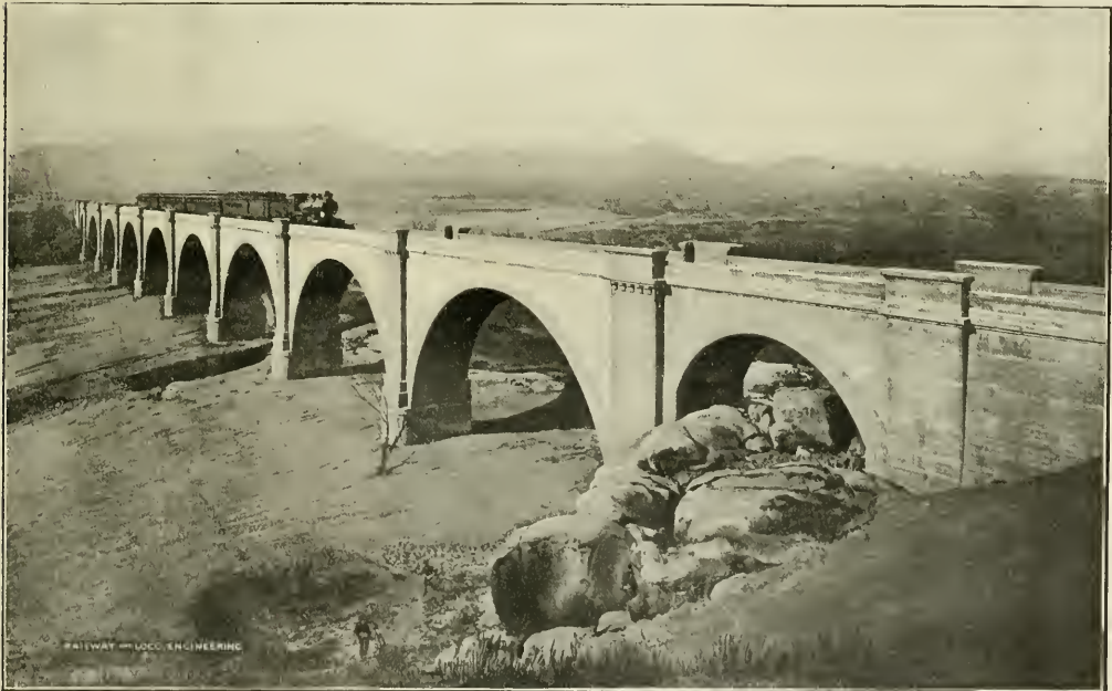
CONCRETE VIADUCT OVER THE SANTA ANA RIVER, IN CALIFORNIA
