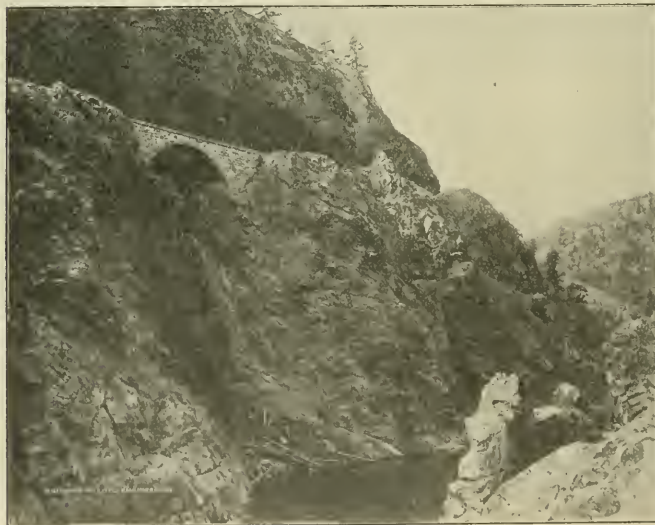
STONE ARCH USED IN MODERN RAILWAY WORK
