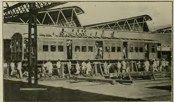
No. 2—TAKEN AT 8.20 A. M. WEDNESDAY—WORK IN PROGRESS.
