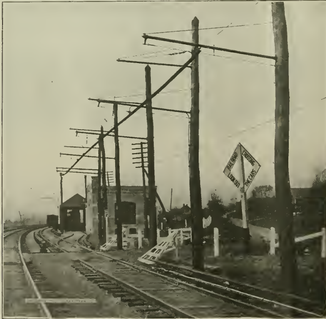
TEST TRACK FOR N. Y. C. ELECTRIC LOCOMOTIVES SHOWING THIRD RAIL ALONG THE LINE AND OVERHEAD CONTACT FOR HIGHWAY CROSSINGS
