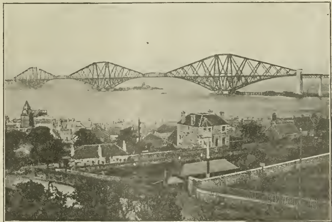
CANTILEVER BRIDGE OVER THE FIRTH OF FORTH FROM THE TOWN OF LEITH, SCOTLAND.
