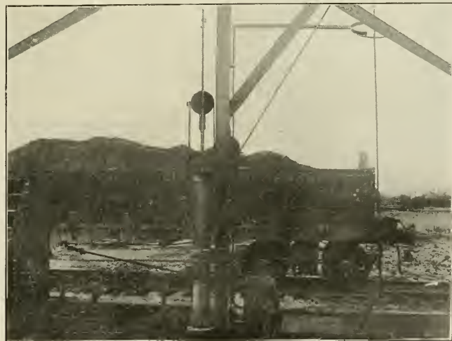
FIG. 4. ASHPIT CRANE MOVING ASH CAR INTO POSITION.
