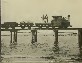
BUILDING THE JETTY AT BANDON, ORE. TIDE COMING IN.
