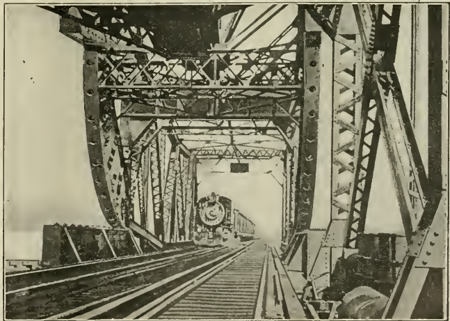
TRAIN PASSING THROUGH ROLLER BRIDGE, C. R. R. OF N. J.
