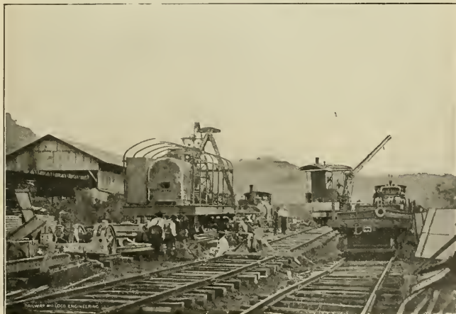
ERECTING A STEAM SHOVEL ON THE GROUND.
