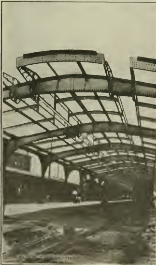
STEEL TRAIN SHED UNDER CONSTRUCTION.
