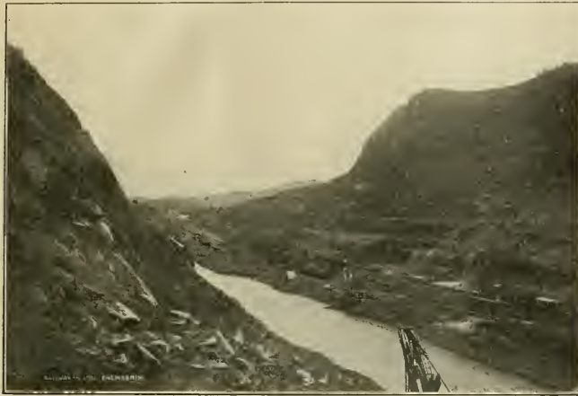
CULEBRA CUT LOOKING NORTH. PANAMA CANAL.
