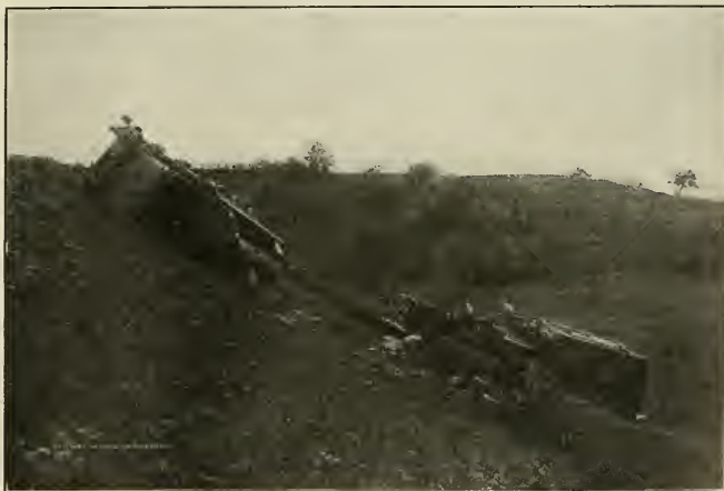
RESULT OF DEFECTIVE TRACK. SCENE SHOWS HEDGEROWS USED INSTEAD OF FENCES IN ENGLAND.
