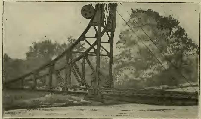
ERIE LIFT BRIDGE, WITH COMPENSATING WEIGHT.
