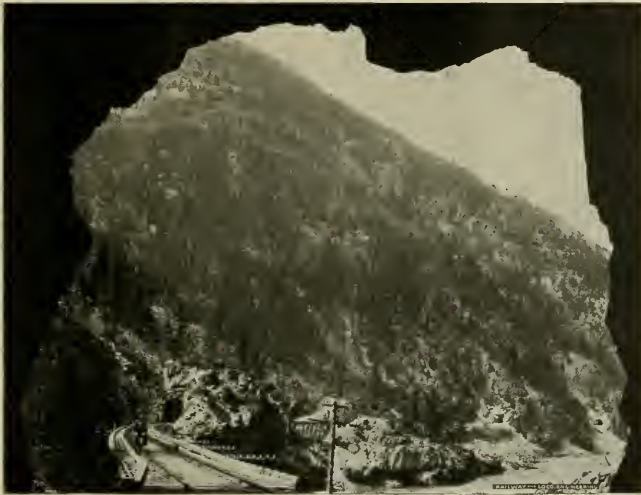
VIEW TAKEN FROM INTERIOR OF ONE TUNNEL SHOWING OPENING OF THREE OTHERS. FRASER CANYON, B. C.
