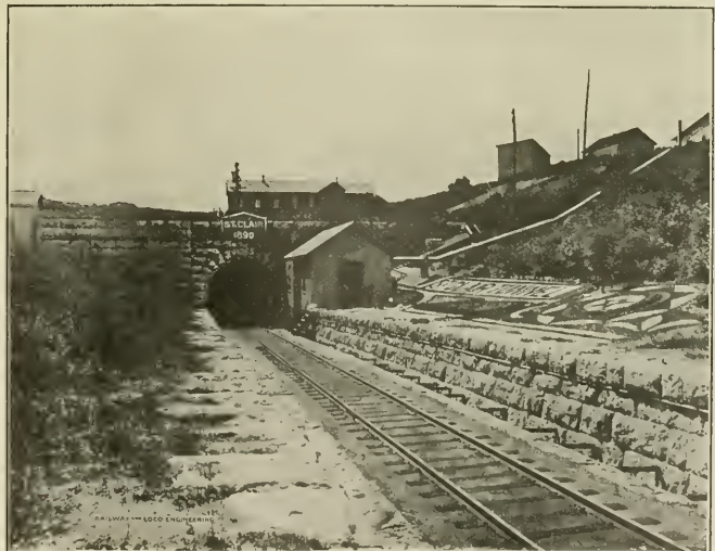
SOUTH PORTAL OF THE ST. CLAIR RIVER TUNNEL.
