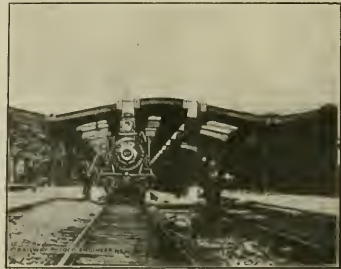
SMOKE STACK BELOW SMOKE DUCT.
