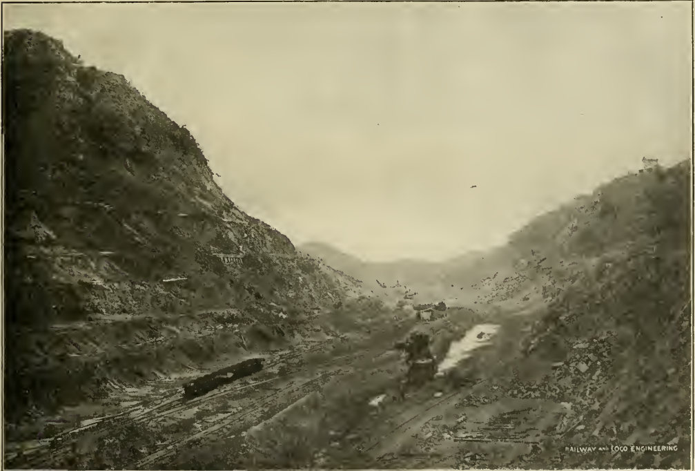
CULEBRA CUT, THE LARGEST EXCAVATION ON THE ROUTE OF THE PANAMA CANAL.
