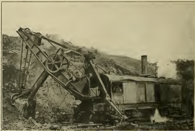
MODERN STEAM SHOVEL CUTTING DOWN A BANK.
