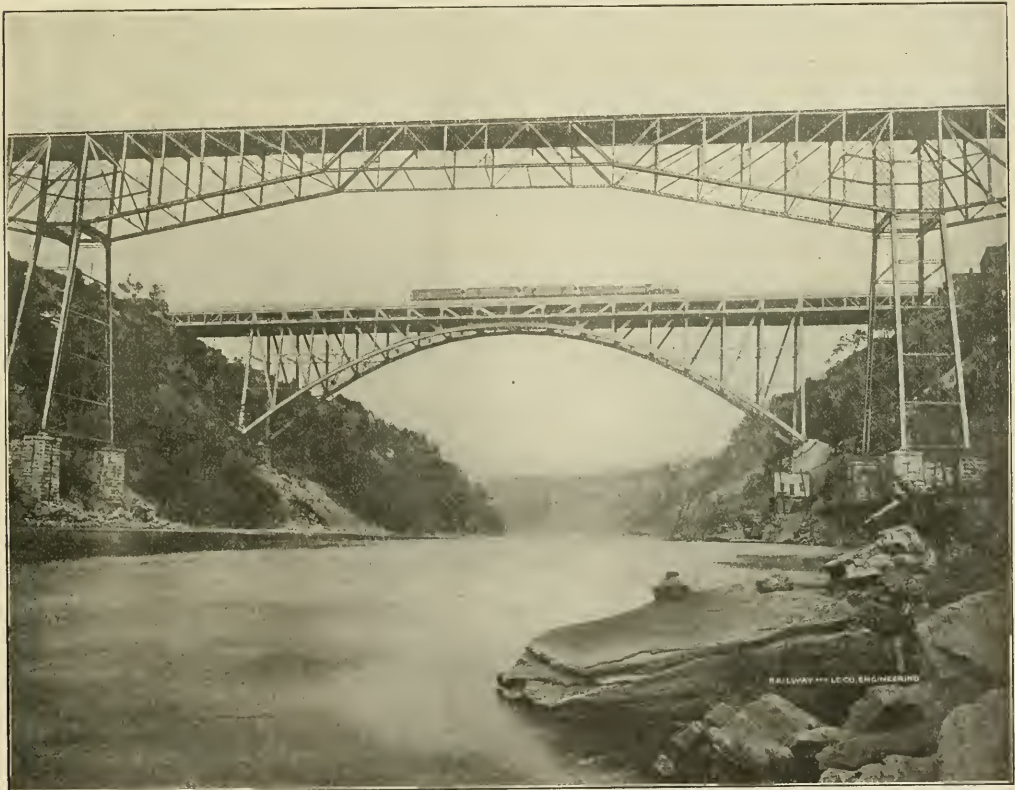
RAILROAD BRIDGES OVER THE NIAGARA GORGE. THE CANTILEVER AND THE STEEL ARCH
