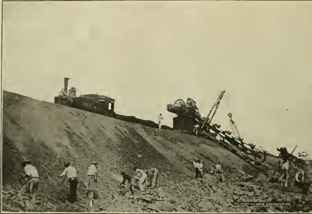
OLD FRENCH EXCAVATOR AT WORK.
