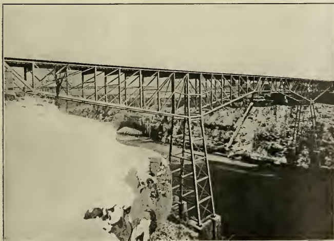
DOUBLE TRACK CANTILEVER BRIDGE OVER THE NIAGARA GORGE.
