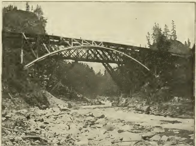
STEEL ARCH REPLACING SPIDER-LEGGED WOODEN STRUCTURE
