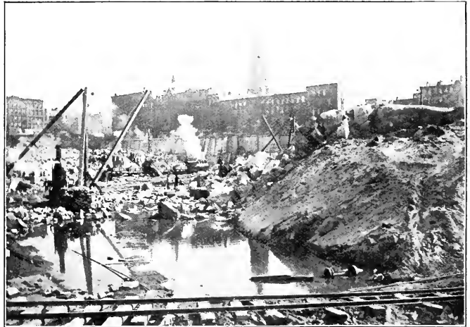
EXCAVATING FOR THE PENNSYLVANIA TERMINAL, NEW YORK CITY.
