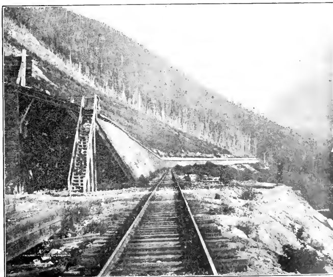
SNOW SHED. WITH SUMMER TRACK OUTSIDE, SHOWING PATH OF SNOW SLIDE WHERE TREES HAVE BEEN SWEEPED AWAY.
