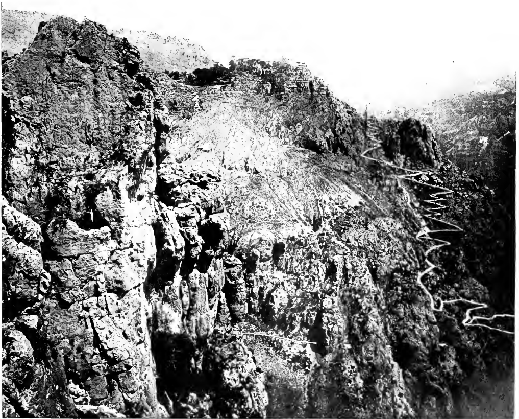
IN THE MARITIME ALPS—SCENE TYPIFYING WHAT A RAILWAY LOCATING ENGINEER MAY ENCOUNTER.
