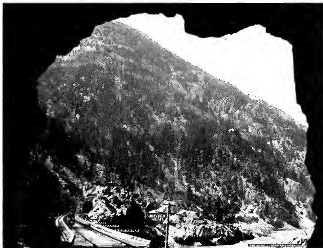
VIEW TAKEN FROM INTERIOR OF ONE TUNNEL SHOWING OPENING OF THREE OTHERS. FRASER CANYON, B. C.
