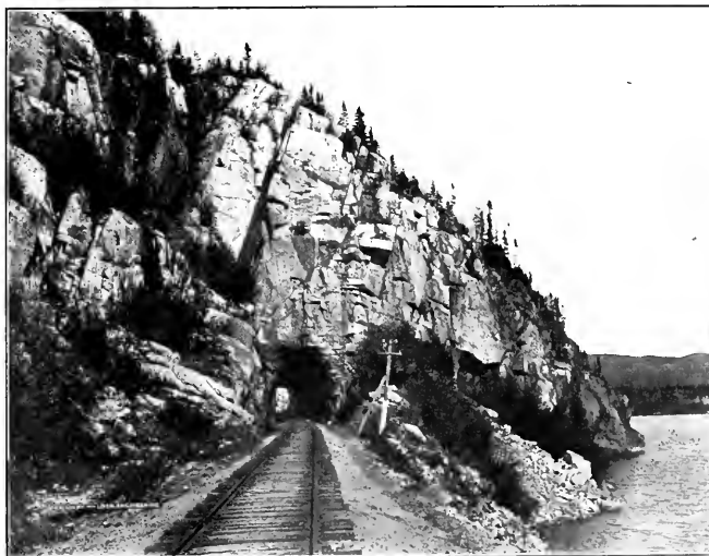
JACK FISH TUNNEL, NORTH SHORE OF LAKE SUPERIOR, ON THE CANADIAN PACIFIC RAILWAY.
