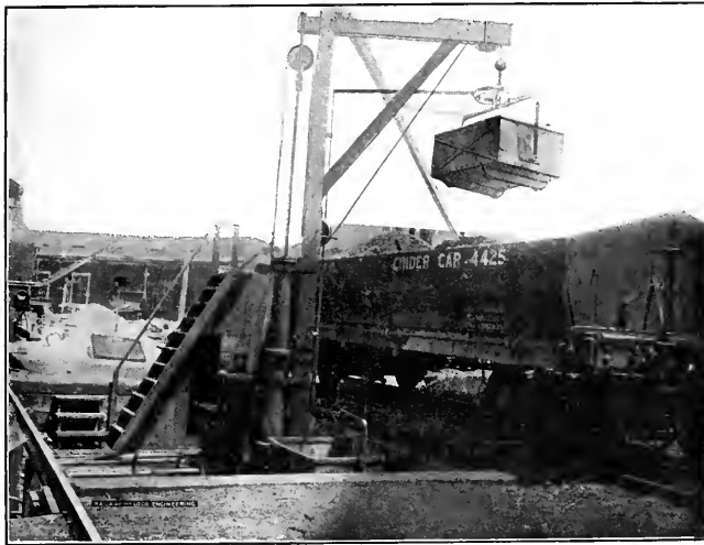
FIG. 3. ASH BUCKET OVER CAR READY FOR DUMPING.
