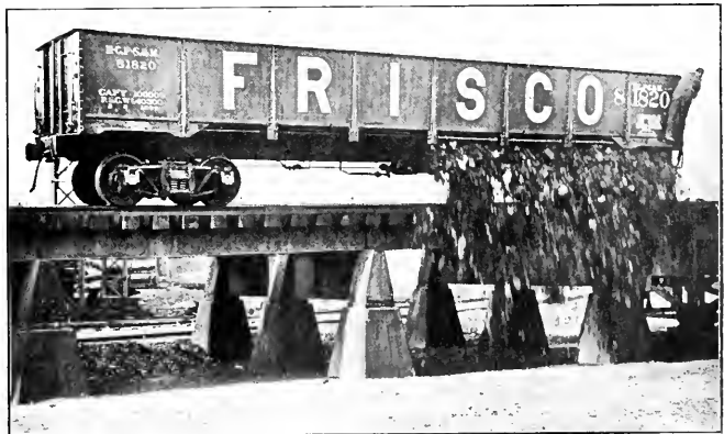
GENERAL SERVICE GONDOLA UNLOADING COAL.
