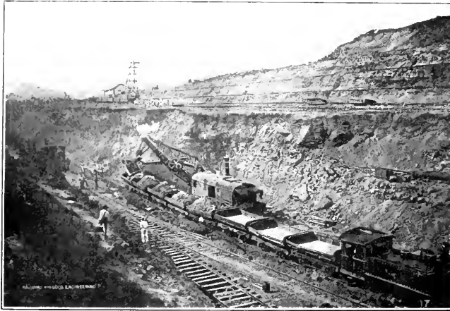
METHOD OF DOING THE WORK ON THE PANAMA CANAL.
