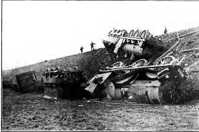
RESULT OF DEFECTIVE TRACK ON AN ENGLISH RAILWAY.
