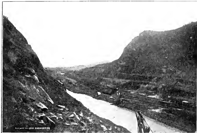
CULEBRA CUT LOOKING NORTH. PANAMA CANAL.
