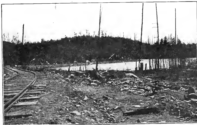
32-IN. GAUGE ROAD WITH FIVE PER CENT. GRADE BETWEEN LAKES, LAKE OF BAYS RAILWAY, ONTARIO.
