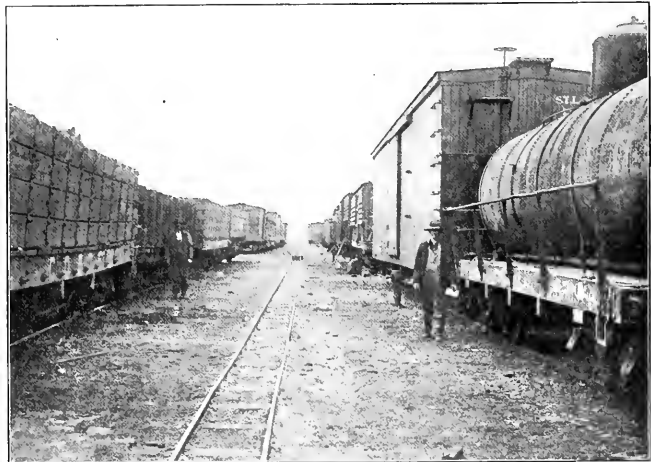
CAR REPAIR TRACKS WITH 20-INCH TRACK FOR DOLLY TRUCK
