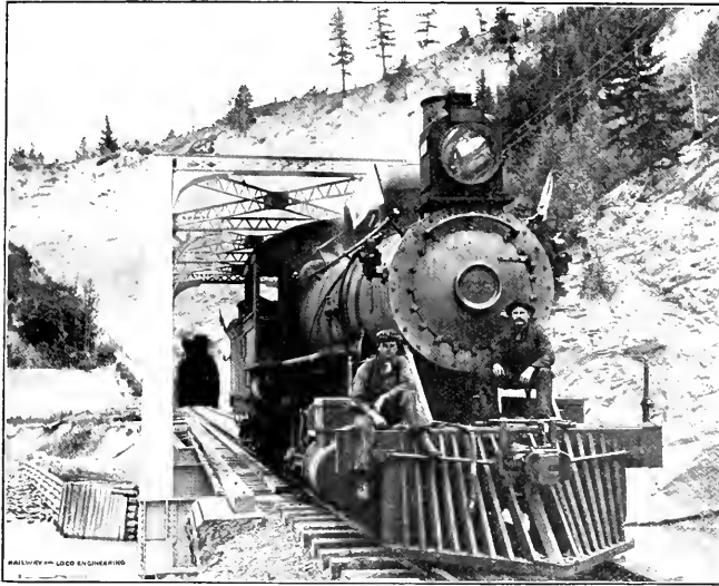
PUSHER ENGINE AND TUNNEL, IN THE ROCKY MOUNTAINS. CAN. PAC. RV.
