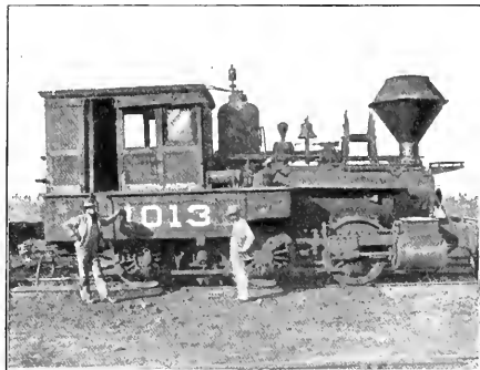
OLD, TIME CENT. PAC. WITH FIRE PUMP AND HOSE REEL
