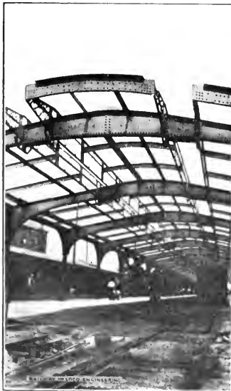
STEEL TRAIN SHED UNDER CONSTRUCTION.
