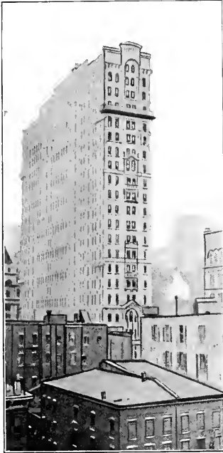
BACK OF TRINITY BUILDING. (From Office of Ry. and Loco. Engineering.)
