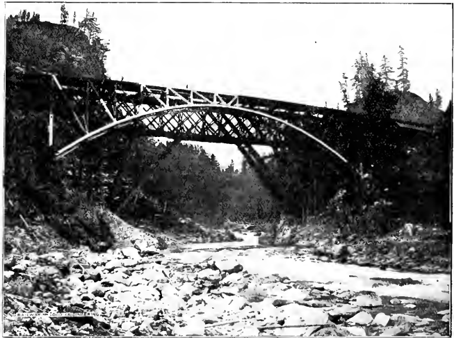
STEEL ARCH REPLACING SPIDER-LEGGED WOODEN STRUCTURE
