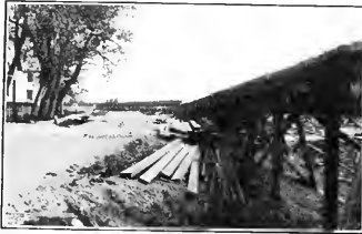
MAKING A FILL
