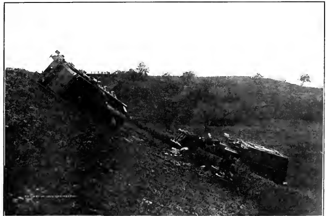
RESULT OF DEFECTIVE TRACK. SCENE SHOWS HEDGEROWS USED INSTEAD OF FENCES IN ENGLAND.
