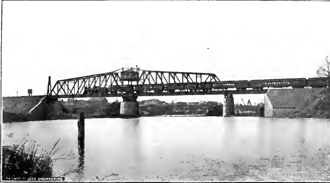
BLACK RIVER SWING BRIDGE ON THE NICKEL PLATE LINE.
