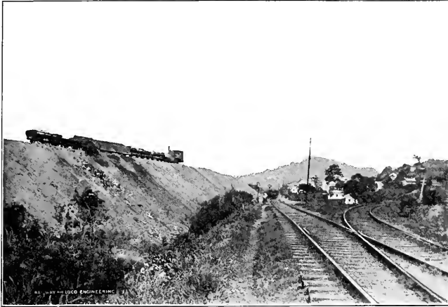
DISPOSING OF MATERIAL TAKEN FROM THE CANAL.
