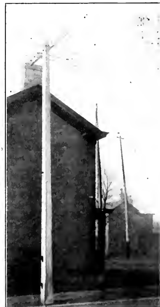
CONCRETE TELEGRAPH POLE.
