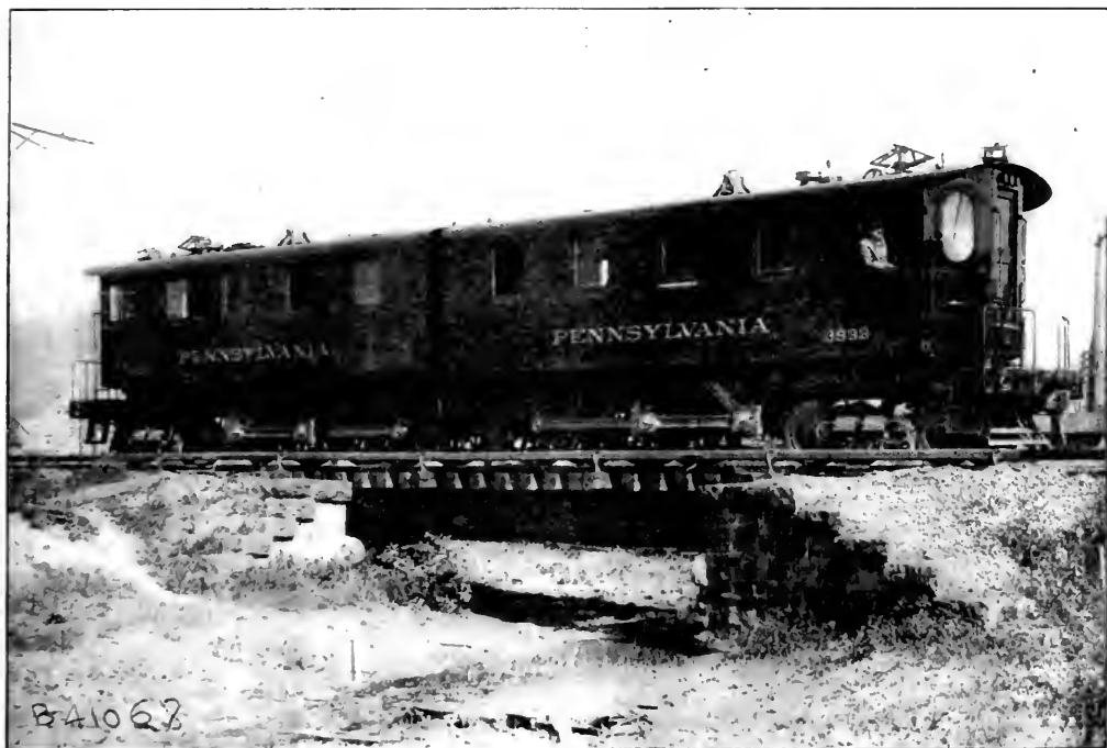
ELECTRIC LOCOMOTIVE FOR THE PENNSYLVANIA TUNNEL SERVICE
