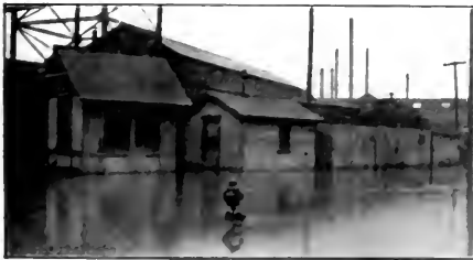
HIGH WATER AT YOUNGSTOWN, PA., YARD.
