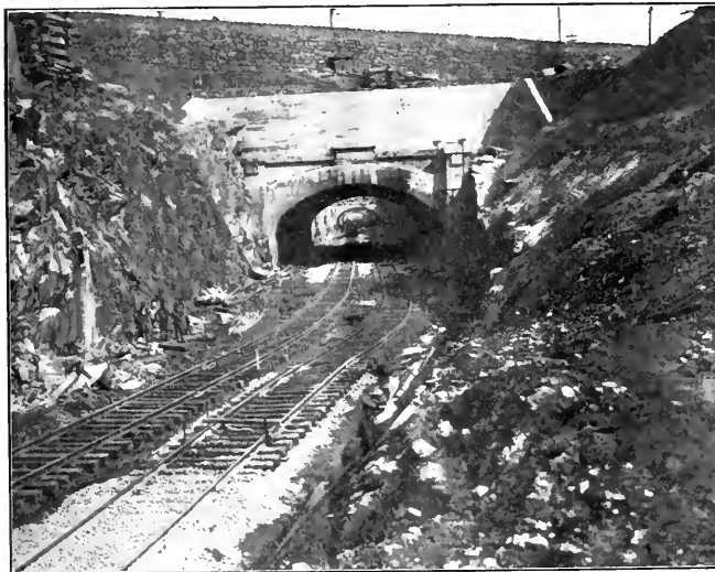
VIEW SHOWING PROGRESS OF THE WORK, TAKEN AT TRACK LEVEL.
