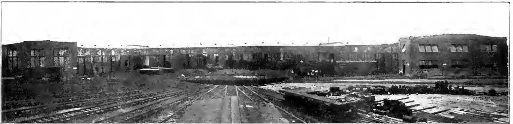
CENTRAL OF GEORGIA RAILROAD. ROUNDHOUSE AT MACON, GA.
