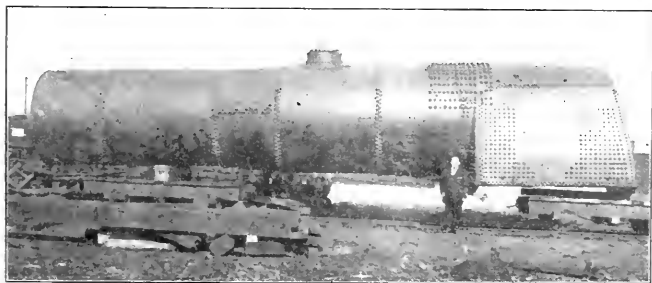
BOILER OF D. H. MALLETT COMPOUND.
