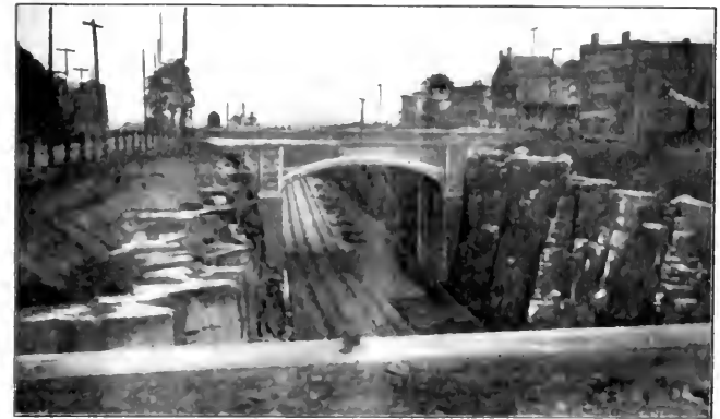
CONCRETE BRIDGE CARRYING STREET ACROSS THE OPEN CUT.
