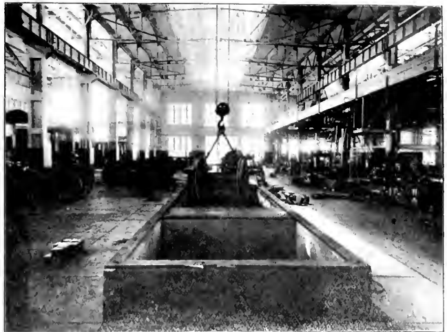
VENTILATED LYE VAT, ERISCO SHOPS AT SPRINGFIELD, MO.
