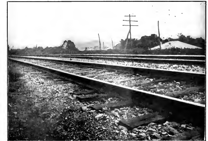
STANDARD ROCK BALLAST TRACK, C. & O.
