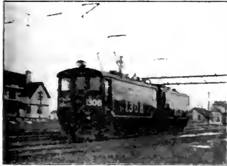
ST. CLAIR TUNNEL LOCOMOTIVE.
