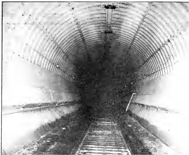
INTERIOR OF THE ST. CLAIR TUNNEL SHOWING LIGHTING SYSTEM.
