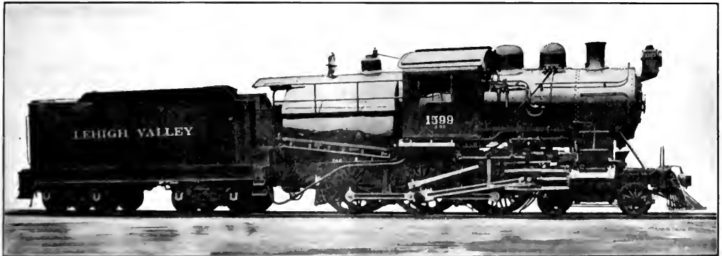
TEN-WHEEL PASSENGER LOCOMOTIVE FOR THE LEHIGH VALLEY.
