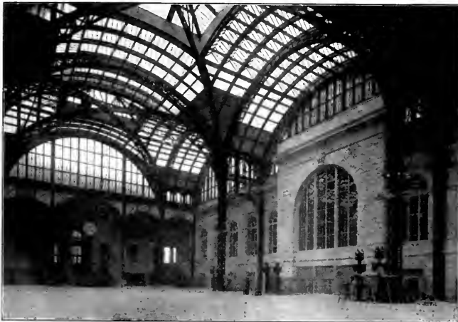
THE CONCOURSE, P. R. R. STATION IN NEW YORK.
