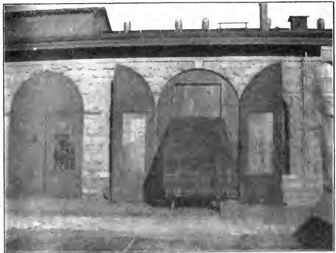
FIG. 2. STORM DOOR OPEN, SET OF FLUES IN PLACE.
