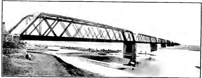
RAILWAY BRIDGE OVER THE FUGI RIVER, JAPAN.
