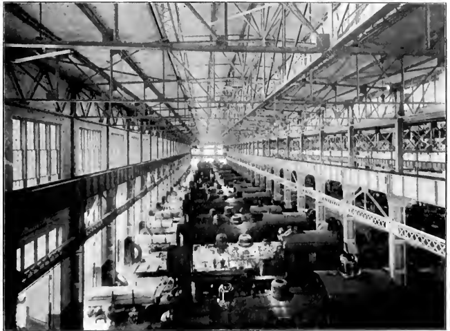
VIEW OF ERECTING SHOP, FRISCO SYSTEM, SPRINGFIELD, MO
