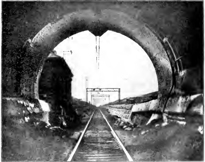
LOOKING OUT OF THE TUNNEL UP THE TRACK TO PORT HURON.
