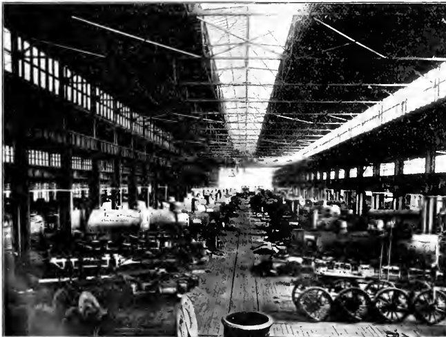
RECTING SHOP, C. R. I. & P. REPAIR PLANT AT SILVIS, ILL.
