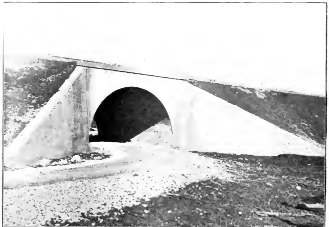
CONCRETE ARCH OVER HIGHWAY, SOUTHERN RAILWAY.
