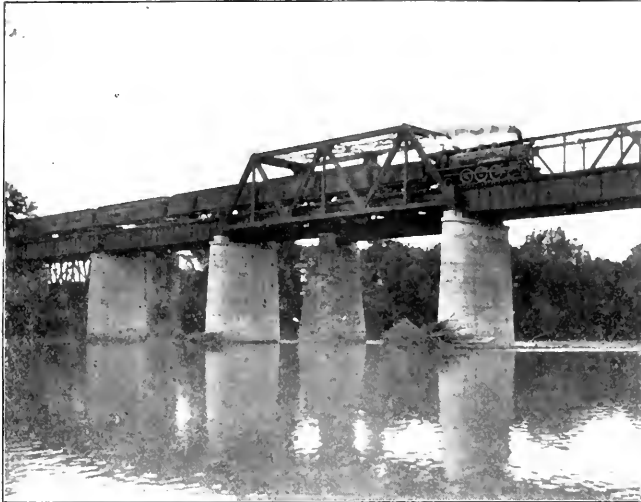
NEW AND OLD HOLSTON RIVER BRIDGES AT STRAWBERRY PLAINS, TENN.
