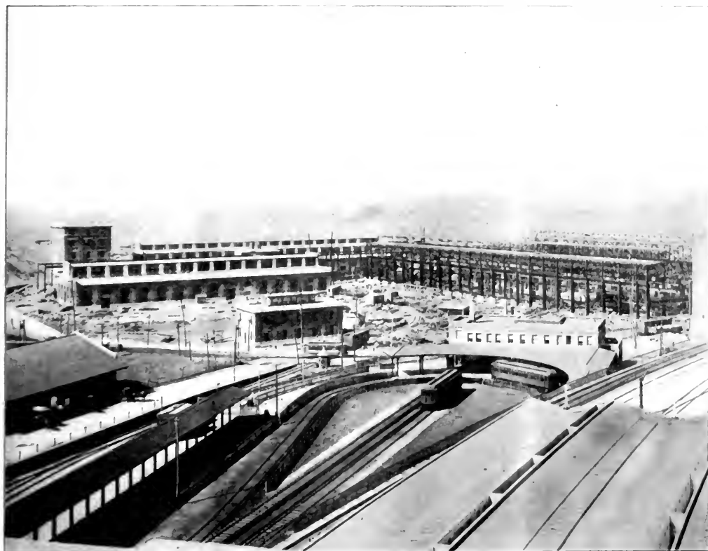
GENERAL VIEW, BEFORE COMPLETION, OF THE D. L. & W. SHOPS AT SCRANTON, PA.
