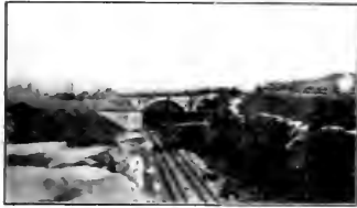
VIEW SHOWING PROGRESS OF WORK.
