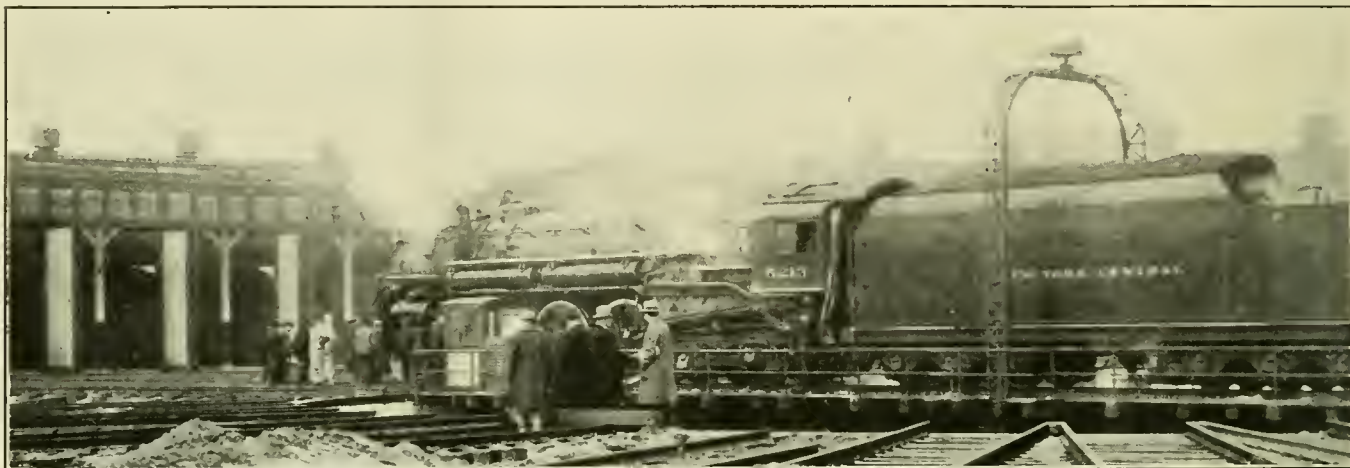
New 100 Foot Turntable of the New York Central Lines at Harmon, N. Y.
