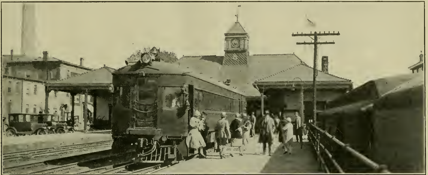
Branch Line Terminal Showing Gas-Electric Car in Service
