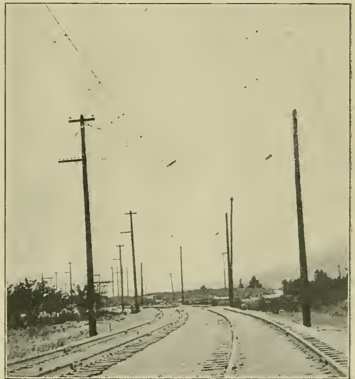
Catenary Cross Span Construction on Great Northern Electrification
