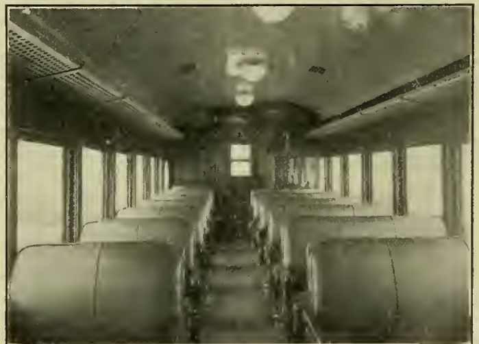
Passenger Compartment of Gas-Electric Car
