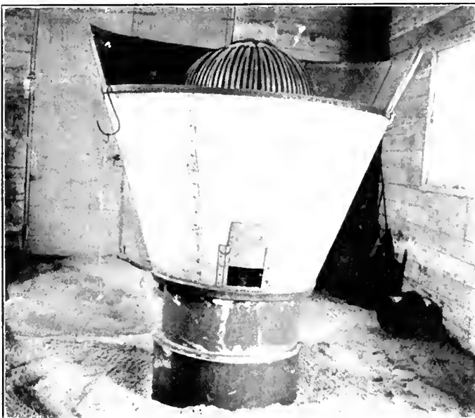
A Novel Dryer for Locomotive Sand
