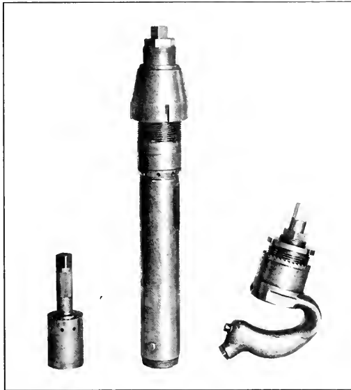
Fig. 14—Tools for Facing Air Hammer Connections
