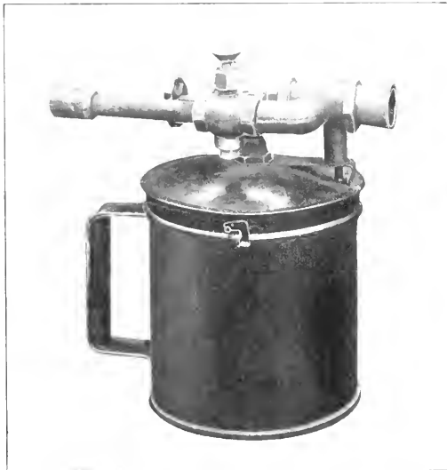
Vacuum Paint Sprayer for Railroad Work
