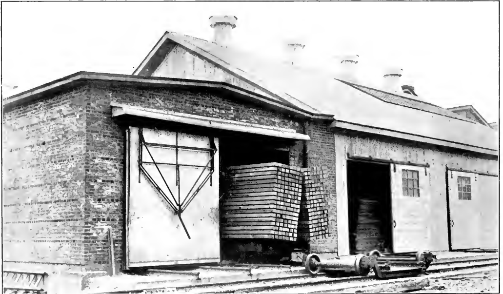
Front View of the Norfolk & Western Dry Kiln
