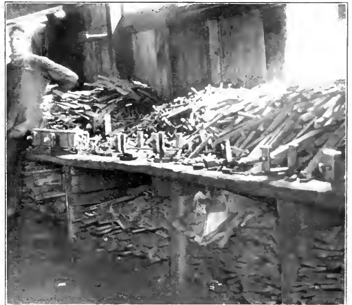
Fig. 3—Piling Bench at St. Cloud Rolling Mill
