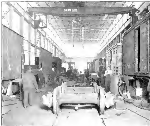
Steel Car Bay in the Car Repair Shop
