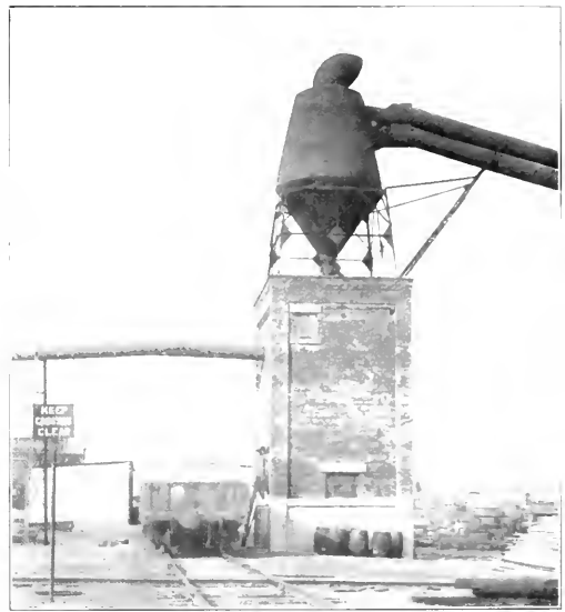
Sawdust House and Separator for Planing Mill
