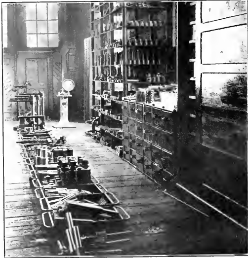
Stock Racks and Material in Process of Manufacture
