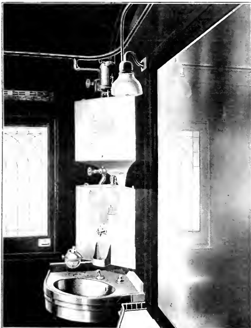
Sanitary Drinking Fountain Applied to a Passenger Car
