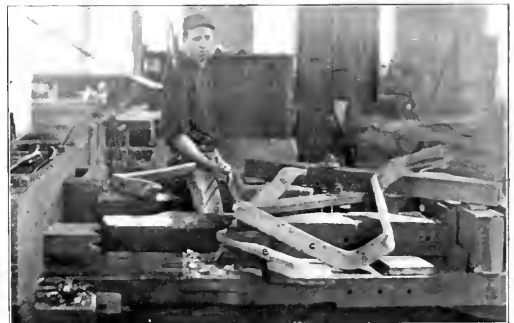
Fig. 14—Formers for Making Brake Mast Supports
