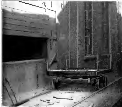
Fig. 2—Rotary Car on Which Tubes Are Carried to the Rattler
