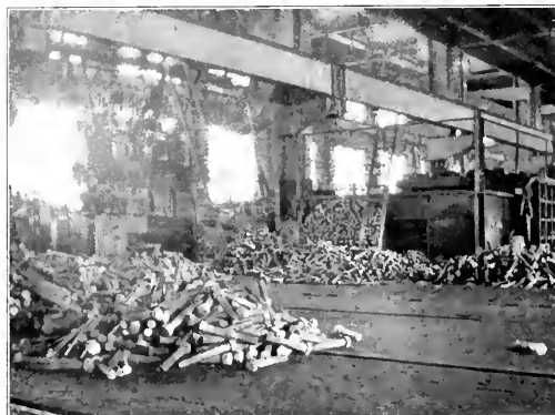
Rough Bolts Ready to Be Pointed
