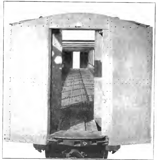
An End View of the Steel Work
