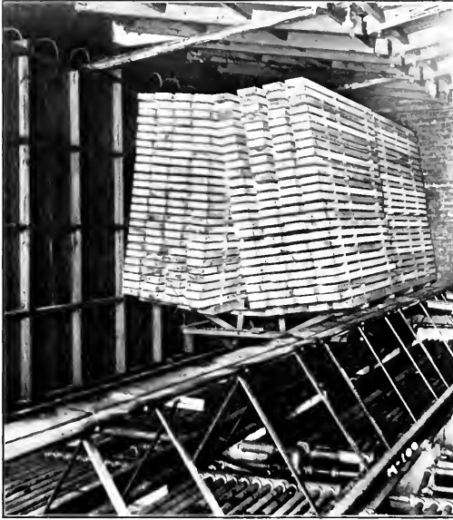
Interior of Humidity Controlled Dry Kiln
