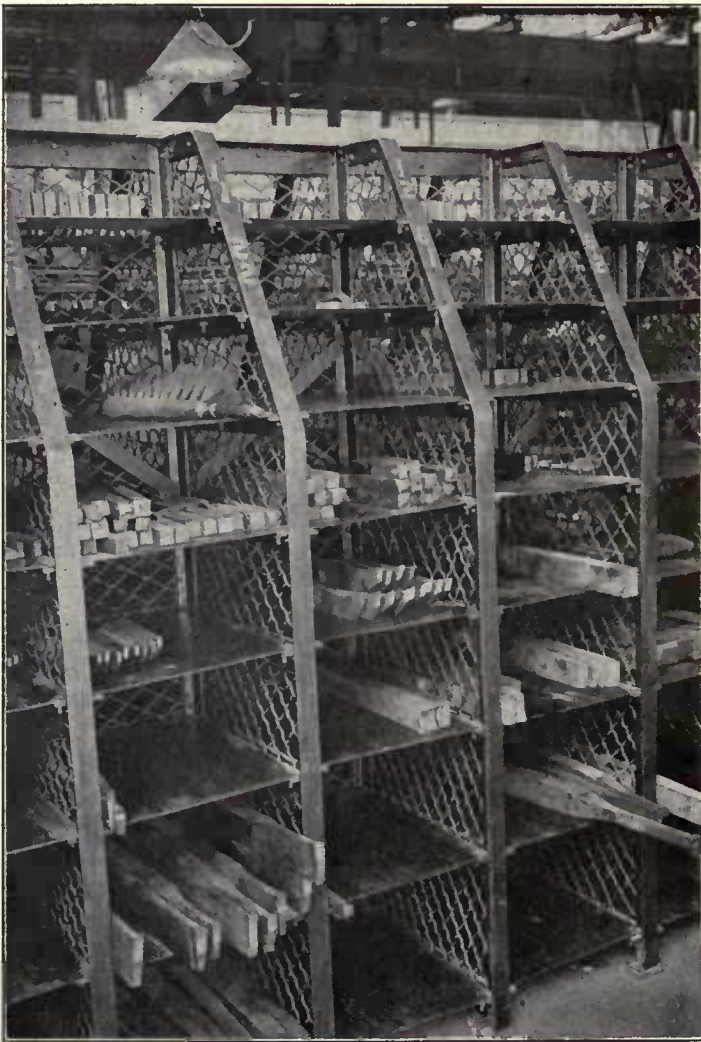
Fig. 224—Rack for Cutting Tools in Tool Room.
