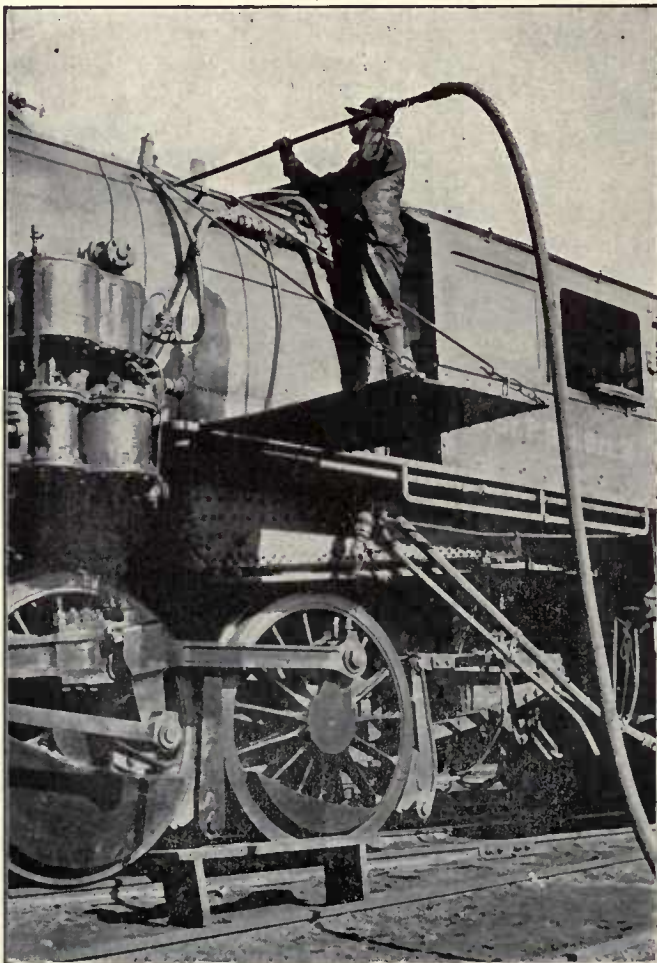
Fig. 520—Platform for Boiler Washer.
