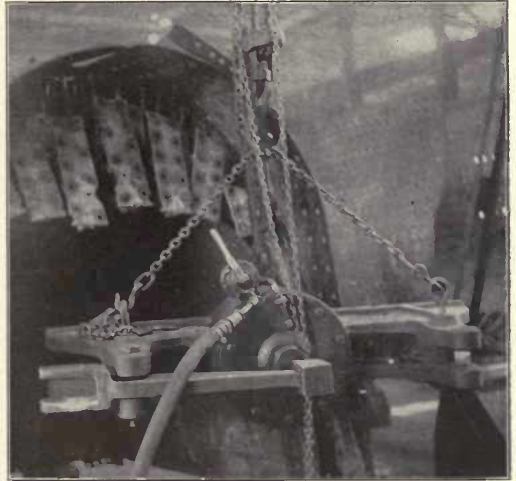
Fig. 354—Application of Staybolt Breaker.
