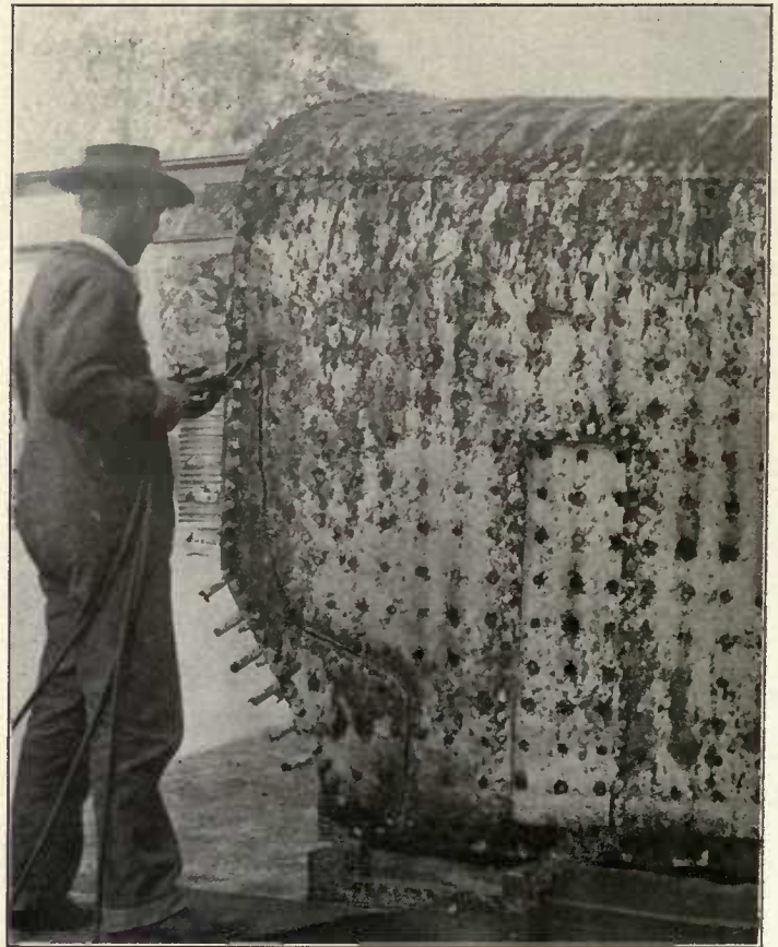
Fig. 422—Oxy-Acetylene Torch Cutting Up Scrap Firebox.
