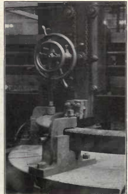
Fig. 217—Chuck Holding Tire.
