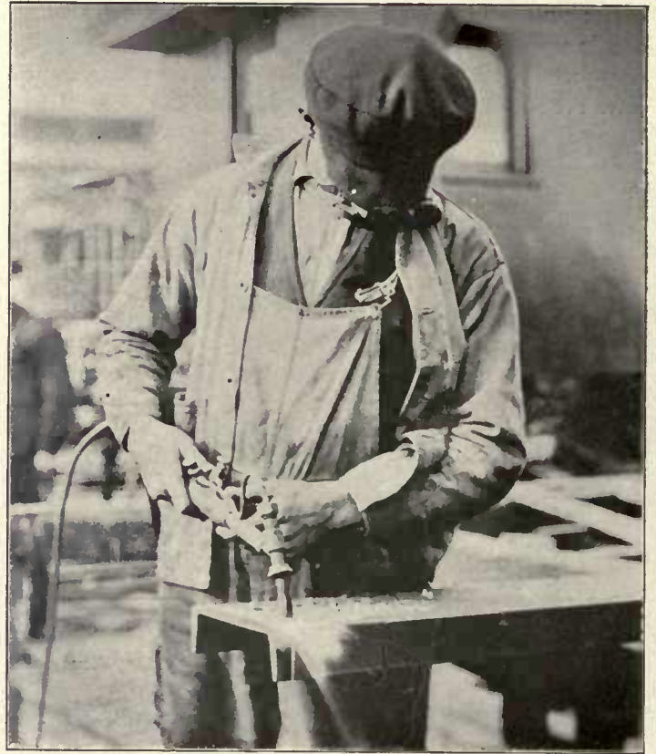
Fig. 432—Cutting a Steel Channel with an Oxy-Acetylene Torch.
