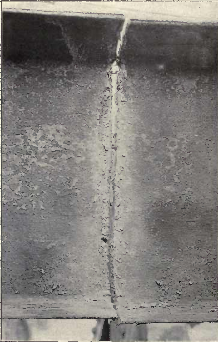
Fig. 431—Steel Center Sill Cut with Oxy-Acetylene.
