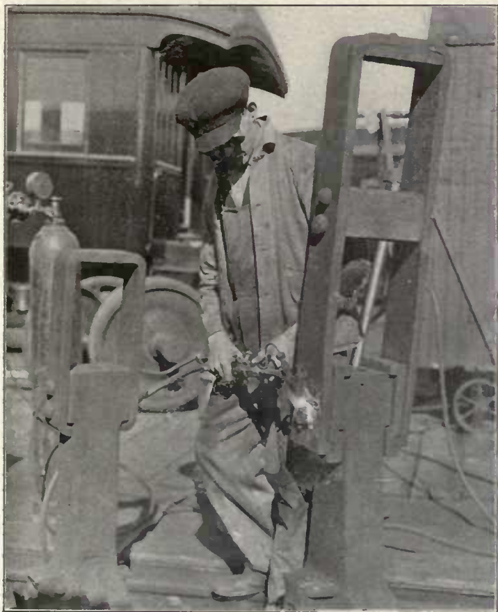
Fig. 435—Cutting off Rivet Head on Coupler Yoke with Oxy-Acetylene Torch.
