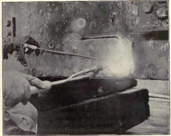
Fig. 417—Patch Welded on Outside of Firebox.
