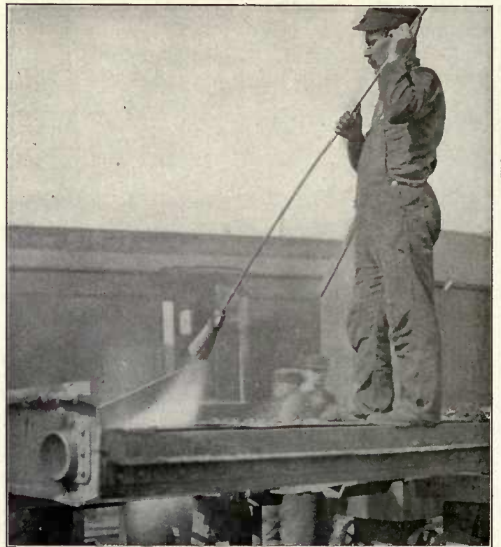
Fig. 647—Heating a Steel Center Sill with Crude Oil Burner.
