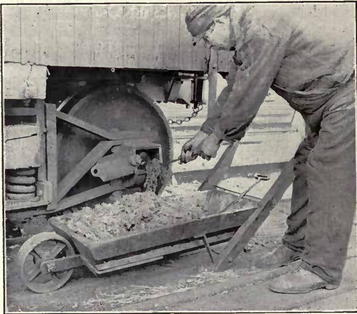
Fig. 609—Cart for Journal Box Packing.
