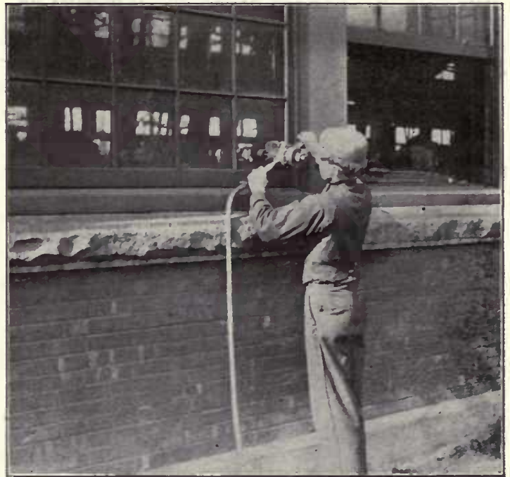
Fig. 801—Cleaning Shop Windows.
