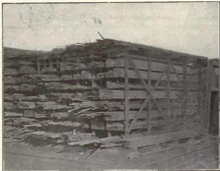
Fig. 795—Partial View of Steel Storage Rack.
