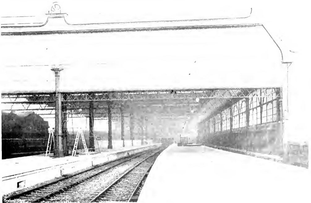
Fig. 4. Part of the New Ticket Office and Platform.
