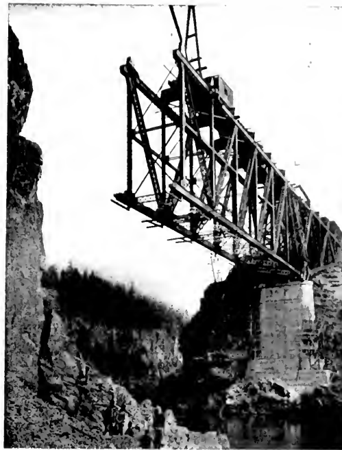
End View of Cantilever in course of Erection
