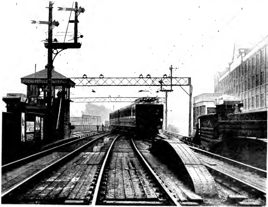
Electric Train on Cross over Road at Peckham Rye
