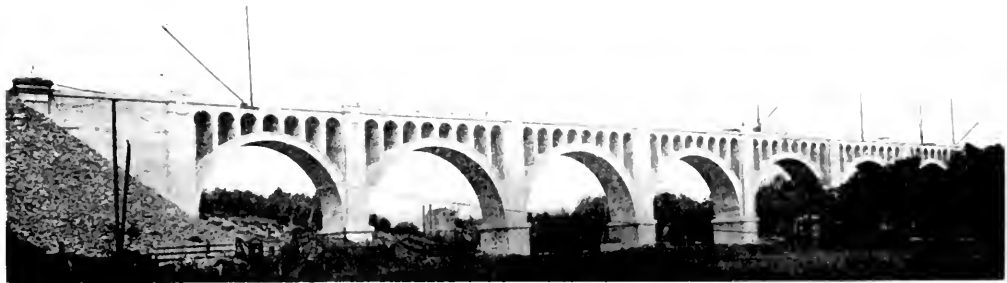
Concrete Arch Viaduct Approaching Completion
