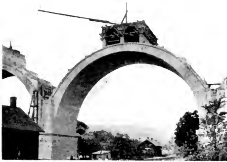
First Spandrel Arch on Main Arch Ring
