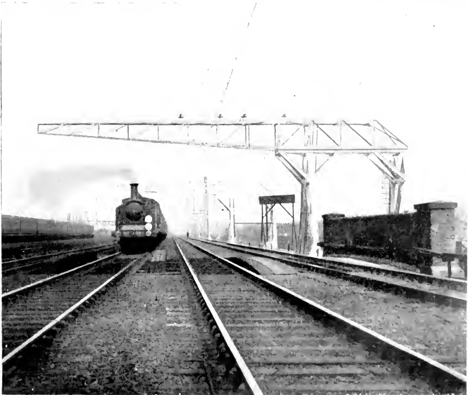
Cantilever and Overhead Wires on Crystal Palace Line
