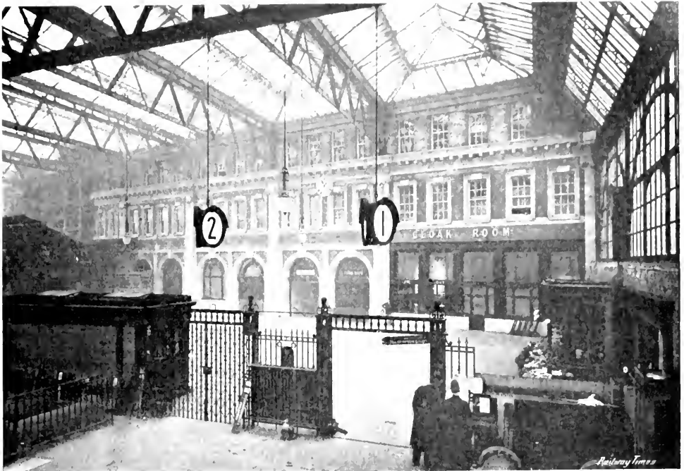
Fig. 3. New Booking Offices and Concourse Leading to Platform. (Ed. W. & A. G. & Co., Architects.)
