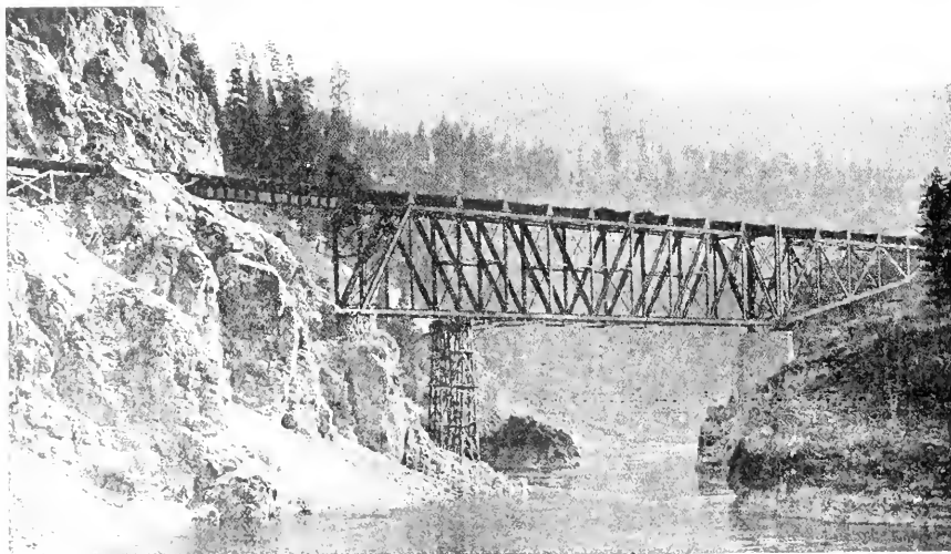
Bridge over Pend Oreille River, Washington
