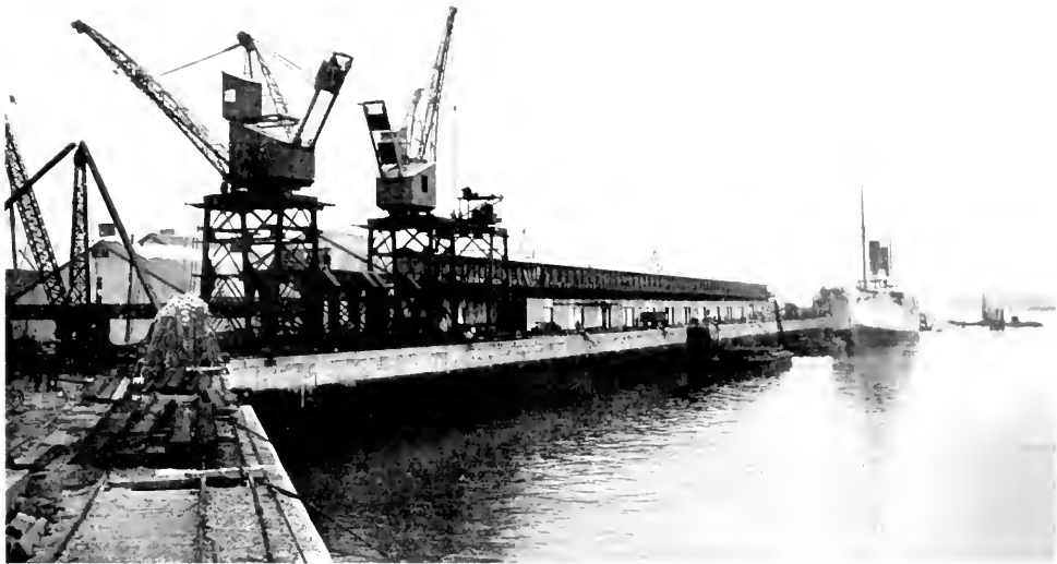
The New 16-Acre Deep Water Dock and Sheds at Southampton—admitting the Largest Vessels at all Stages of the Tide.
