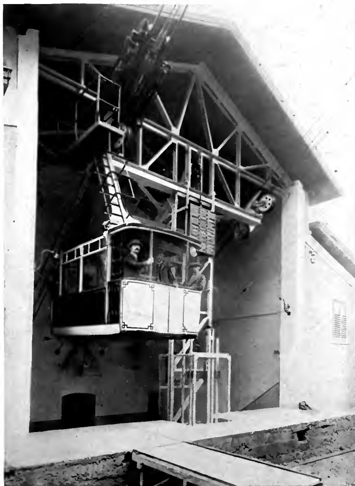
THE STARTING STATION ON THE KOHLERER AERIAL RAILWAY AT EISACK.
