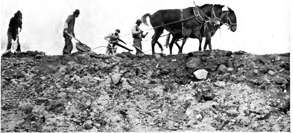
Photograph by permission of the Canadian Northern Railway. PLOUGHING OFF THE TOP OF A HILL TO LEVEL THE GRADE ON THE CANADIAN NORTHERN TRANSCONTINENTAL.
