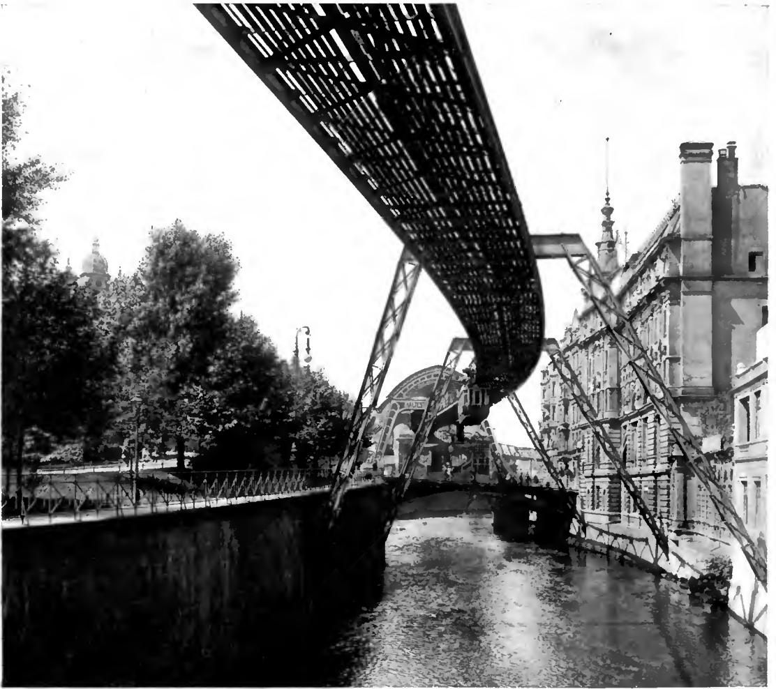
THE RAILWAY ABOVE THE WUPPER RIVER IN ELBERFELD. Showing the A-shaped supports.
