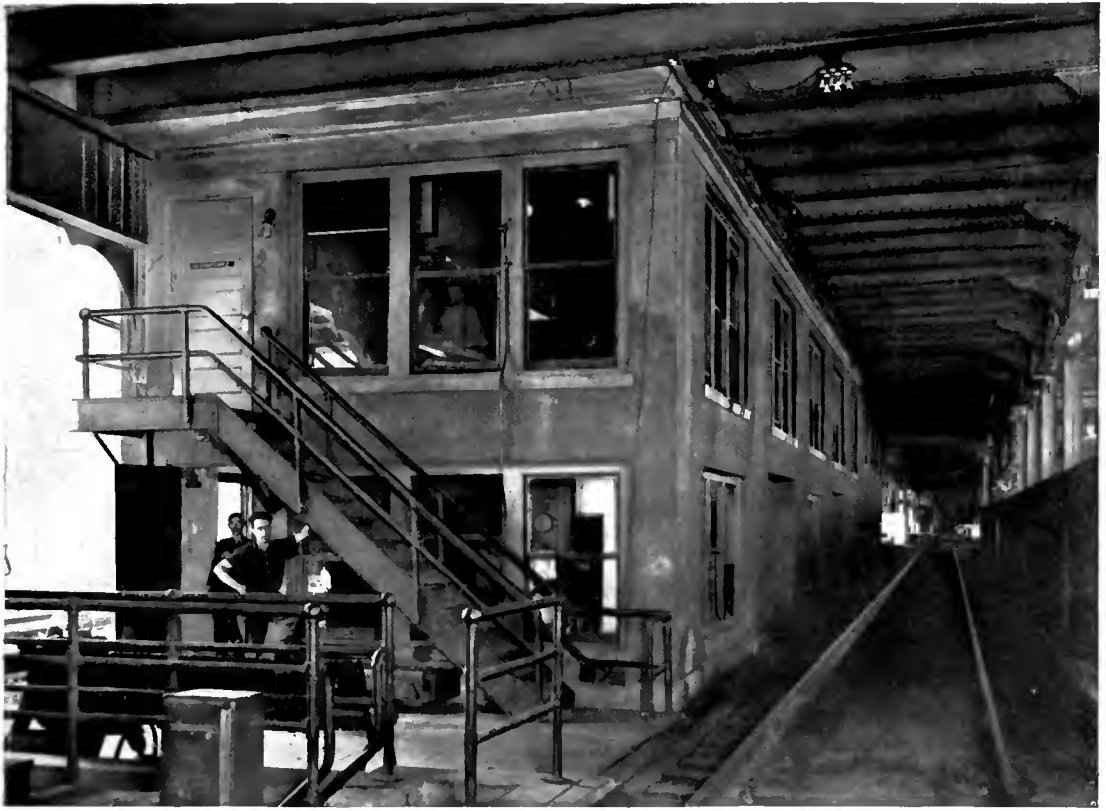
EXTERIOR OF THE CABIN CONTAINING THE 360-LEVER MACHINE CONTROLLING ALL TRAIN MOVEMENTS TO AND FROM THE UPPER LEVEL.
