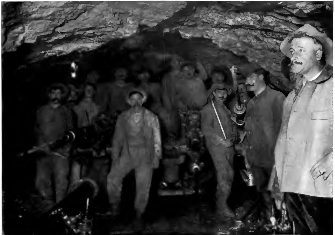
A BORING GANG WITH A MEYER DRILL IN THE HEADING.
