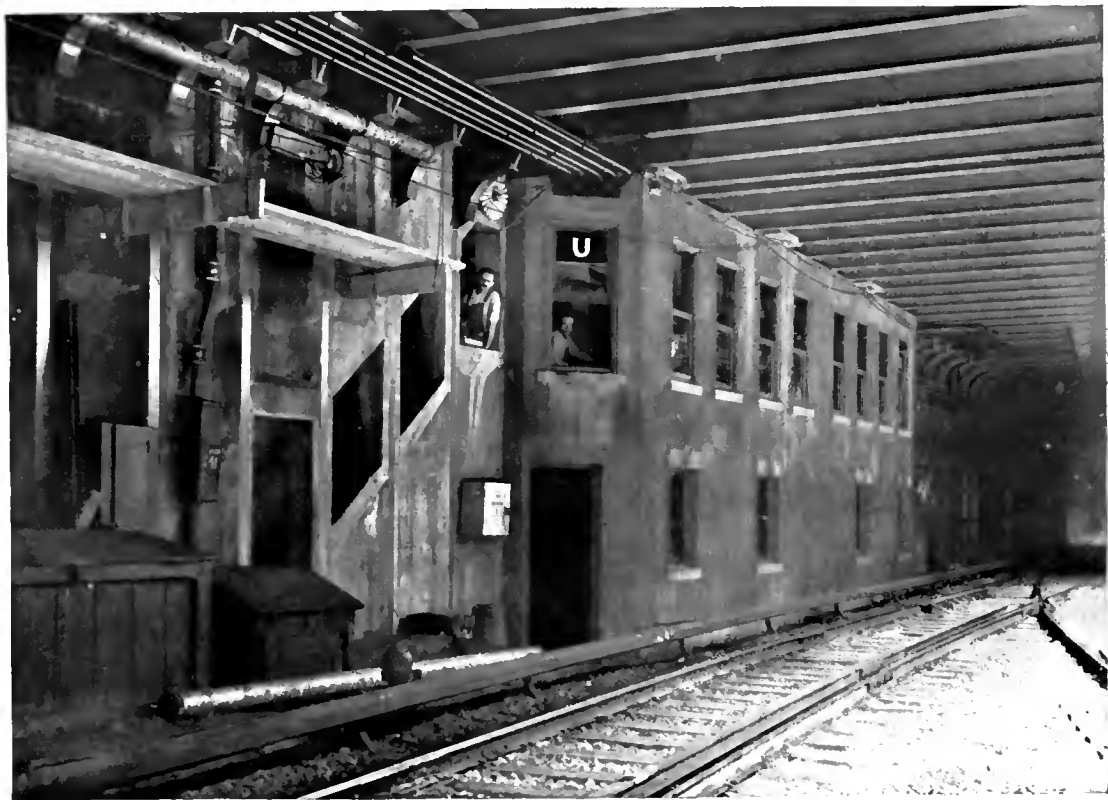
EXTERIOR OF ONE OF THE UNDERGROUND INTERLOCKING STATIONS.
