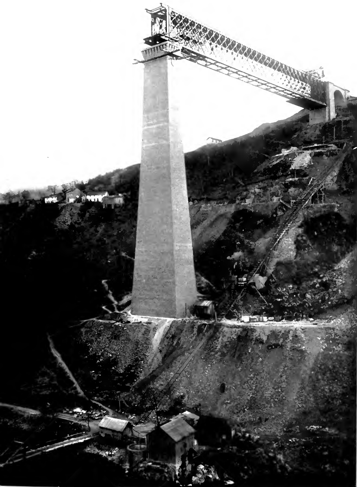
THE FIRST COMPLETED SPAN OF THE FADES VIADUCT. The view shows the engineers' inclined railway down the valley side.
