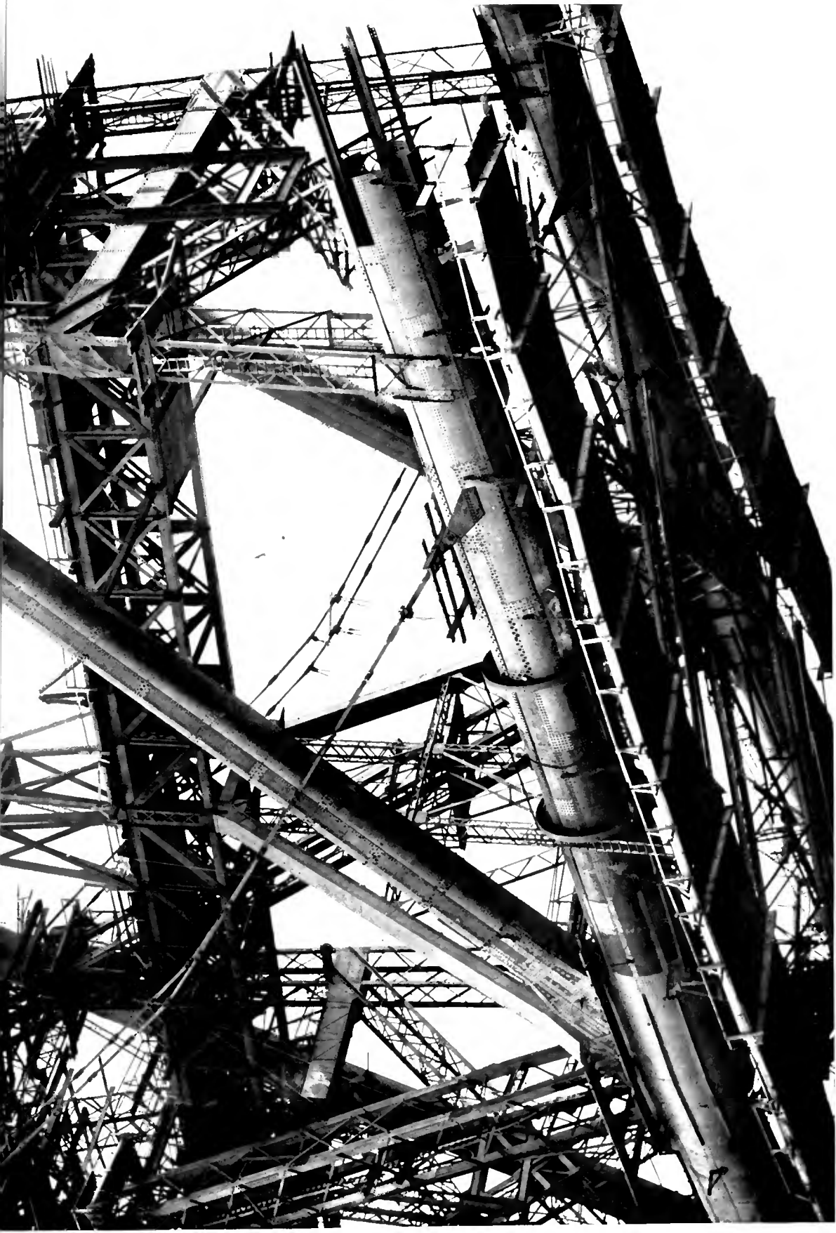
BUILDING THE MIGHTY FABRIC OF STEEL: THE FIVE NORTH CANTILEVER, JULY 6, 1888. This photograph conveys a vivid idea of the gigantic character of the work and the ingenious methods adopted in erection. At the bottom are the huge steel tubes which spring from the base of each cantilever pier.
