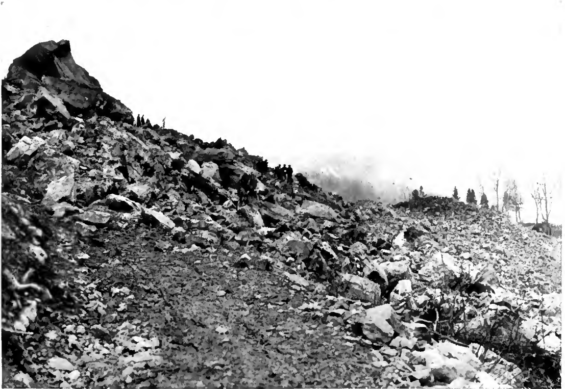
After the blast: 20,000 tons of disintegrated granite.
