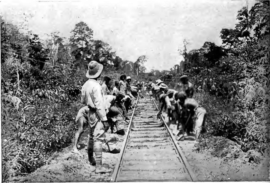
LEVELLING AND BALLASTING THE LINE. The work was done entirely by negro labour
