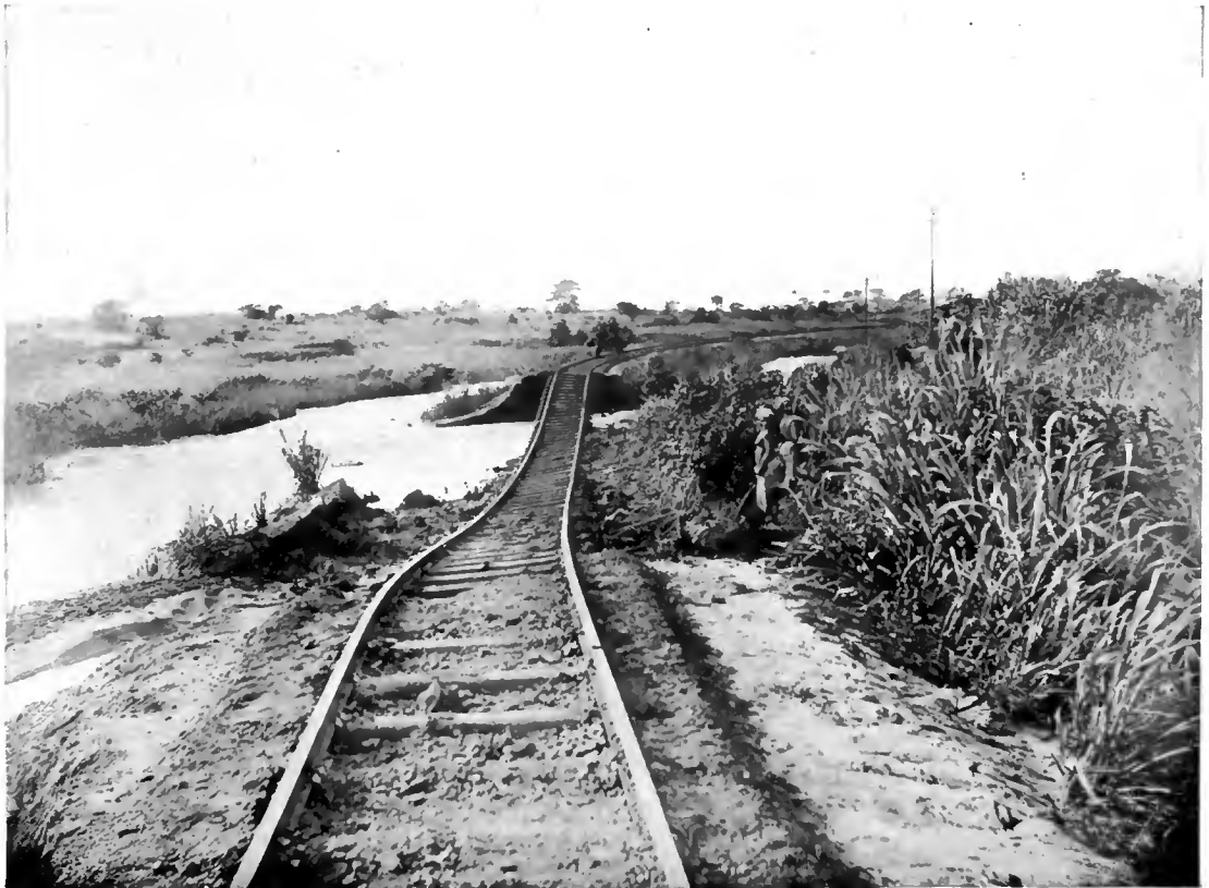
A CONSTANT MENACE TO SECTIONS OF THE GOLD COAST RAILWAY. A wash-out in the Achemotah Valley.
