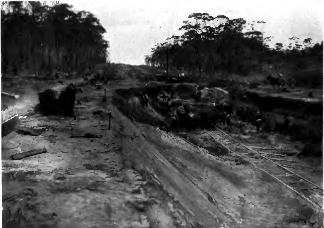
CUTTING OUT THE ZIGZAG. NEW SOUTH WALES.
