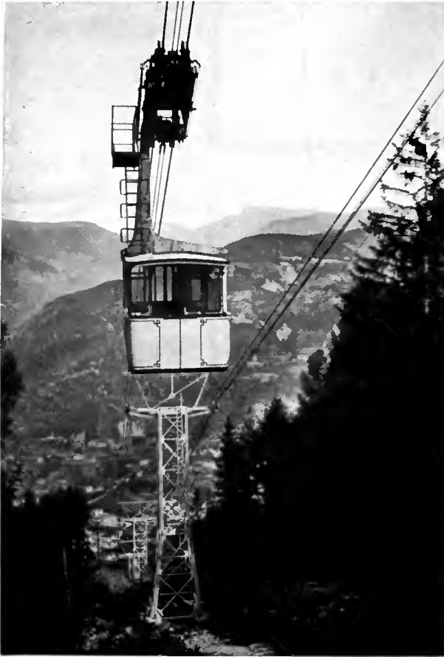
VIEW OF THE TRACK OF THE KOHLERER AERIAL RAILWAY. Showing the method of suspending the car from the track carriage, and the two cables.
