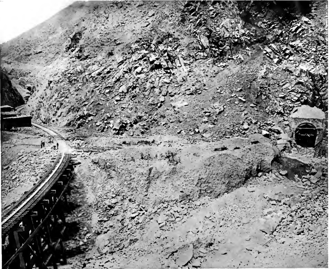
BUILDING THE ESPERANZA TUNNEL ON THE OROYA RAILWAY.
