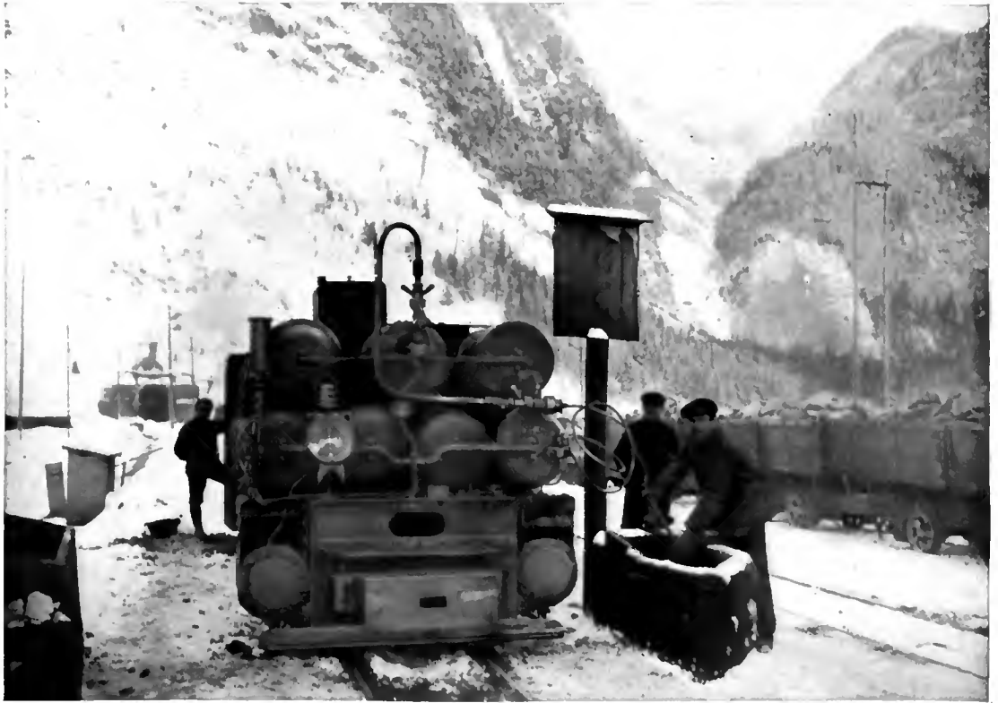
CHARGING A COMPRESSED-AIR ENGINE AT KANDERSTEG.
