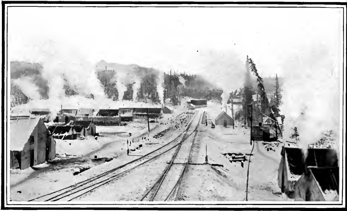
A RAILWAY CONSTRUCTION CAMP ON THE BORDERS OF THE ARCTIC CIRCLE.
