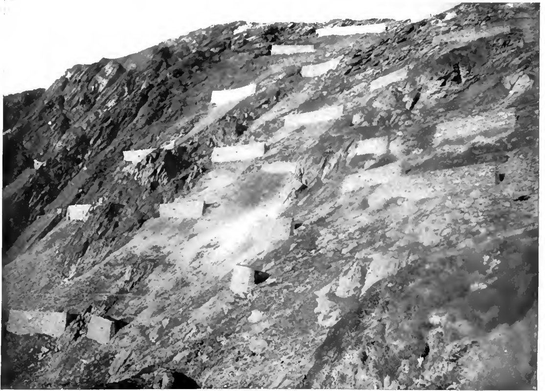
WALLS BUILT ON THE MOUNTAIN SLOPES TO PROTECT THE TUNNEL-ENTRANCES FROM AVALANCHES.
