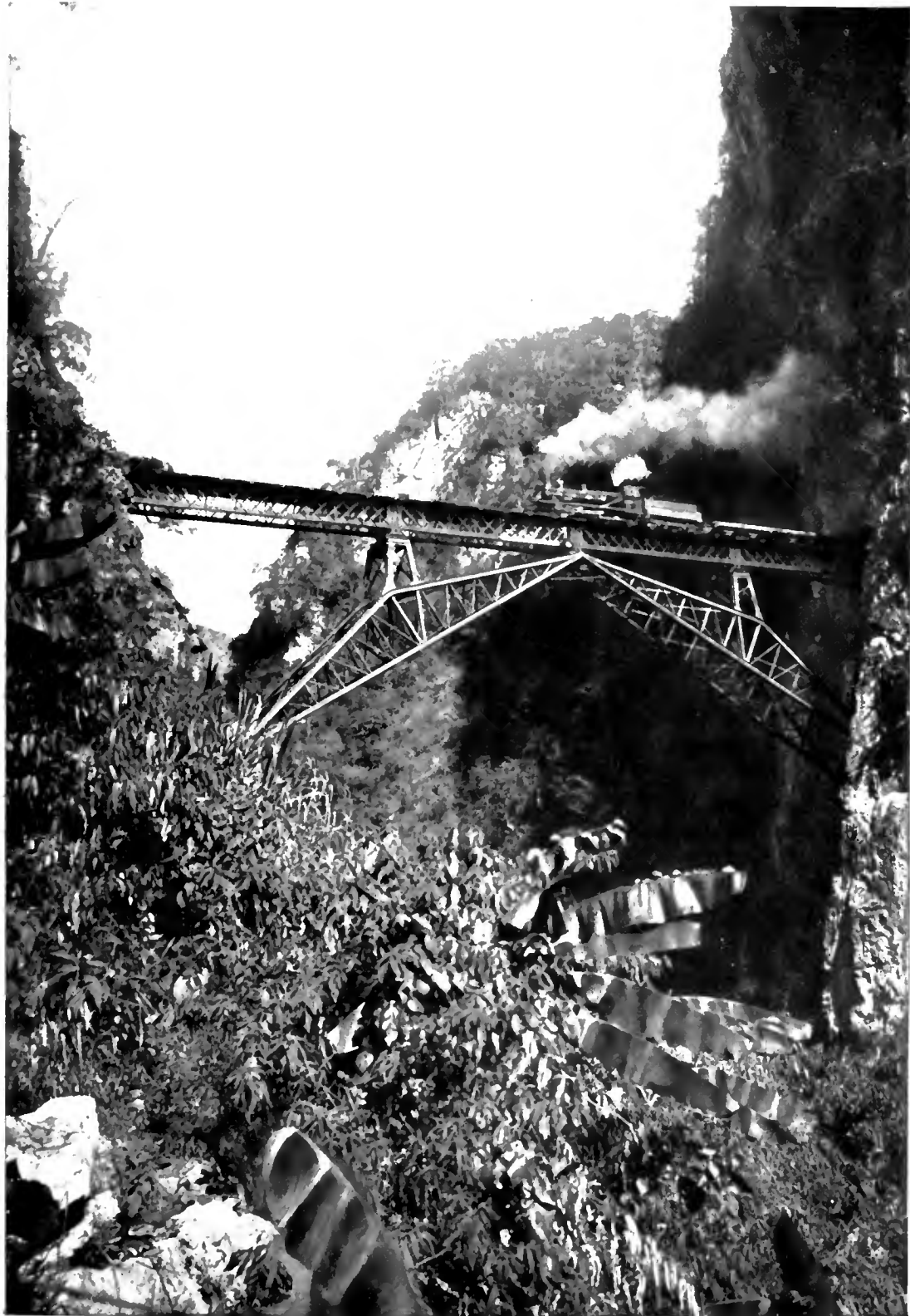
THE FAUX NAM-TI BRIDGE COMPLETE.
