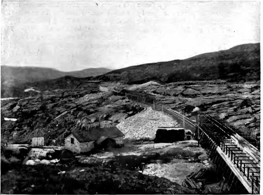
BUILDING A SNOW-SHED ON THE LOFOTEN RAILWAY, SCANDINAVIA.
