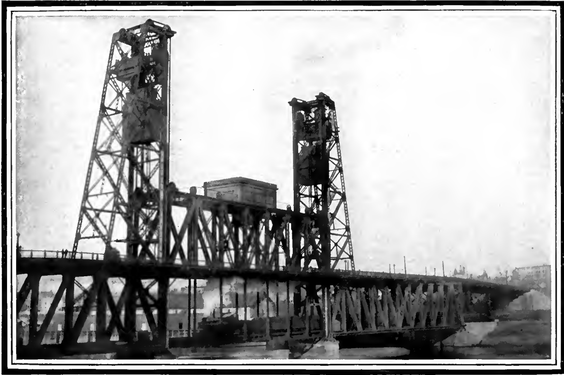
THE BRIDGE OPEN FOR VEHICULAR, PEDESTRIAN, AND TRAIN SERVICE.
