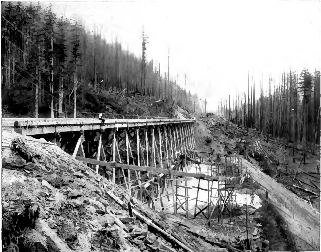
SLUICING A TRESTLE: THE LATEST METHOD OF BUILDING AN EMBANKMENT.
