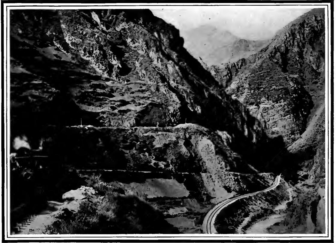
THREE DIFFERENT LEVELS ON THE OROYA RAILWAY.
