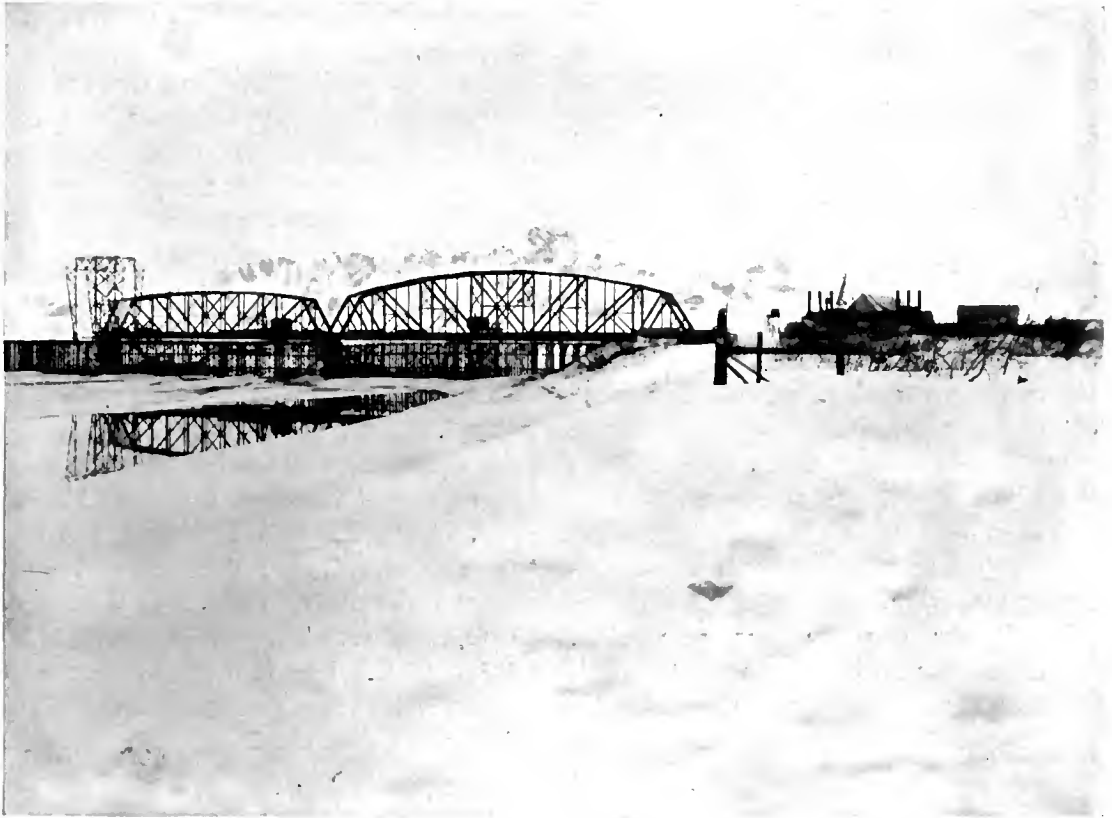
BUILDING THE GREAT STEEL BRIDGE ACROSS THE COPPER RIVER.
