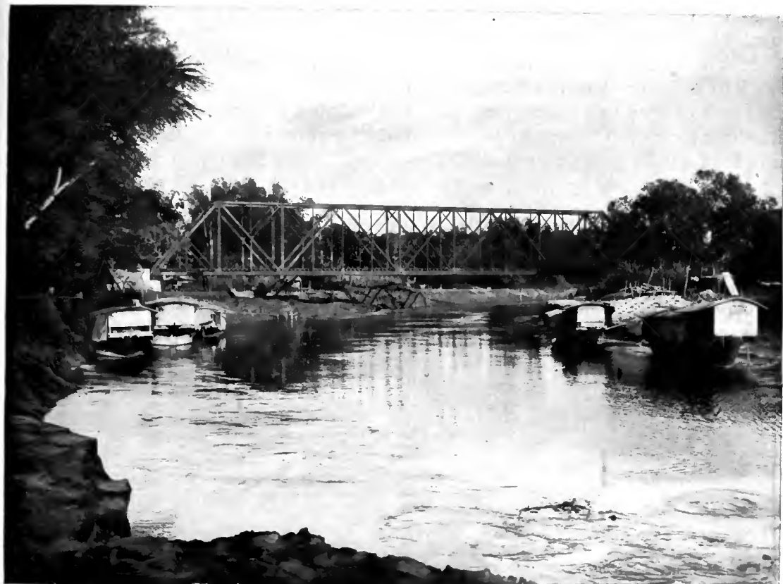
A SINGLE SPAN BRIDGE OVER THE KLONG THA LAW, ON THE NORTHERN RAILWAY, SIAM The span is 263 feet. On the river are some of the quaint craft by which transportation was effected before the railway was built.
