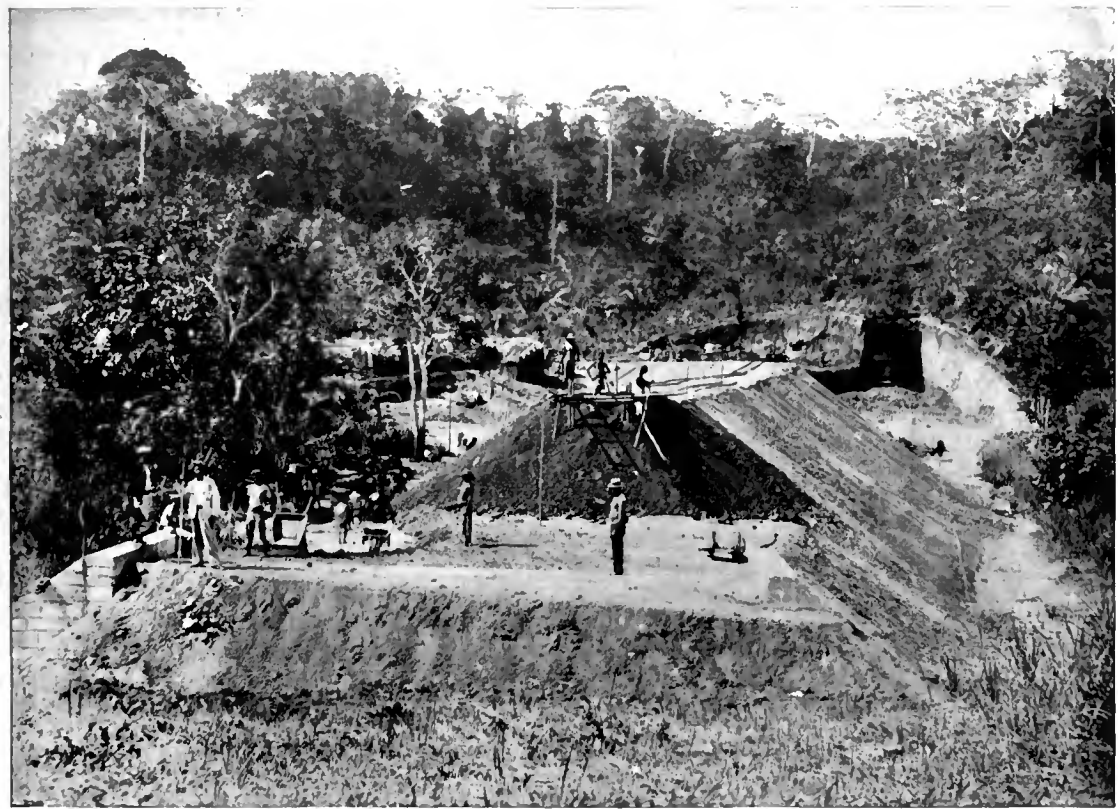
BUILDING UP THE GRADE TO TRACK LEVEL.
