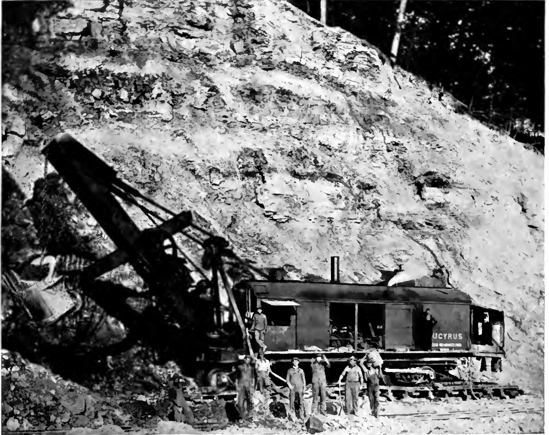
THE STEAM SHOVEL PLOUGHING ITS WAY THROUGH A DEEP CUT.
