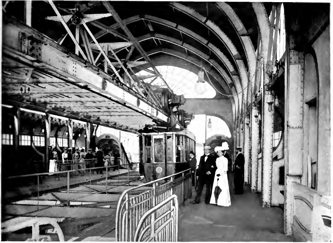
THE INTERIOR OF DOEPPERSBERG STATION AT ELBERFELD. Showing method of suspending the car and the wire netting protection between platforms.
