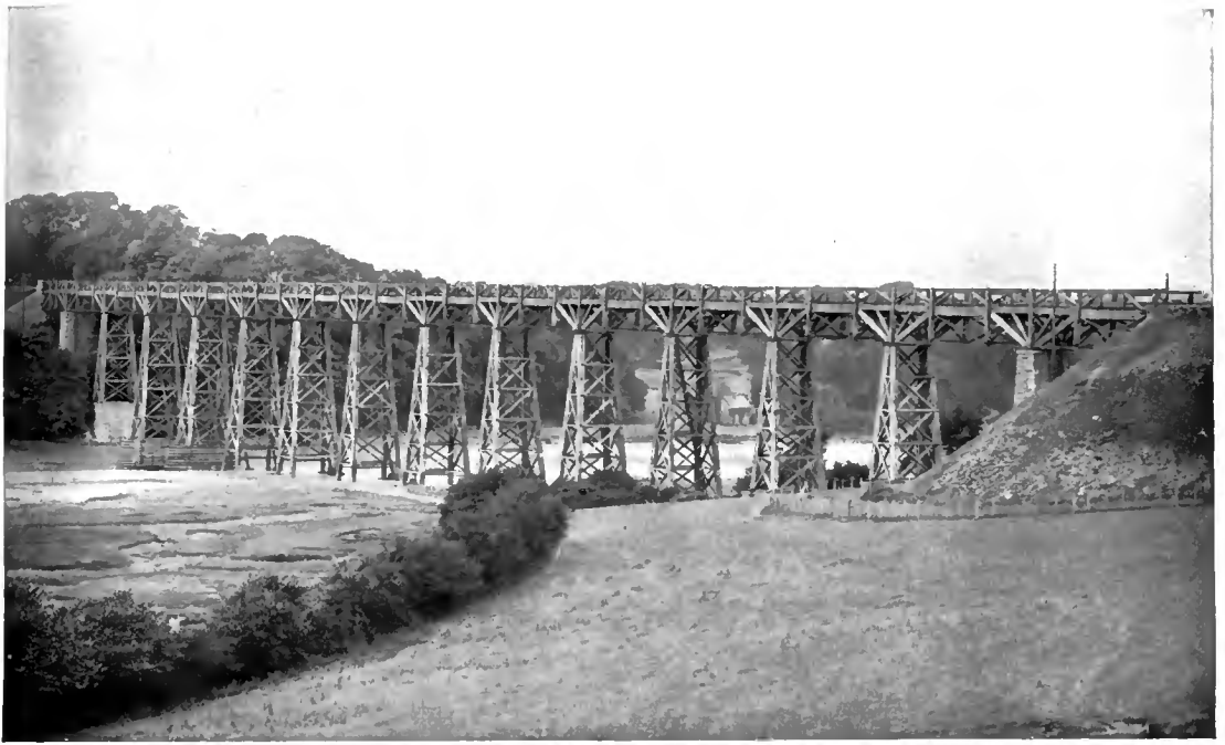
Photograph supplied by the Great Western Railway Co.
