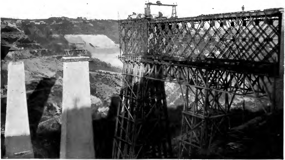
THE TIMBER FALSEWORK FOR ERECTING ONE-HALF OF A SHORE SPAN.
