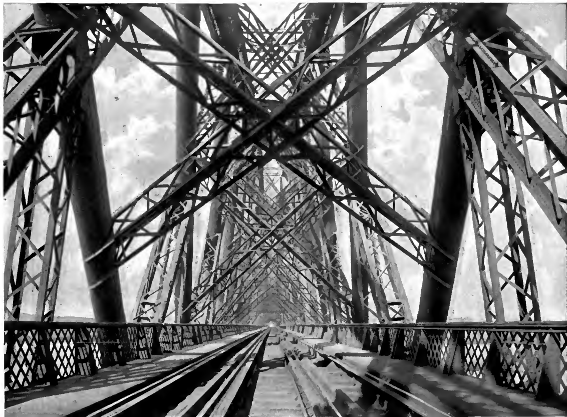
LOOKING THROUGH THE FORTH BRIDGE.
