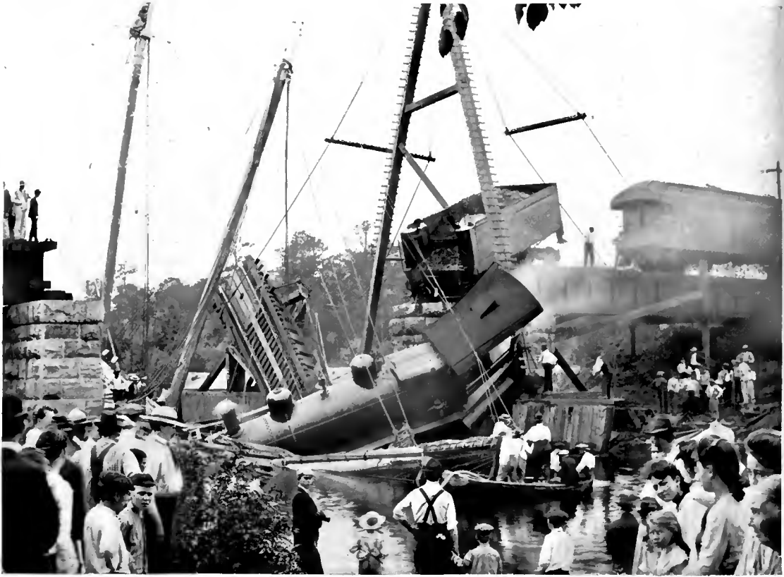
A NASTY SMASH: THE LOCOMOTIVE FELL THROUGH AN OPEN DRAWBRIDGE ON TO THE DECK OF A VESSEL WHICH HAPPENED TO BE PASSING AT THE MOMENT: THE LATTER WAS SUNK BY THE IMPACT.
