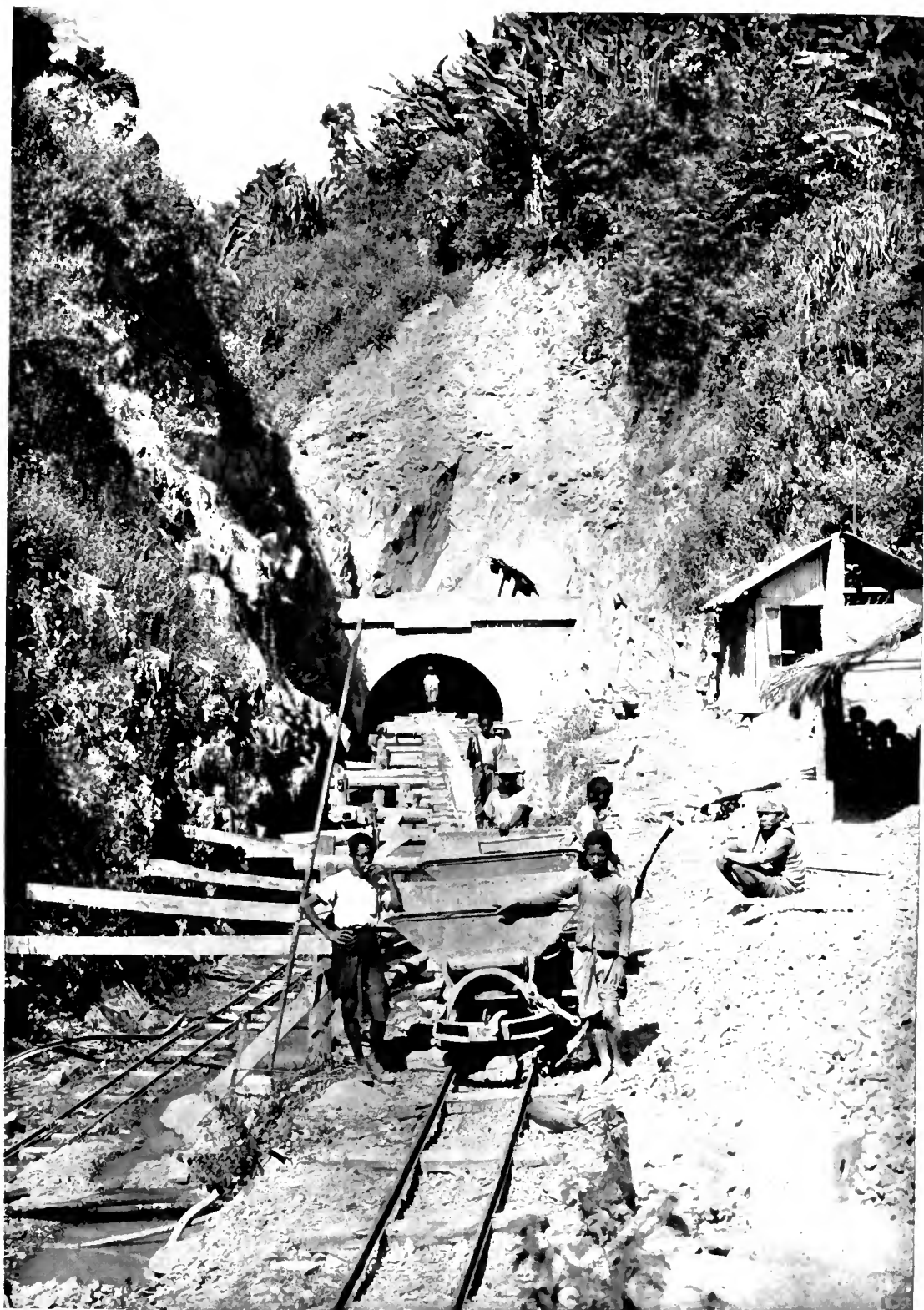
BUILDING A TUNNEL ON THE MOUNTAIN SECTION OF THE NORTHERN RAILWAY OF SIAM.
