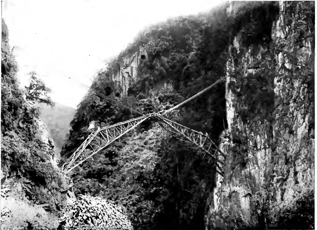
THE BASCULES OF THE FAUX NAM-TI BRIDGE SET AND CONNECTED. Showing the ropes whereby each section was lowered.
