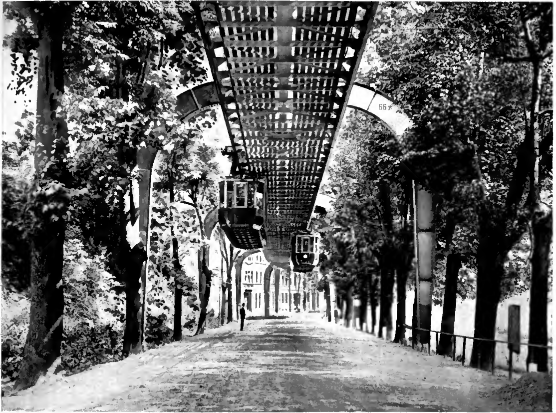
THE SUSPENDED RAILWAY OVER A PUBLIC HIGHWAY. Showing the inverted U-shaped supports for the two tracks.
