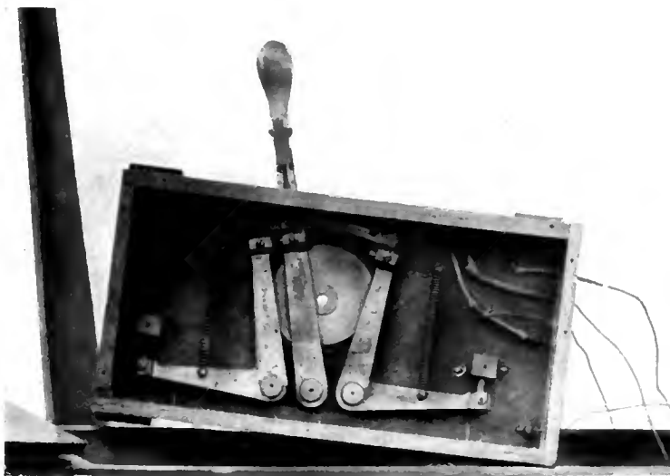
THE CONTROLLER OF EDISON'S FIRST ELECTRIC LOCOMOTIVE.
