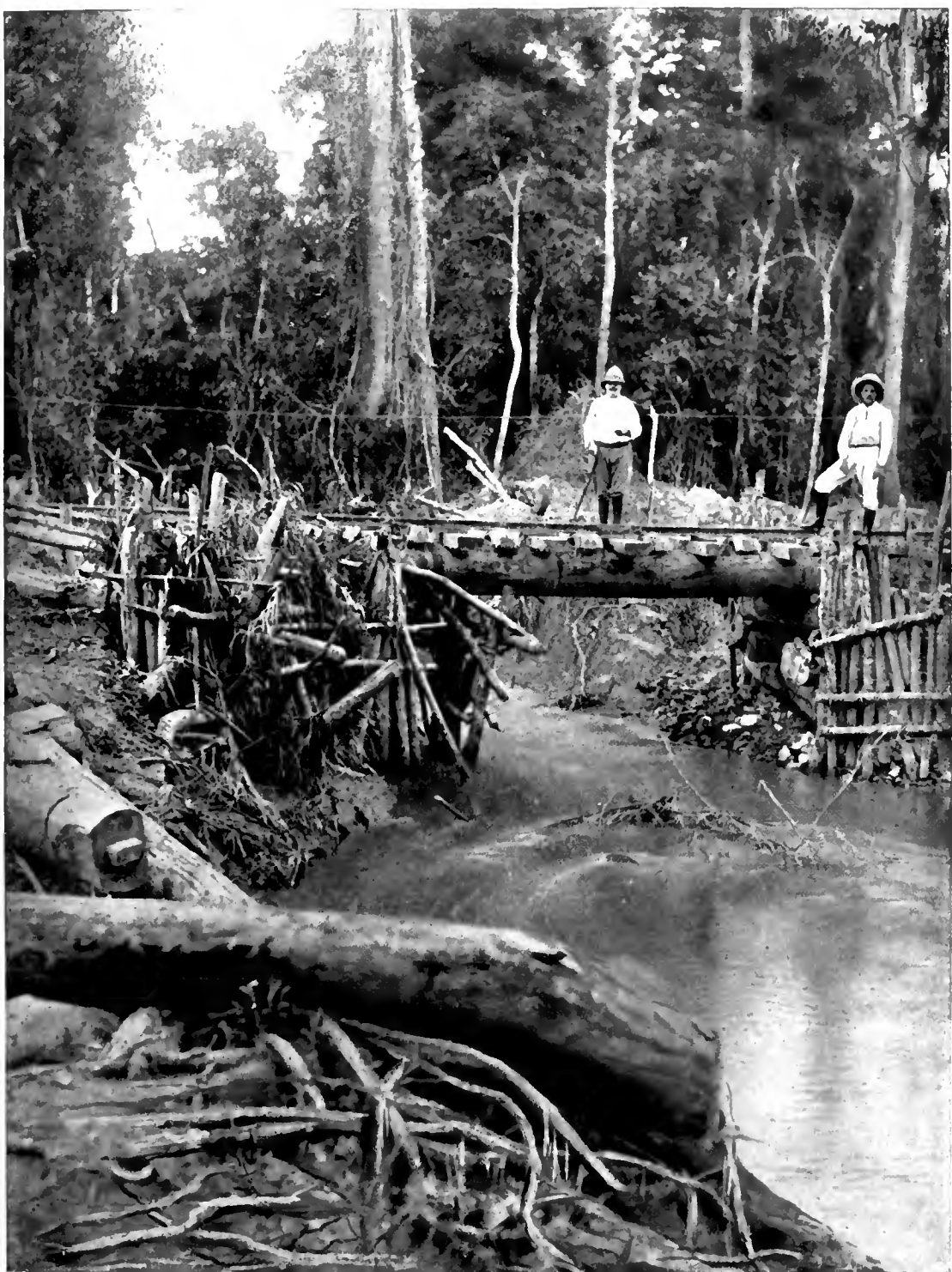
A TEMPORARY BRIDGE OVER THE SUYAM RIVER.
