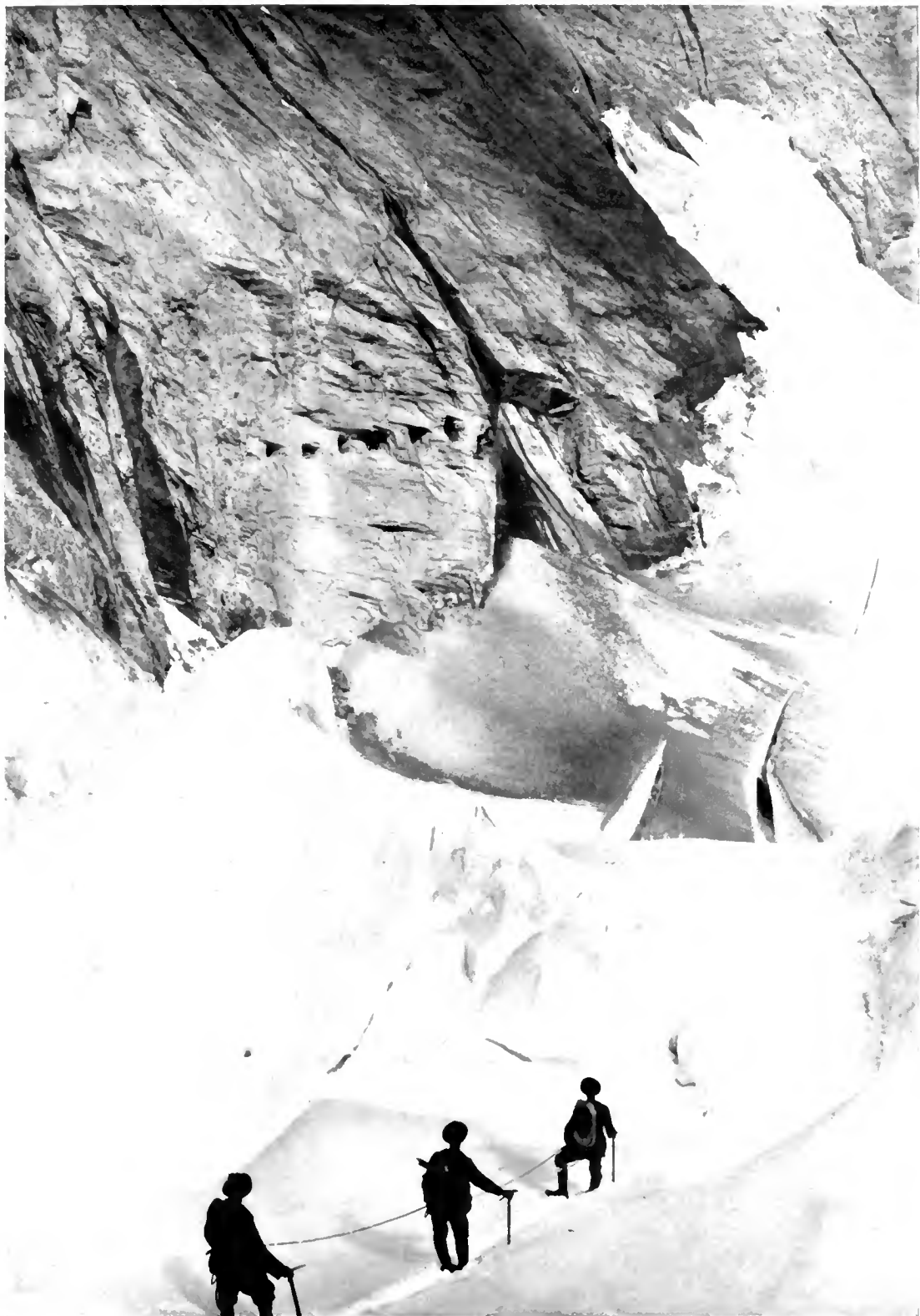
EISMEER STATION FROM THE OUTSIDE, SHOWING WINDOWS TWENTY FEET WIDE CUT IN THE ROCK.
