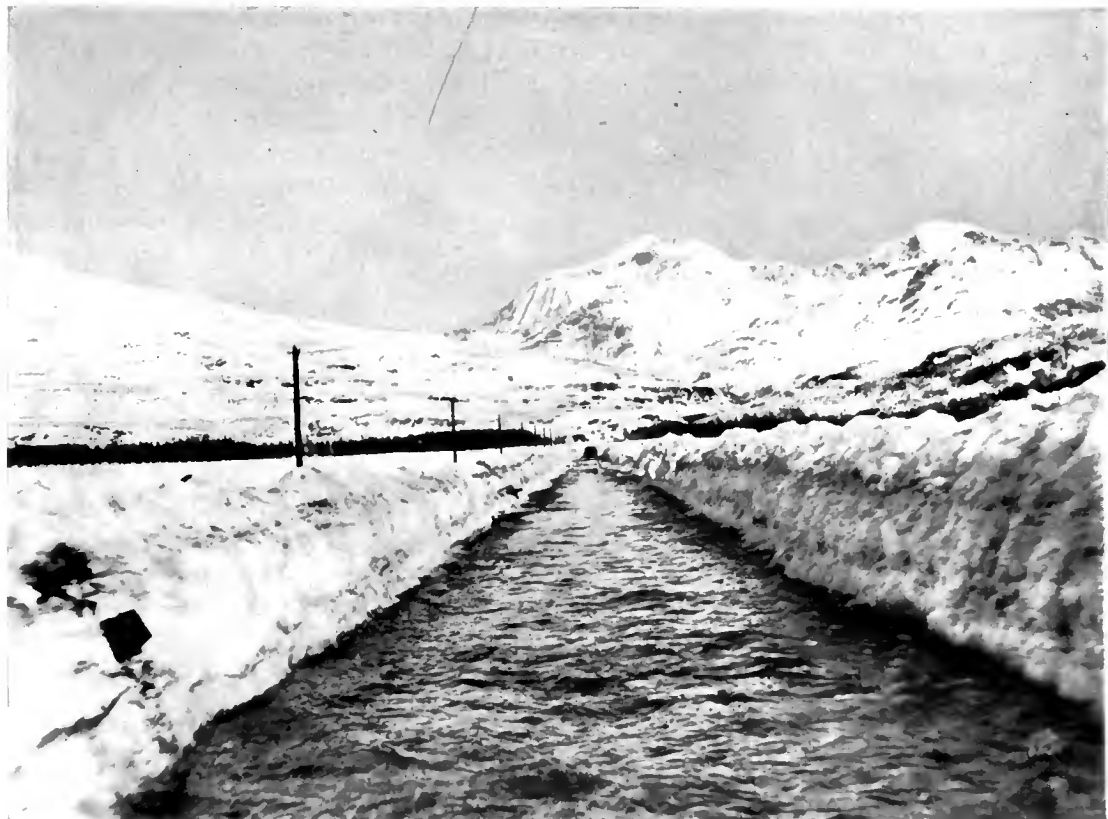
NOT A CANAL, BUT THE RAILWAY FLOODED.
