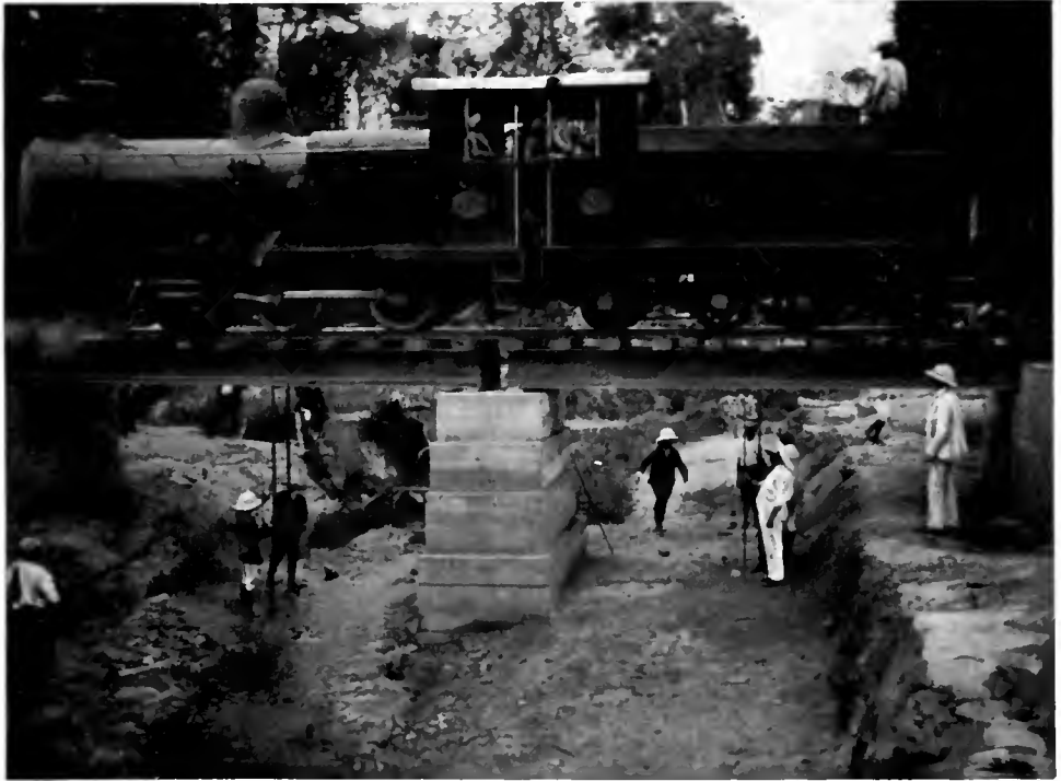
TESTING A BRIDGE ON THE GOLD COAST RAILWAY.
