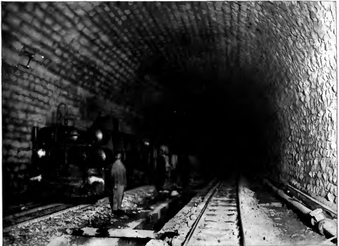
A SECTION OF THE COMPLETED TUNNEL SHOWING LINING.
