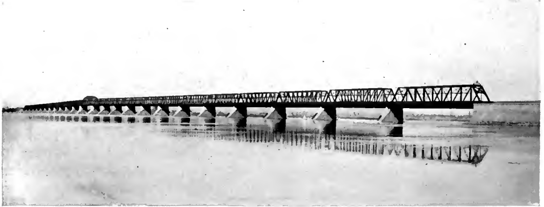
THE VICTORIA JUBILEE BRIDGE, MONTREAL, SHOWING THE NEW SUPERSTRUCTURE.
