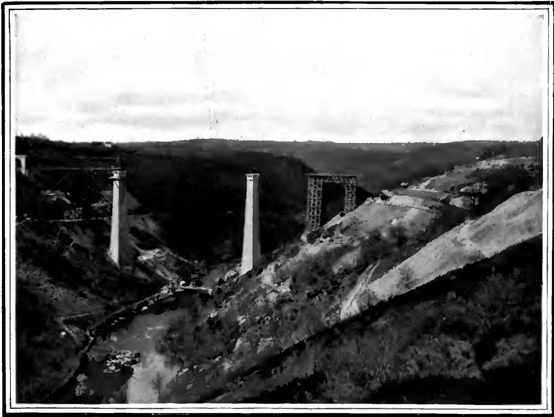
GENERAL VIEW OF THE SIOULE RIVER VALLEY AND THE VIADUCT WORKS SHOWING THE TWO CHIMNEY-LIKE PIERS.
