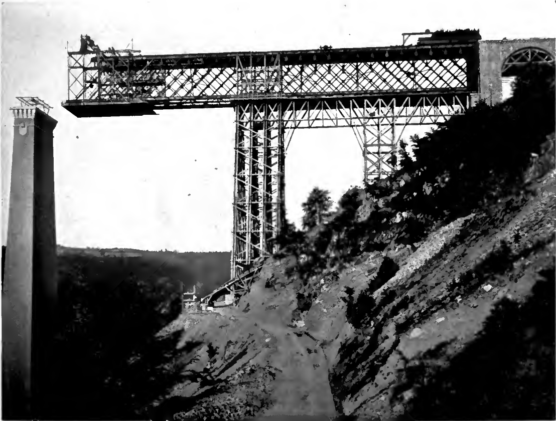
CRAWLING FOOT BY FOOT TOWARDS THE FIRST PIER.
