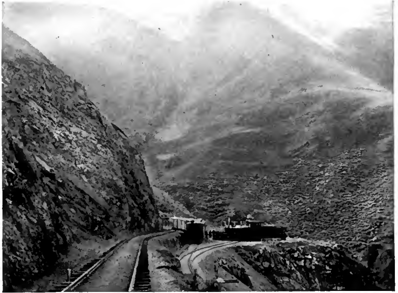
THE MEIGGS V-SWITCH ON THE OROYA RAILWAY.
