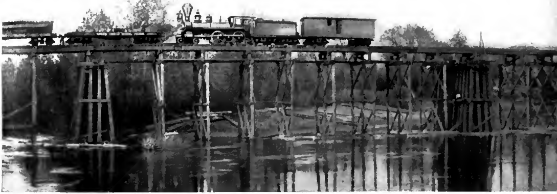
AN EARLY LOCOMOTIVE AND ROLLING STOCK, SHOWING CHEAP TIMBER TRESTLE CONSTRUCTION.
