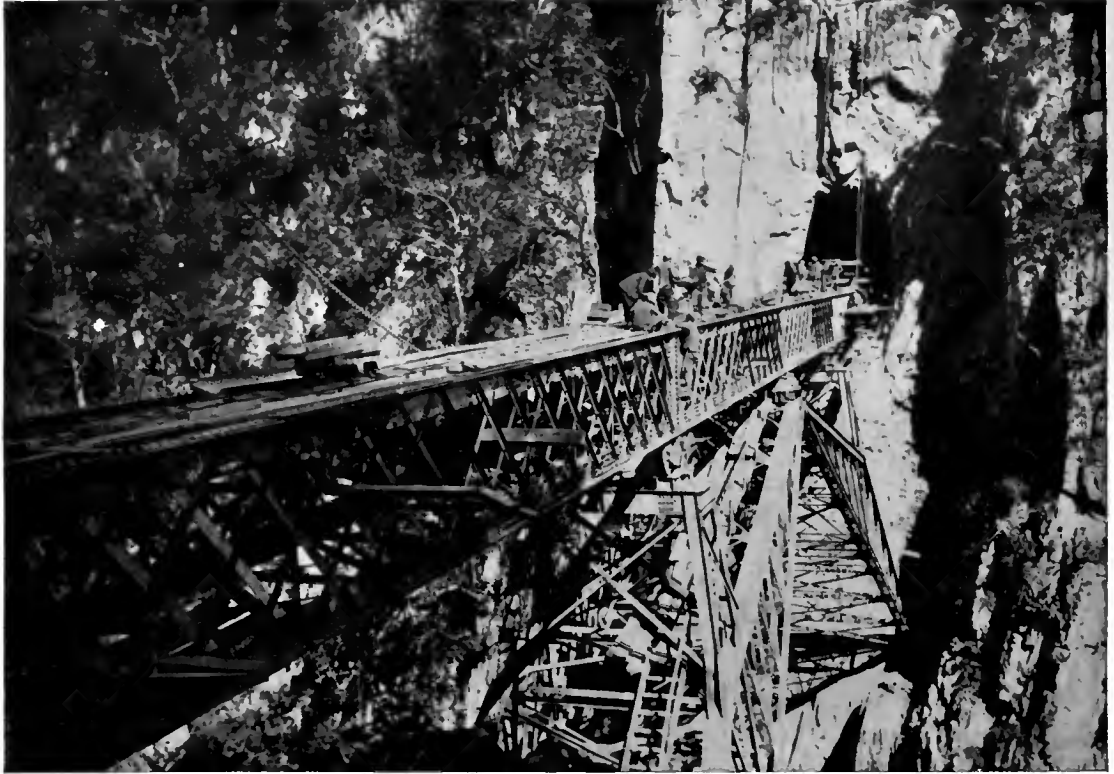
RIVETING UP THE TRACK DECK OF THE FAUX NAM-TI BRIDGE.
