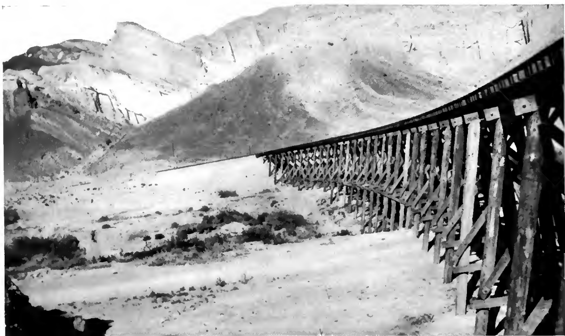
A HEAVY STRETCH OF TRESTLING.
