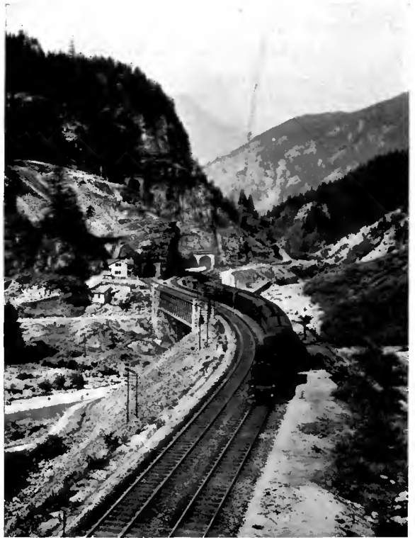
ONE OF THE SPIRAL TUNNELS ON THE ST. GOTTHARD RAILWAY.
