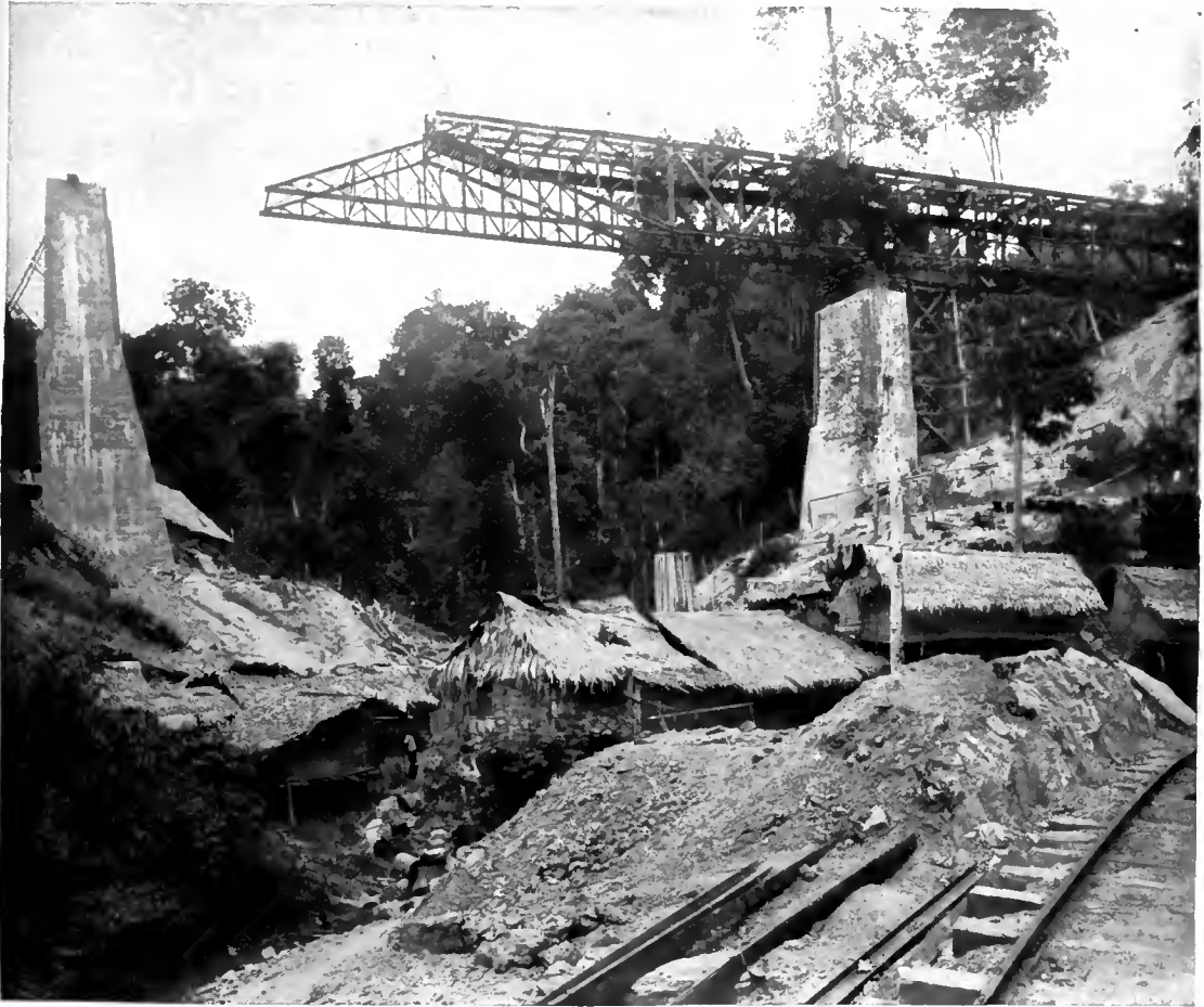
BRIDGE-BUILDING IN THE SIAMESE JUNGLE.
