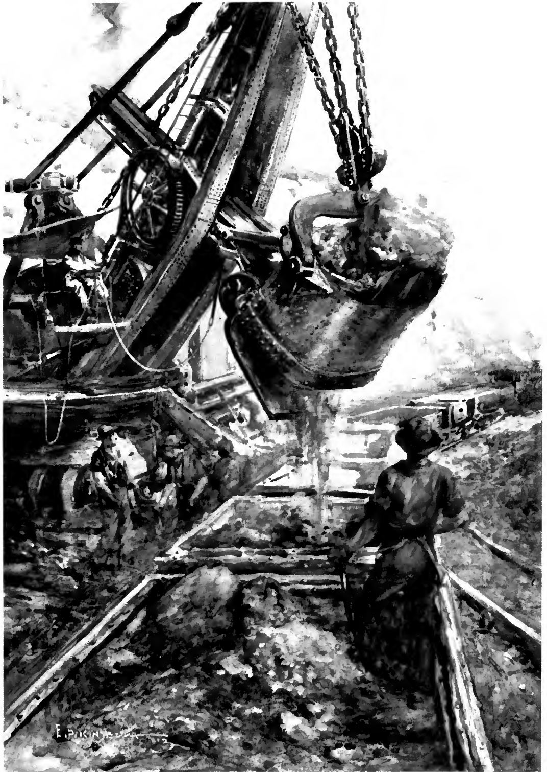
THE STEAM SHOVEL, THE RAILWAY BUILDERS' MOST SERVICEABLE TOOL. Few devices have facilitated and expedited railway construction so much as the steam shovel, which is capable of removing three or more tons of spoil at a time
