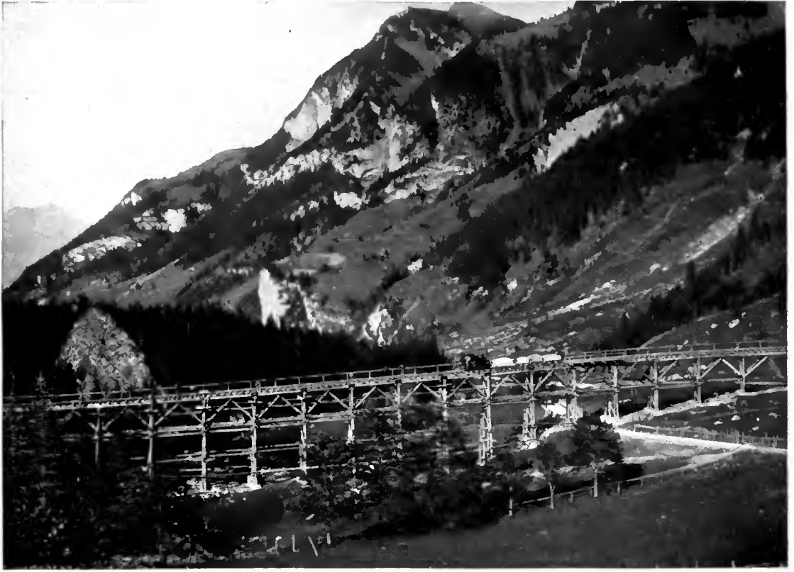
THE TEMPORARY TIMBER VIADUCT AND CONSTRUCTION TRAIN.
