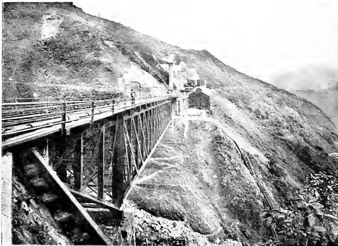
BANKHEAD SHOWING POWER HOUSE FOR DRIVING THE CABLES.
