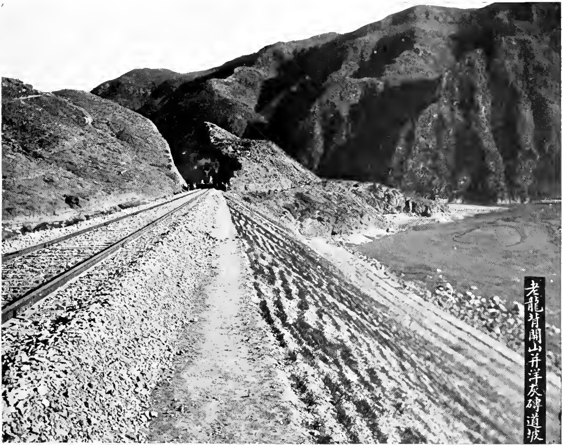
A TYPICAL STRETCH OF TRACK AMONG THE MOUNTAINS ON THE PEKING-KALGAN RAILWAY, SHOWING SOLID CHARACTER OF THE GRADE.
