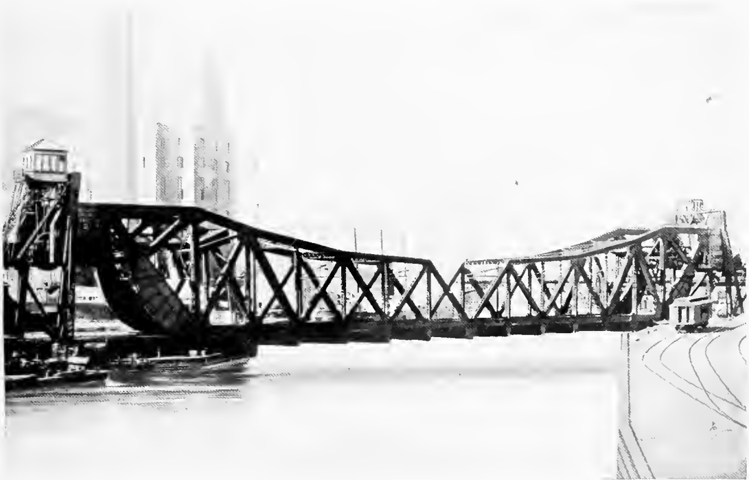
275-FOOT DOUBLE-LEAF DOUBLE-TRACK SCHERZER ROLLING LIFT BRIDGE ACROSS THE CHICAGO RIVER AT THE ENTRANCE TO THE GRAND CENTRAL STATION, CHICAGO.
