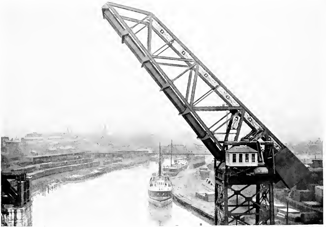
160-FOOT SINGLE-LEAF DOUBLE-TRACK SCHERZER ROLLING LIFT BRIDGE ACROSS THE CUYAHOGA RIVER AT CLEVELAND, OHIO, U.S.A.
