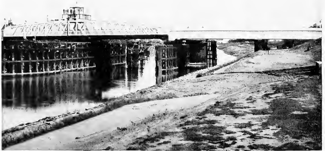
THE SUTTON SWING BRIDGE.
