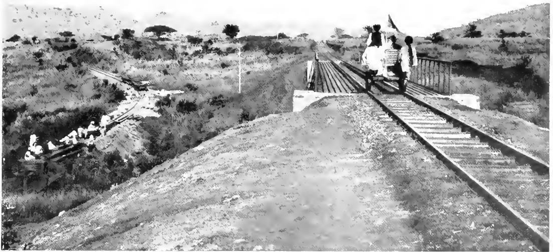
A BIG LOOP ON THE UGANDA RAILWAY TO OVERCOME A SUDDEN STEEP ASCENT.
