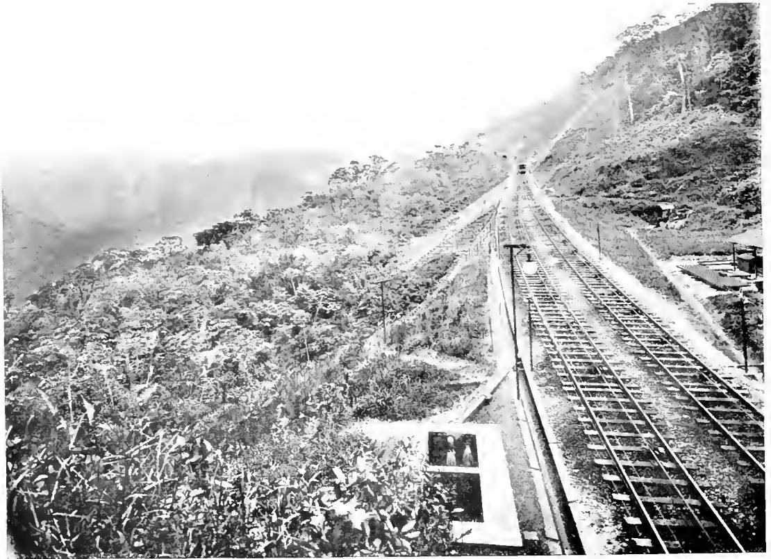
PASSING PLACE ON THE INCLINE. SHOWING UP AND DOWN TRACKS AND CABLES.
