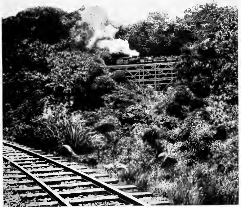
SHAY GEARED LOCOMOTIVE ROUNDING HORSE-SHOE CURVE OF 164 FEET RADIUS AND RISING 1 IN 20 UPON THE MOUNT ARISAN RAILWAY, FORMOSA.
