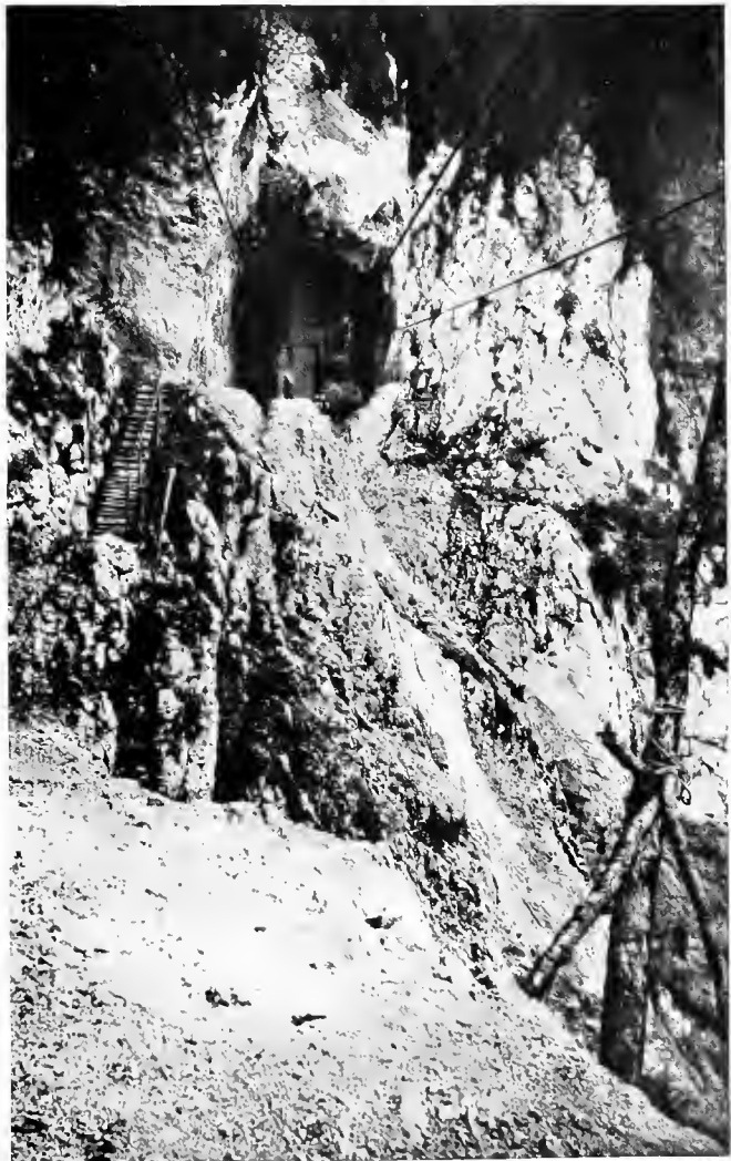
THE ENTRANCE TO THE TUNNEL ON THE SERVIAN LUMBER RAILWAY THROUGH WHICH THE AERIAL-WAY IS CARRIED TO OVERCOME A MOUNTAIN SPUR.
