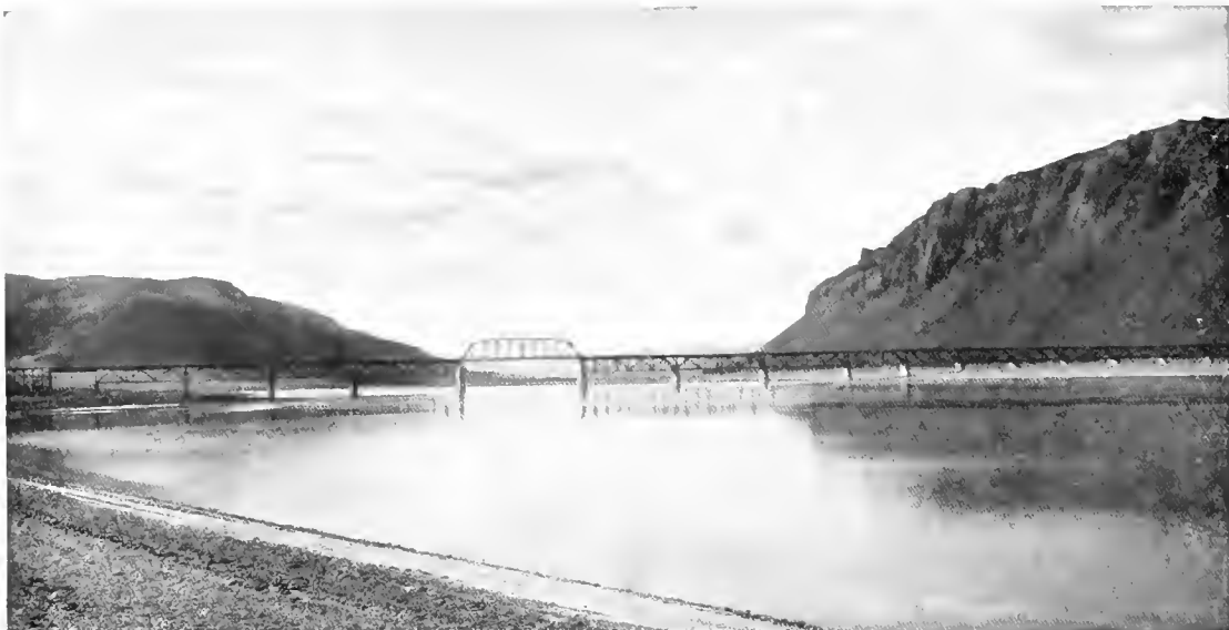
THE MASSIVE STEEL BRIDGE WHICH CARRIES THE CHICAGO, MILWAUKEE AND PUGET SOUND RAILWAY ACROSS THE COLUMBIA RIVER, NEAR BEVERLY, WASHINGTON.
