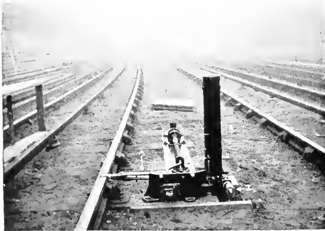
THE AUTOMATIC FOGGING APPARATUS FOR PLACING DETONATORS ON THE RUNNING RAIL.
