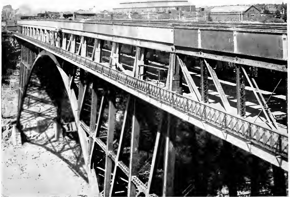
VIEW OF THE NIAGARA SPAN BRIDGE AFTER THE REMOVAL OF THE SUSPENSION BRIDGE. Showing top railway deck and lower deck for public use.
