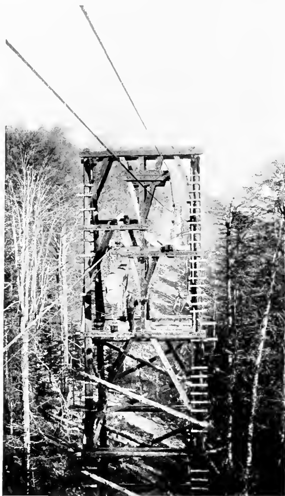
TYPICAL WOODEN TOWER SUPPORTING THE SERVIAN LUMBER AERIAL RAILWAY.
