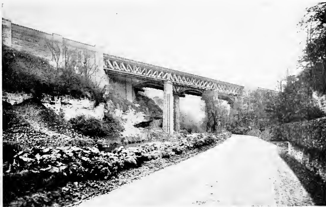
MILLER'S DALE VIADUCTS. 1905.
