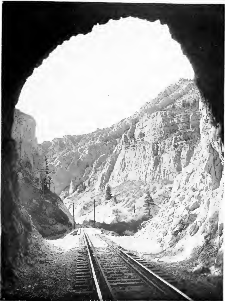
LOOKING ALONG THE LINE FROM ONE OF THE TUNNELS IN SIXTEEN-MILE CANYON, MONTANA.
