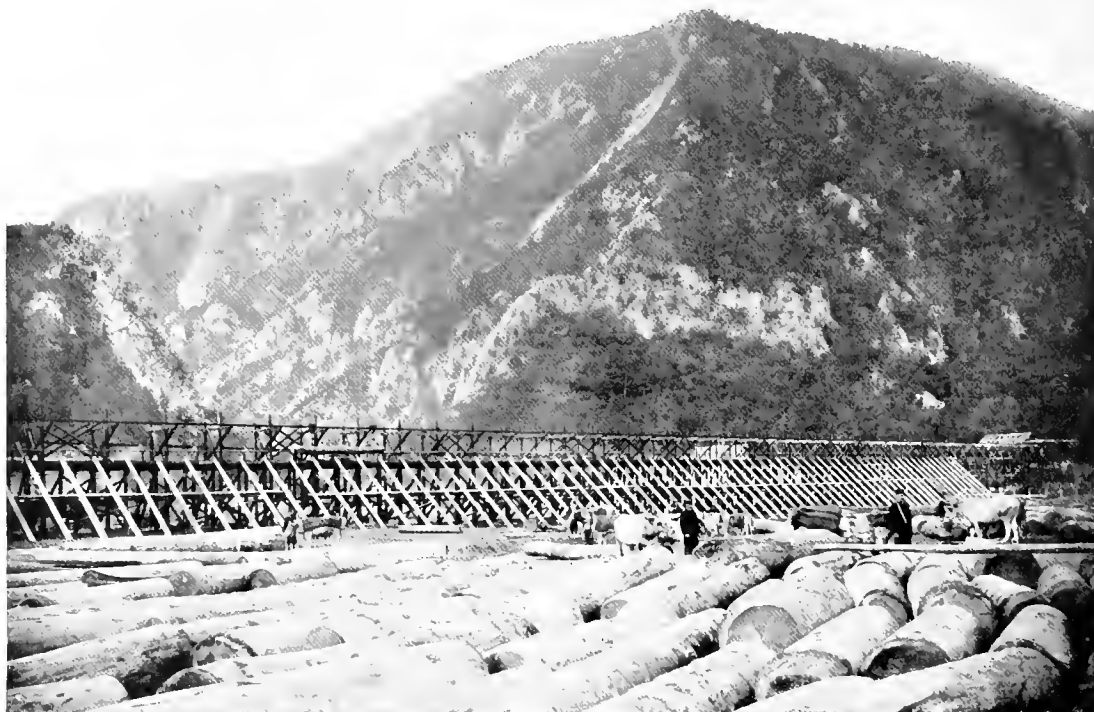
THE UNLOADING STATION OF THE SERVIAN LUMBER AERIAL RAILWAY UPON THE DRINA RIVER. The logs are made up into rafts and floated down the waterway.
