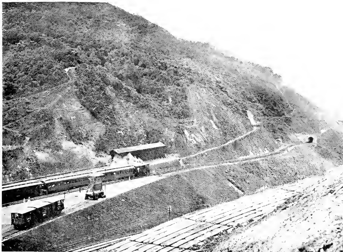
A BANKHEAD ON THE INCLINE SECTION OF THE SAN PAULO RAILWAY.
