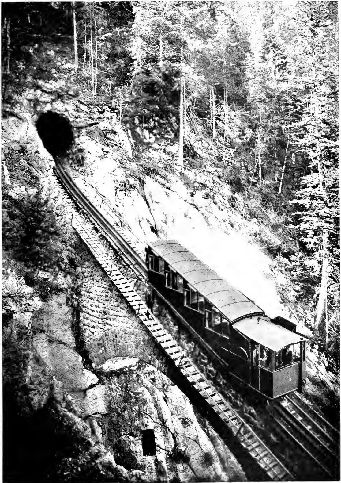
THE STIFFEST BANK ON THE PILATUS RAILWAY.
