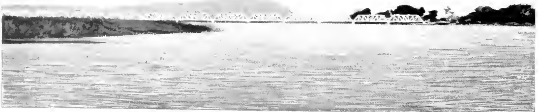
THE LONGEST BRIDGE IN AFRICA. ACROSS THE KAFUE RIVER.
