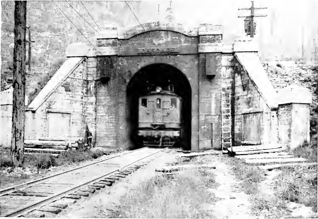
THE WESTERN MOUTH OF THE CASCADE TUNNEL, SHOWING ELECTRICALLY-DRAWN TRAIN EMERGING.
