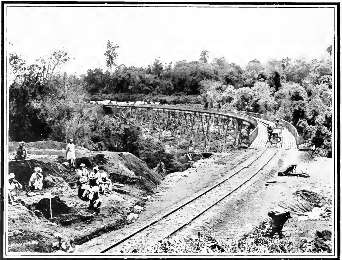
A BRIDGE CONSTRUCTION CAMP ON THE UGANDA RAILWAY.
