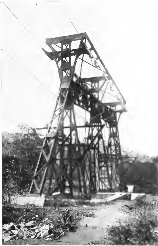
A TENSION STATION, SHOWING THE TOWERS WITH THE CONCRETE BLOCKS WHEREBY THE LINE IS KEPT TAUT.
