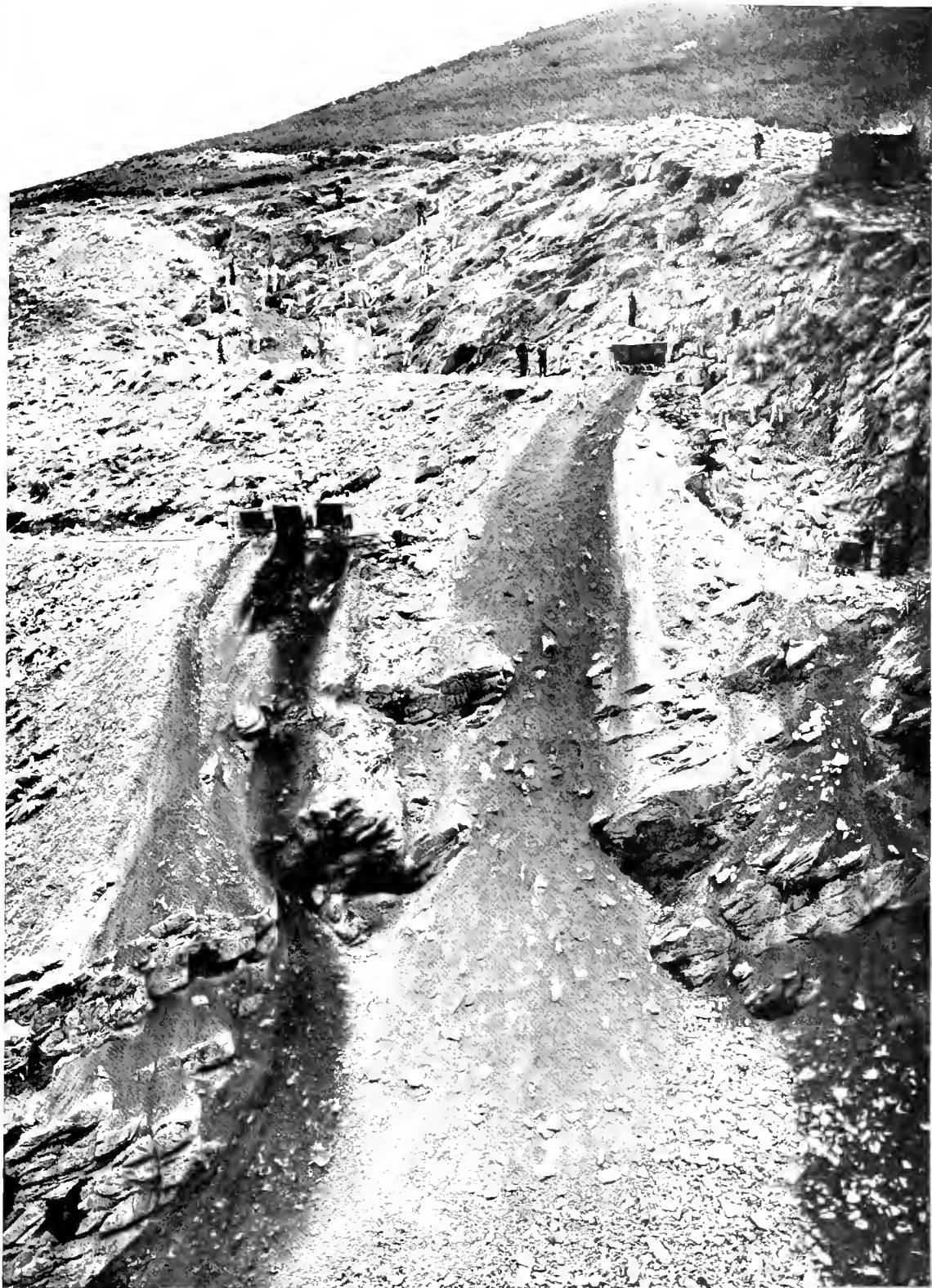
CONSTRUCTING THE RAILWAY OVER THE OULENIQUE MOUNTAINS BETWEEN GEORG AND OUDTSHOORN.
