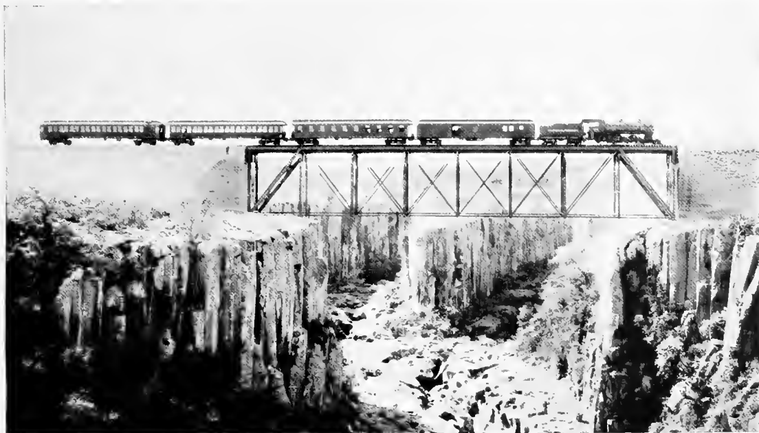
CHOÑE RIVER BRIDGE
