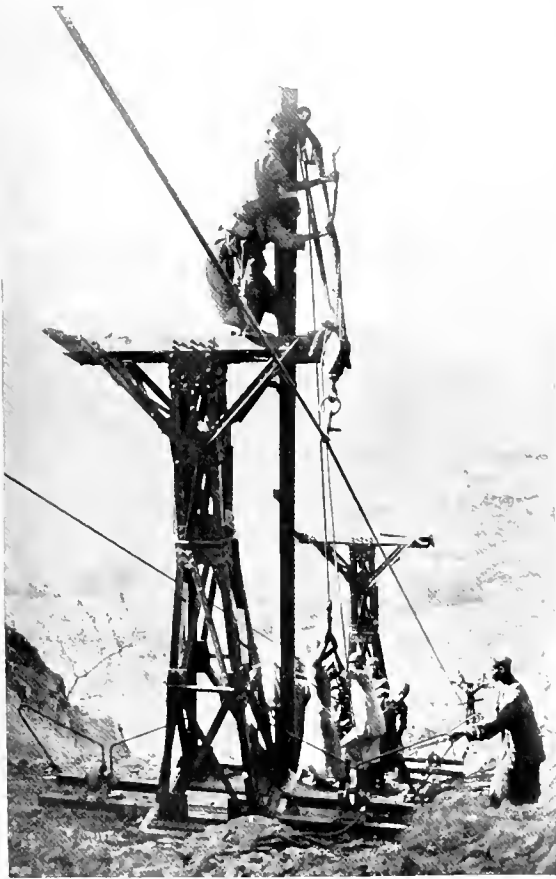
LIFTING THE CABLES UPON THE SUPPORTS.
