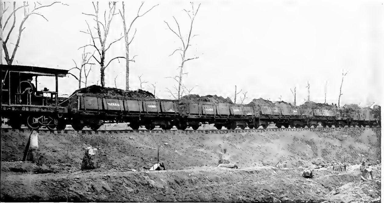
THE LIDGERWOOD UNLOADER. locomotive, and the necessary steam for driving the unloader is drawn from the boiler of the locomotive.
