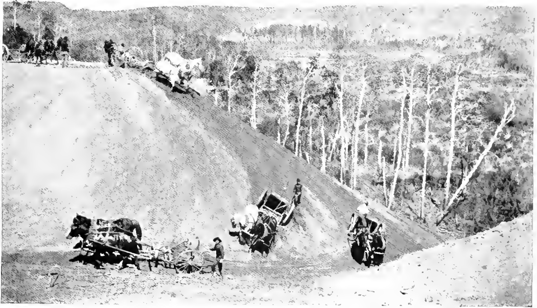
BUILDING A HIGH EMBANKMENT.
