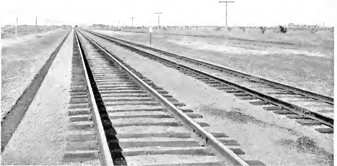
ROAD-BED BALLASTED WITH SHERMAN GRAVEL
