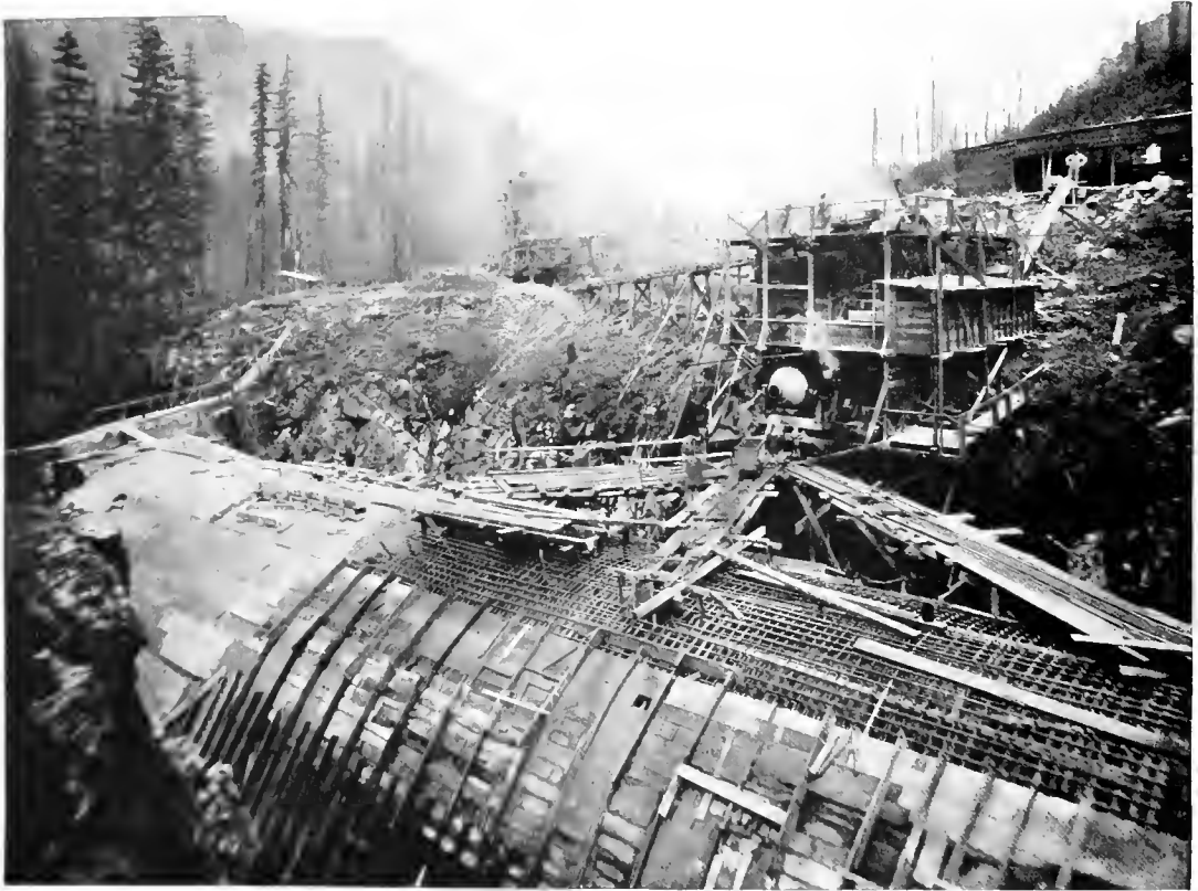
BUILDING THE PORTAL OF THE CASCADE TUNNEL.
