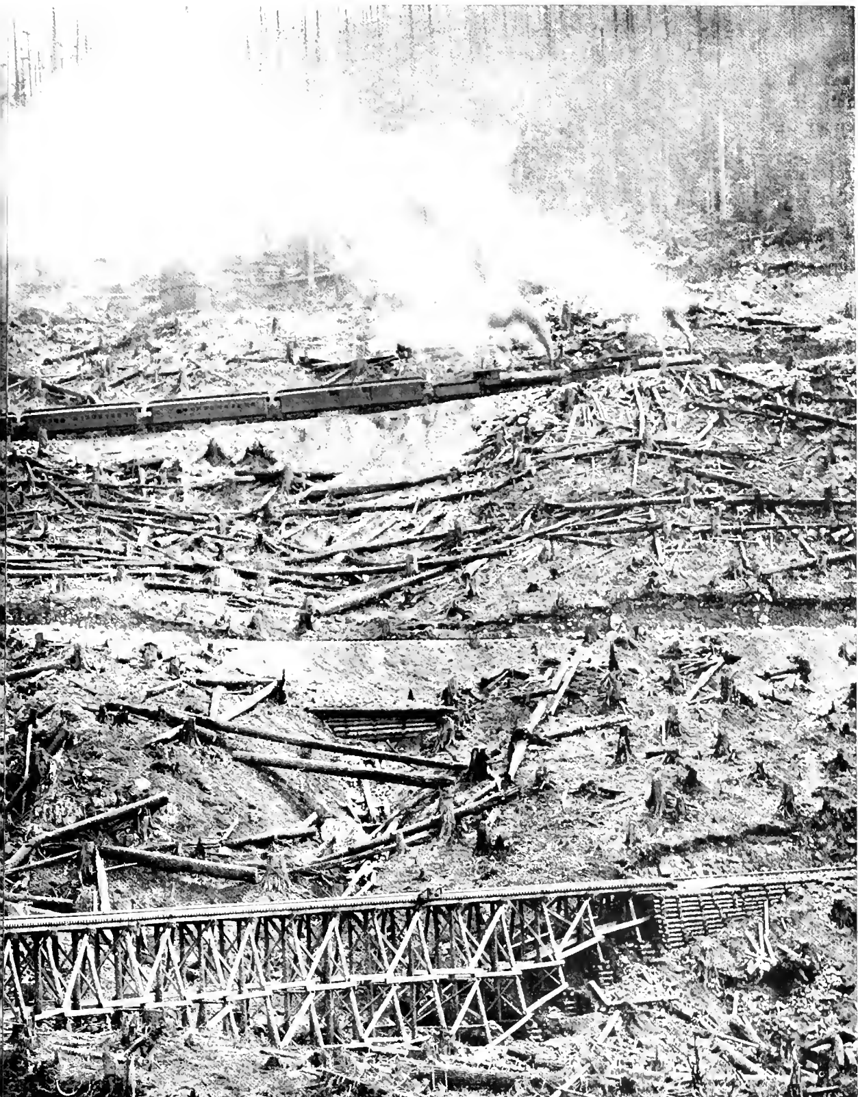
DURING THE PERIOD THE CASCADE TUNNEL WAS UNDER CONSTRUCTION, zig-zag by means of three locomotives. In the photograph four tracks are to be seen. This expensive directly the tunnel was completed.
