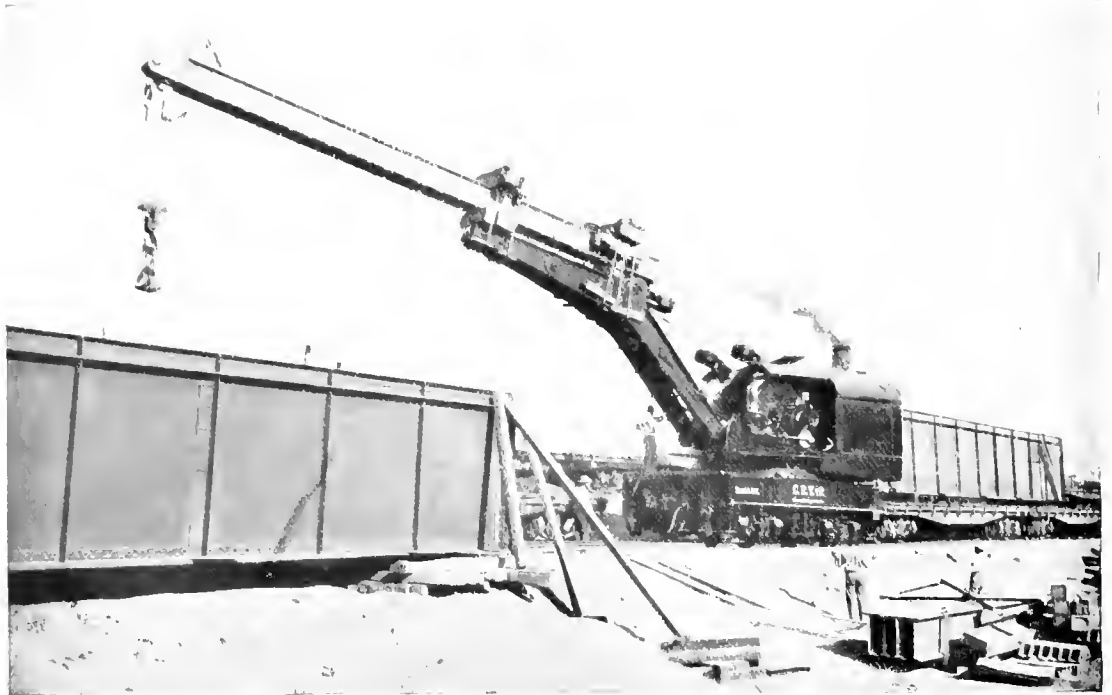
AN INDUSTRIAL WORKS WRECKING CRANE ADAPTED TO HANDLE AN AWKWARD LOAD. An extemporised boom attached to the crane-jib enabled this machine to place unaided an 80-foot girder weighing 20 tons.
