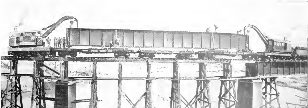
HOW WRECKING CRANES LOWER INTO POSITION A MASSIVE PLATE GIRDER.
