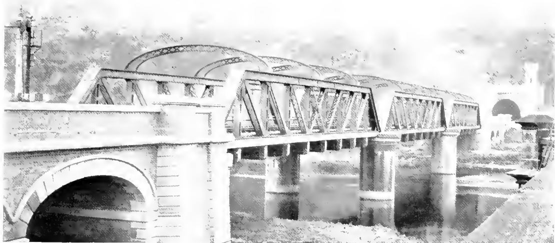
Photograph supplied by the Midland Railway Co. THE TRENT VIADUCT AND REDHILL TUNNEL. Showing the castellated portal.
