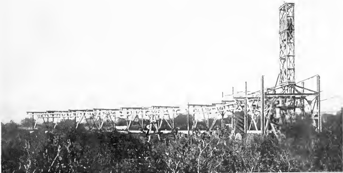
THE UNLOADING STATION, WHERE THE LUMBER IS TRANSFERRED TO THE STEAM LOCOMOTIVE RAILWAY FOR HAULAGE TO THE COAST.
