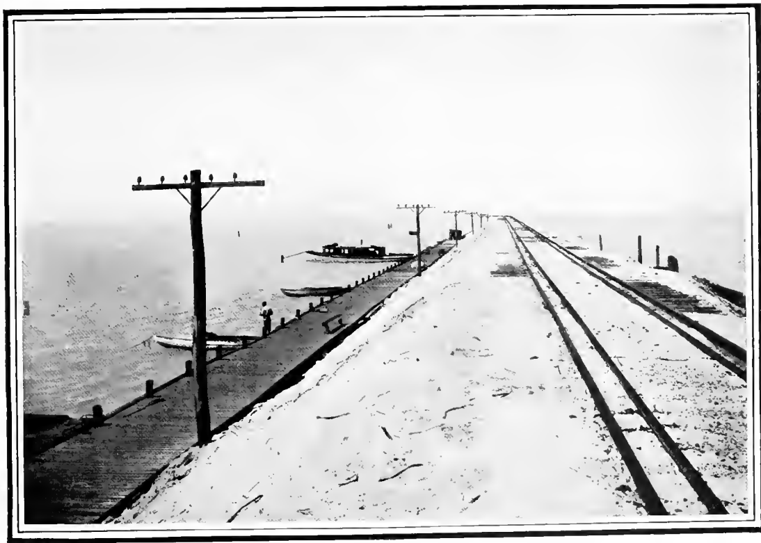
THE FINISHED EARTHEN EMBANKMENT IN THE "SHALLOWS" BETWEEN THE KEYS—AS SOLID AS A ROCK
