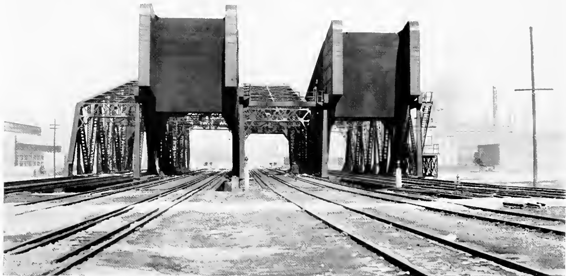
FOUR SINGLE-LEAF DOUBLE-TRACK SCHERZER ROLLING LIFT BRIDGES, SIDE BY SIDE, FORMING AN EIGHT-TRACK STRUCTURE ACROSS THE SHIP CANAL, CHICAGO.
