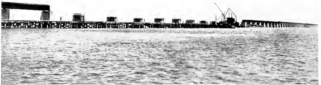
THE RAILWAY EAST OF PIGEON KEY, SHOWING PIERS AND BRIDGE CONSTRUCTION.
