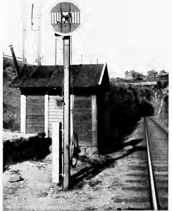
A DISTANT SIGNAL ON A SWEDISH RAILWAY FITTED WITH THE AGA FLASHLIGHT.
