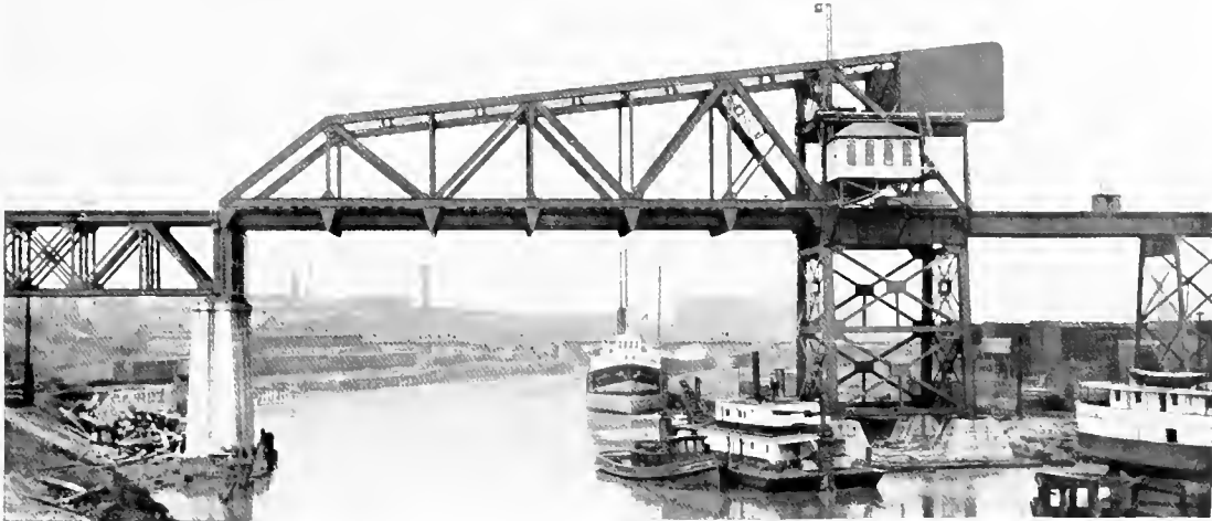
160-FOOT SINGLE-LEAF DOUBLE-TRACK SCHERZER ROLLING LIFT BRIDGE ACROSS THE CUYAHOGA RIVER AT CLEVELAND, OHIO, U.S.A., IN CLOSED POSITION.
