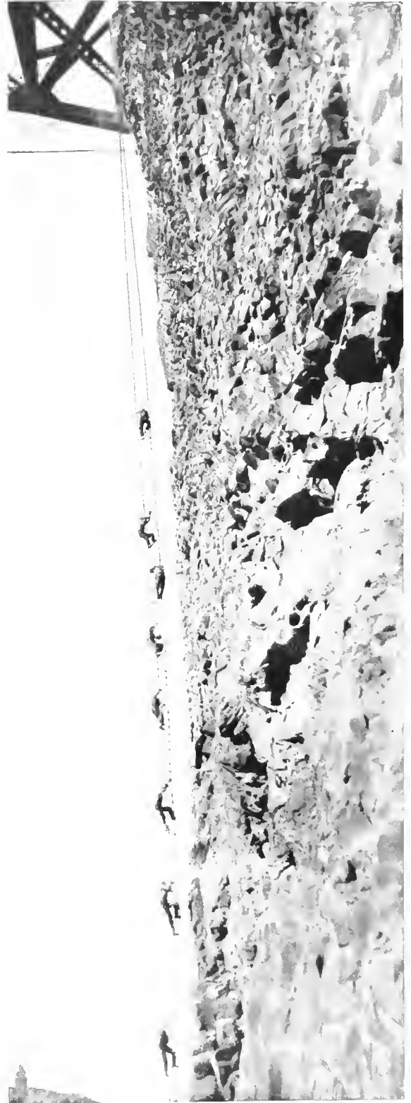
HOW THE "FLIES" WHO BUILT THE CROOKED RIVER CANYON BRIDGE REACHED THEIR WORK. A rope ladder was slung over the cliff communicating with the camp below.
