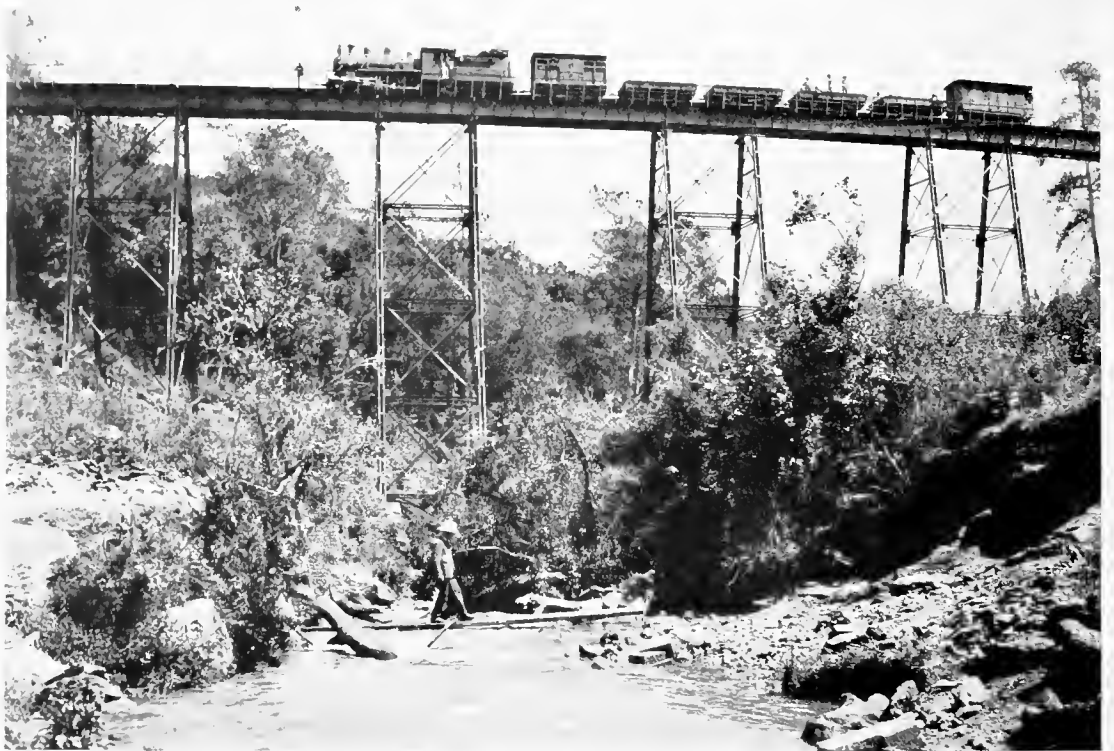
A STEEL TRESTLE BRIDGE ON THE UGANDA RAILWAY.
