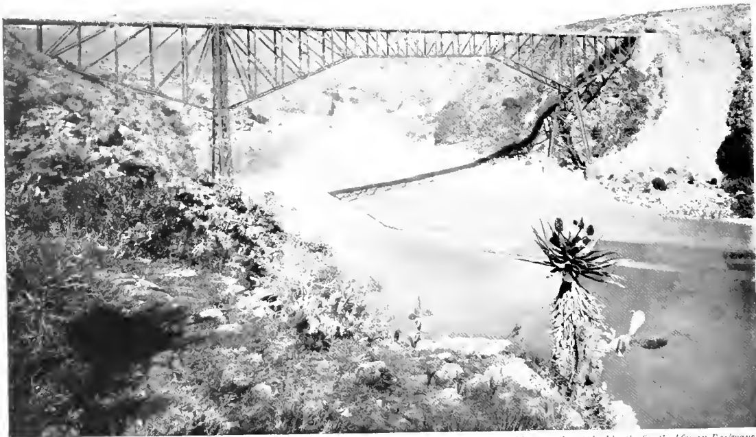
CANTILEVER BRIDGE SPANNING THE GOURITZ RIVER, NEAR MOSSIE BAY.
