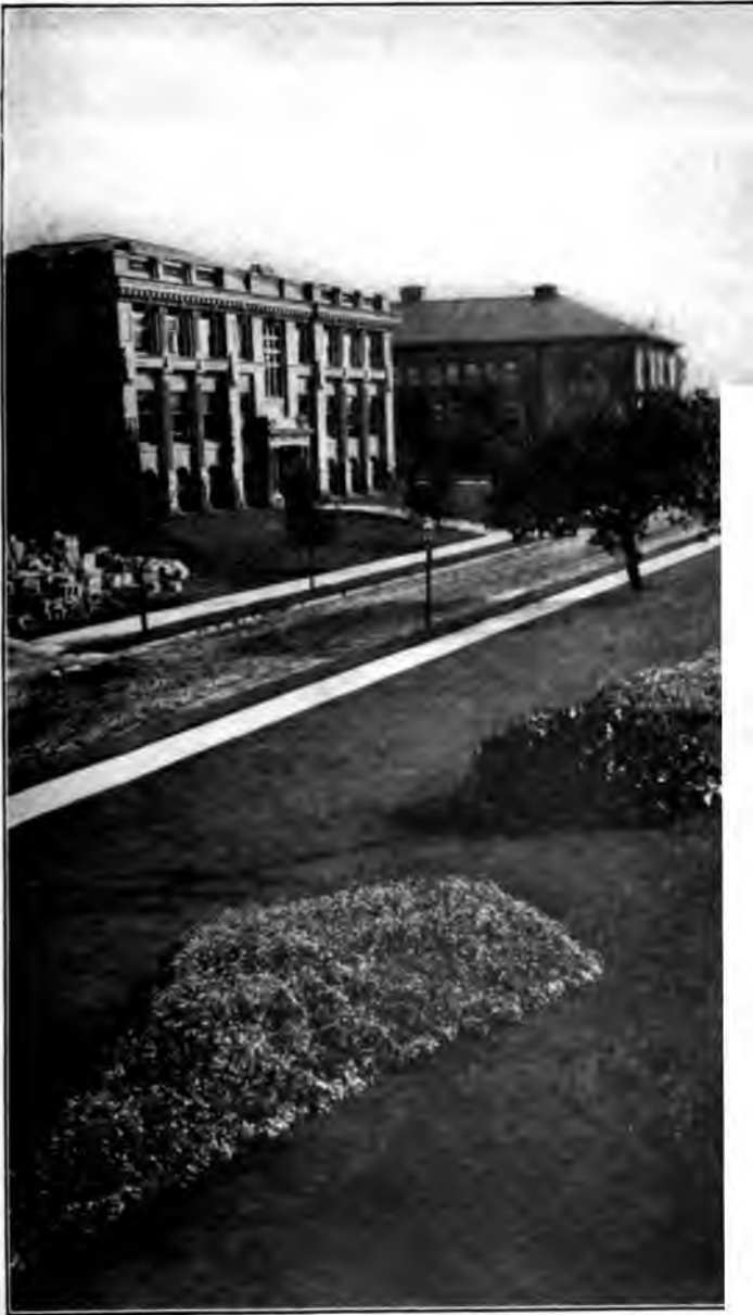
PHYSICS AND CHEMISTRY BUILDINGS University of Minnesota
