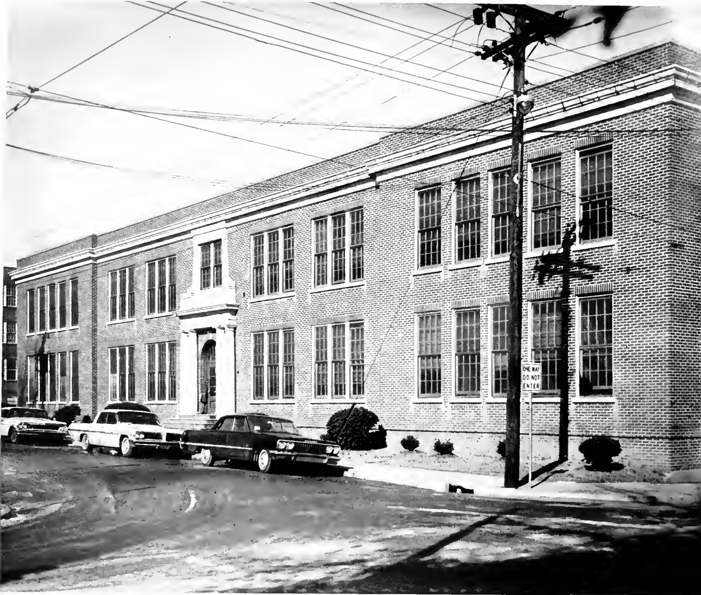
CAROLINA HALL-Classroom Building
