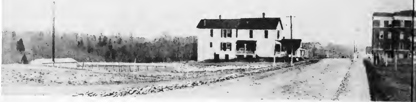
Central Heating Plant
