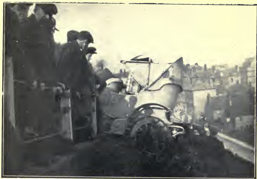
A Motor dash over the Slope Road.
