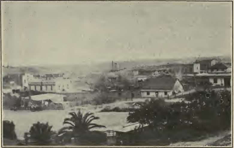
GENERAL VIEW OF YUMA, ARIZONA.
