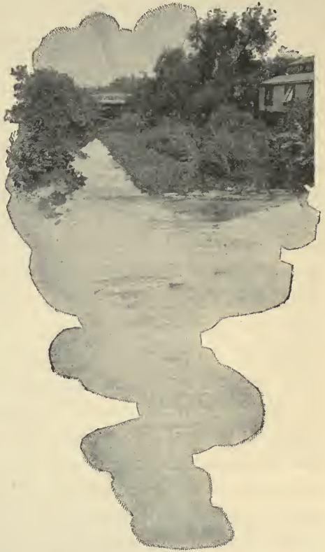
CROCKET STREET BRIDGE OVER SAN ANTONIO RIVER.
