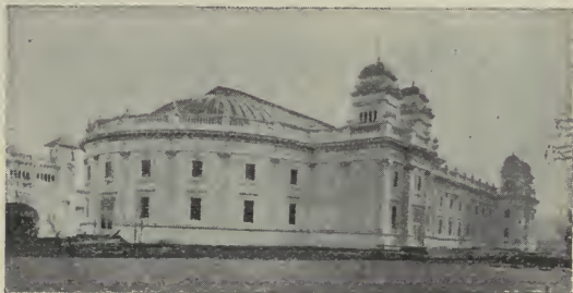
ORIENTAL EXHIBIT BUILDING.
