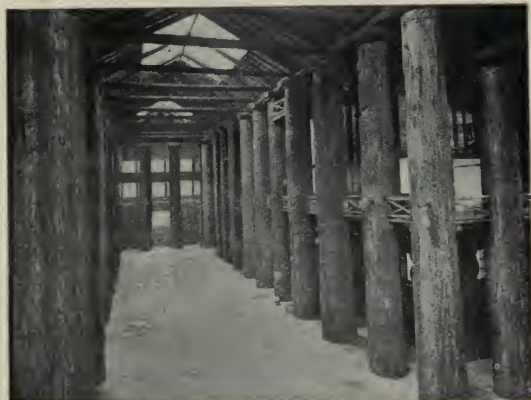
INTERIOR OF THE FORESTRY BUILDING
