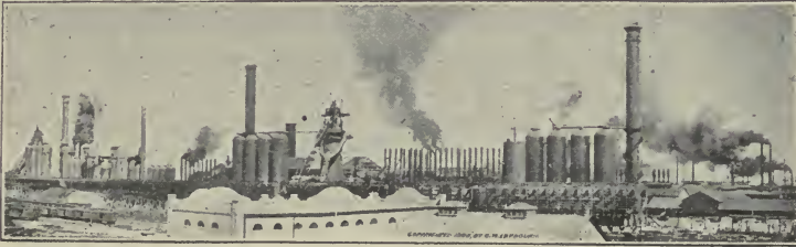
THE MINNEQUA STEEL WORKS, PUEBLO.
