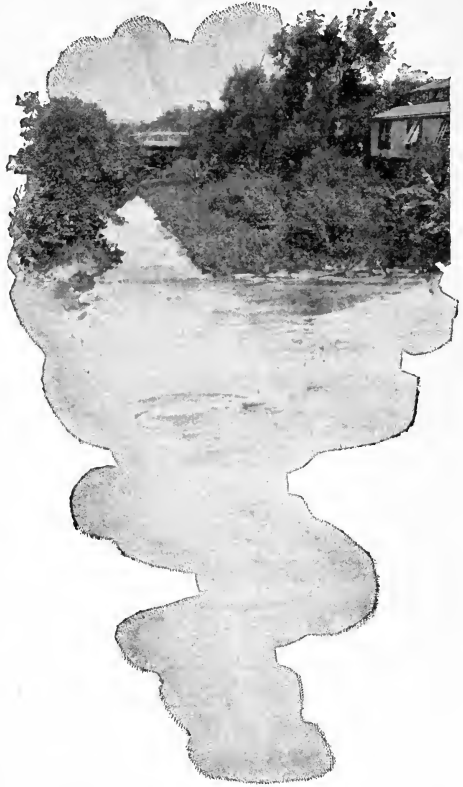
CROCKET STREET BRIDGE OVER SAN ANTONIO RIVER.
