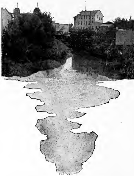
A RIVER BRIDGE, SAN ANTONIO.
