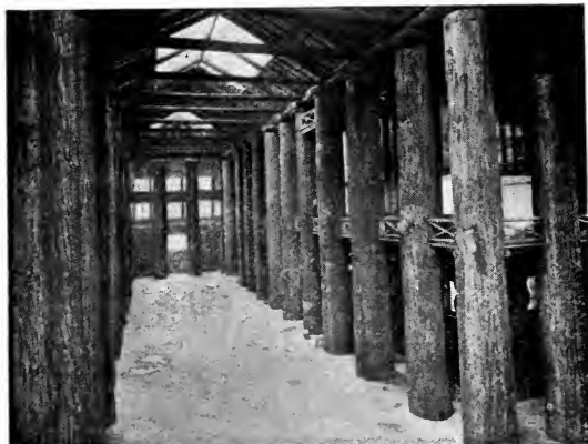
INTERIOR OF THE FORESTRY BUILDING
