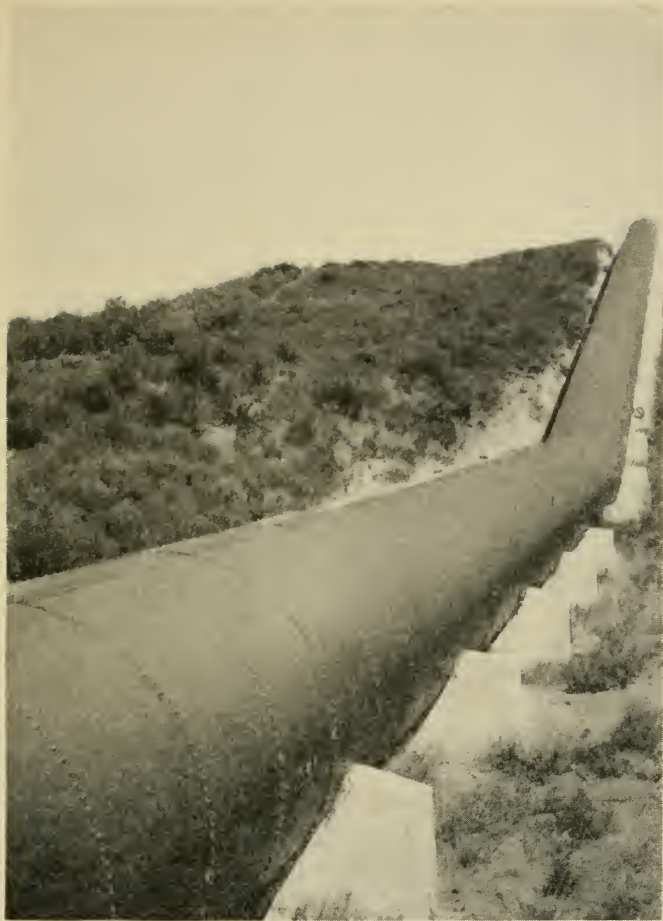
PORTION OF THE OWEN'S ACQUEDUCT
