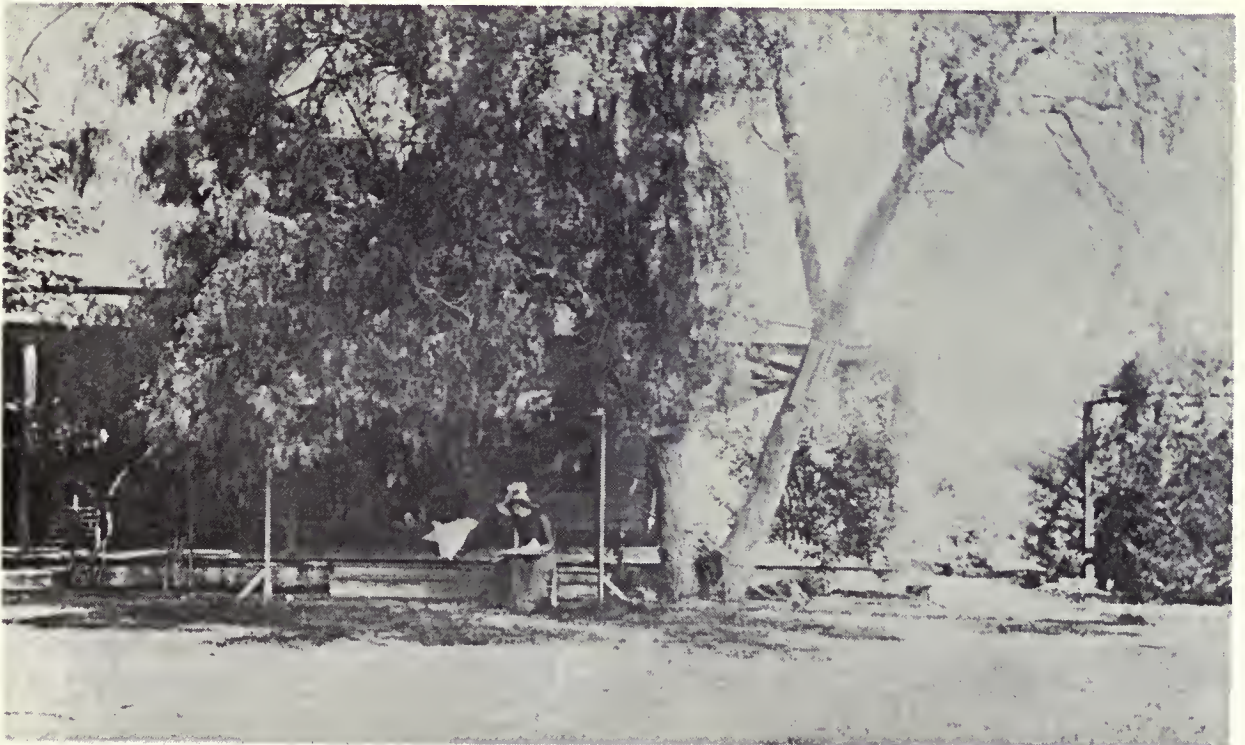
Georgia Schweitzer in front of the porch of the Brandenstein home, with an unidentified individual in a hammock just behind.
