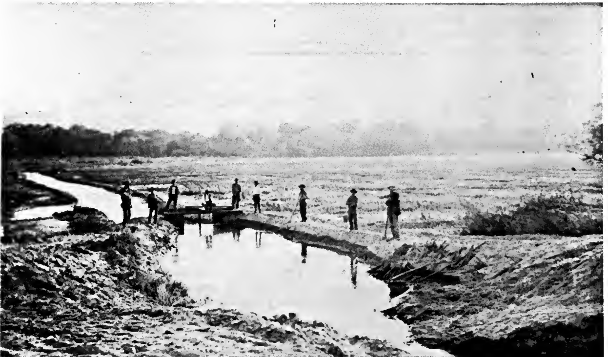
The irrigation canal built under Meyer Brandenstein's direction came to be known to later generations as "Grandpa's ditch."
