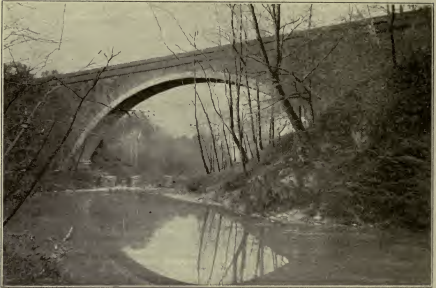
THE CABIN JOHN BRIDGE. — Length of Span, 220 Feet; Height, 57 Feet.
