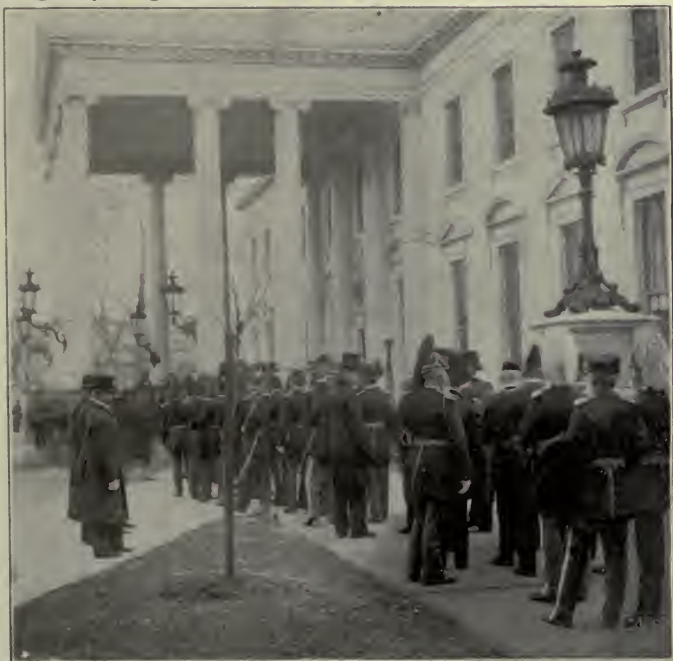
IN LINE ON A RECEPTION DAY.—At the White House.
