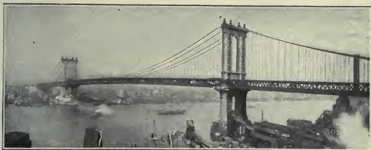
Manhattan Bridge Bowery and Canal St., Manhattan Flatbush Ave., Brooklyn Page 10
