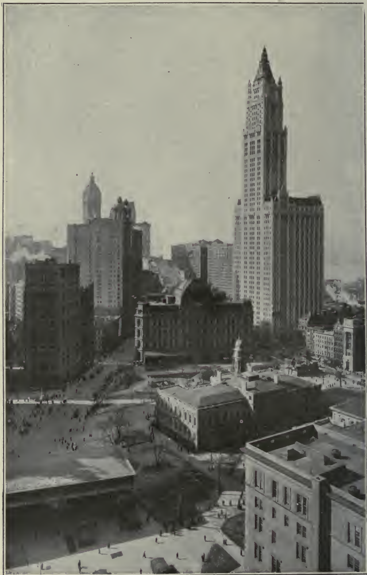
Looking South from Municipal Building
