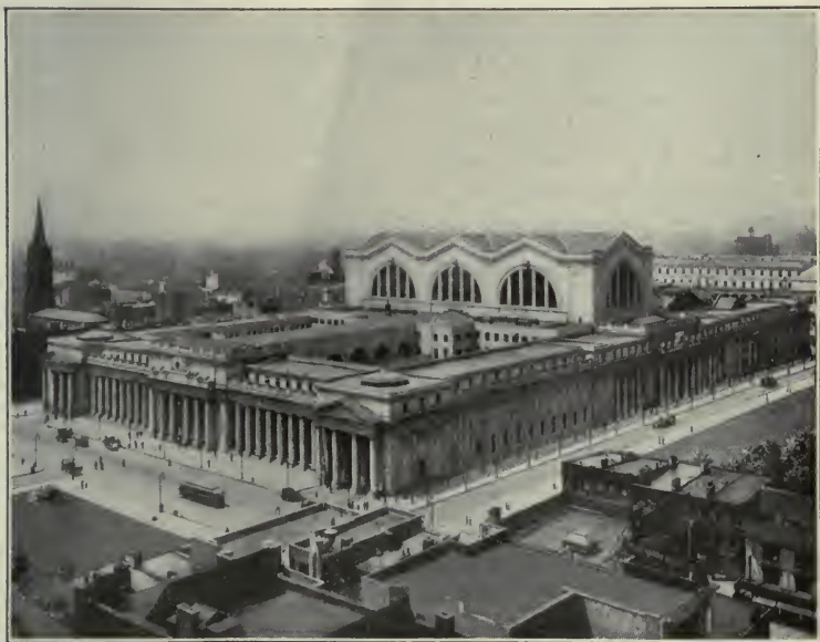
Pennsylvania Station Seventh Ave., 32d to 33d Street
