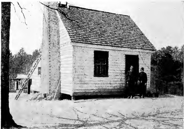
TYPICAL HOUSE WITH "MUD-AND-STICK" CHIMNEY
