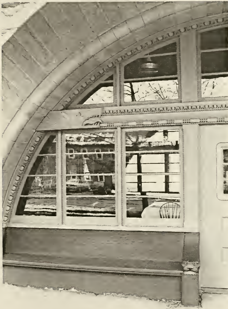
FIGURE 28: Detail of exterior of Old Colony Railroad Station, track side elevation.
