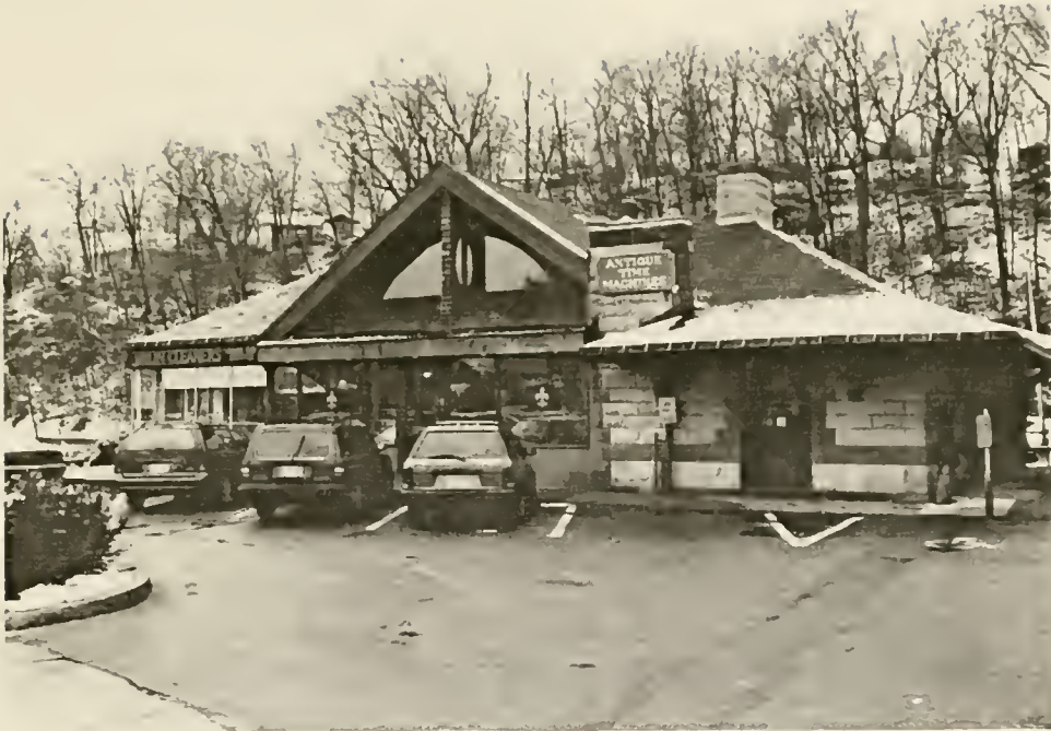
FIGURE 23: Street (west) elevation, Wellesley Hills Station.
