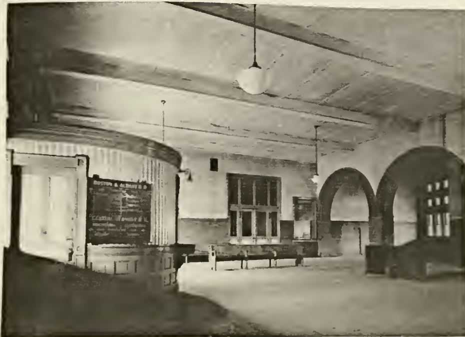
FIGURE 52: Photograph of interior of Union Passenger Station.
