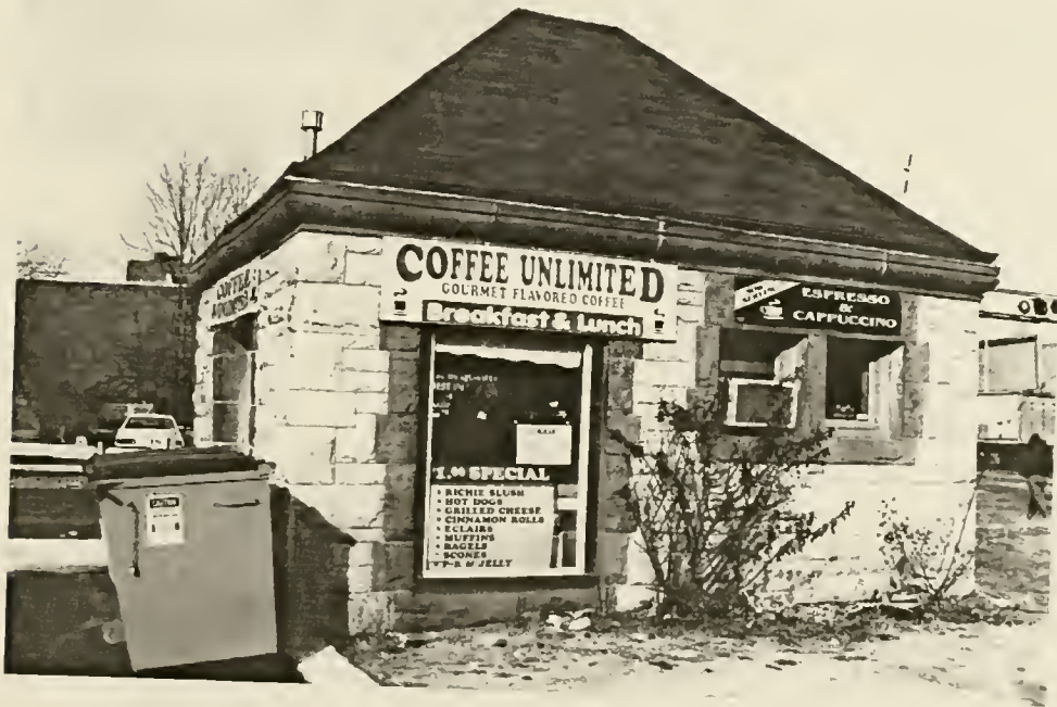
FIGURE 68: South Framingham Station, secondary building.
