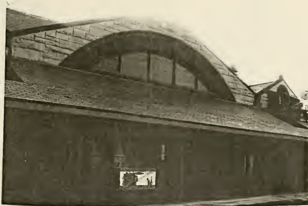
FIGURE 67: South Framingham Station.
