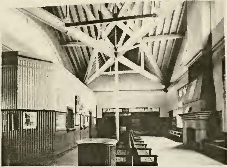
FIGURE 63: Historic American Buildings Survey Photograph of South Framingham Station interior.
