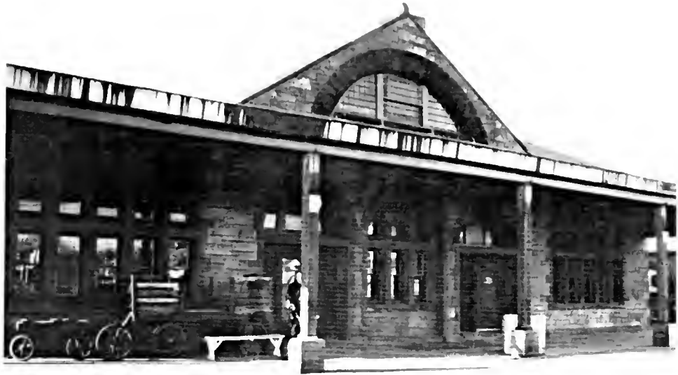
FIGURE 53: Union Passenger Station.
