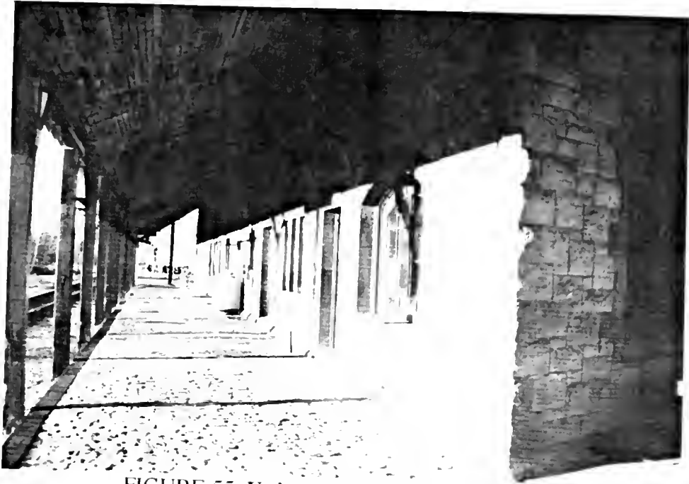
FIGURE 55: Union Passenger Station.
