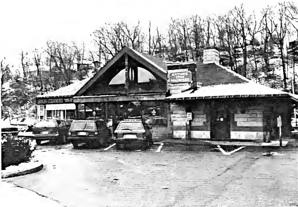
FIGURE 23: Street (west) elevation, Wellesley Hills Station.
