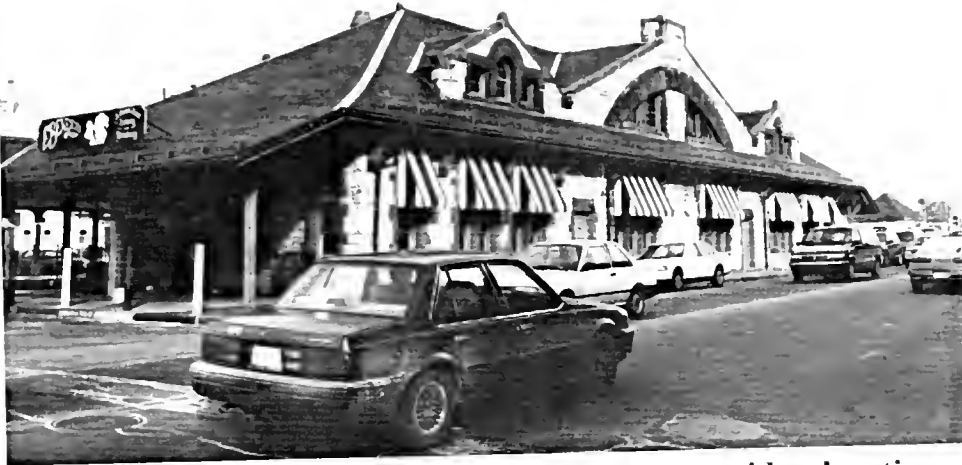
FIGURE 65: South Framingham Station, street-side elevation.
