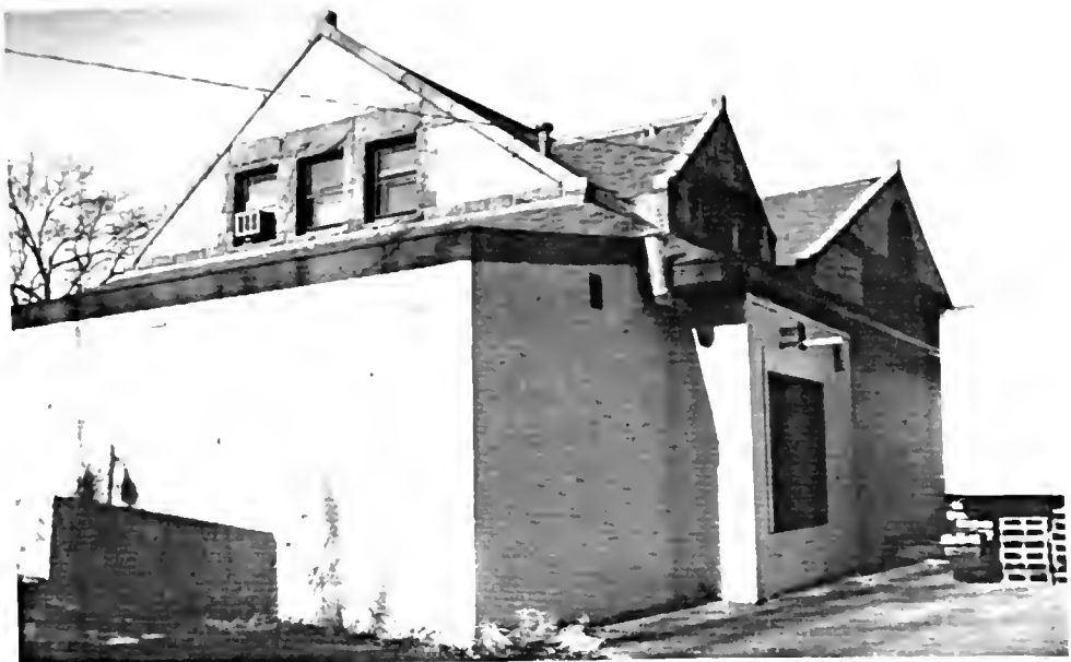
FIGURE 43: Connecticut River Railroad Station, alterations.
