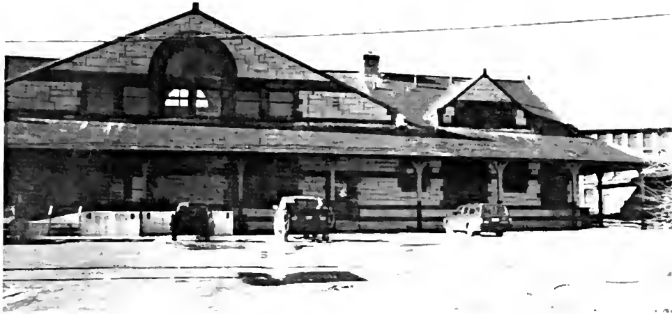
FIGURE 41: Connecticut River Railroad Station.
