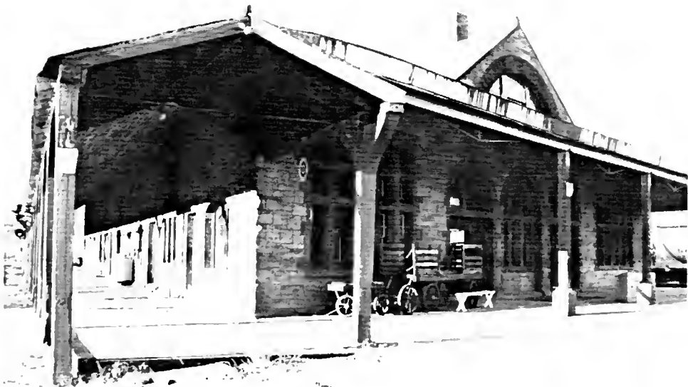
FIGURE 54: Union Passenger Station.
