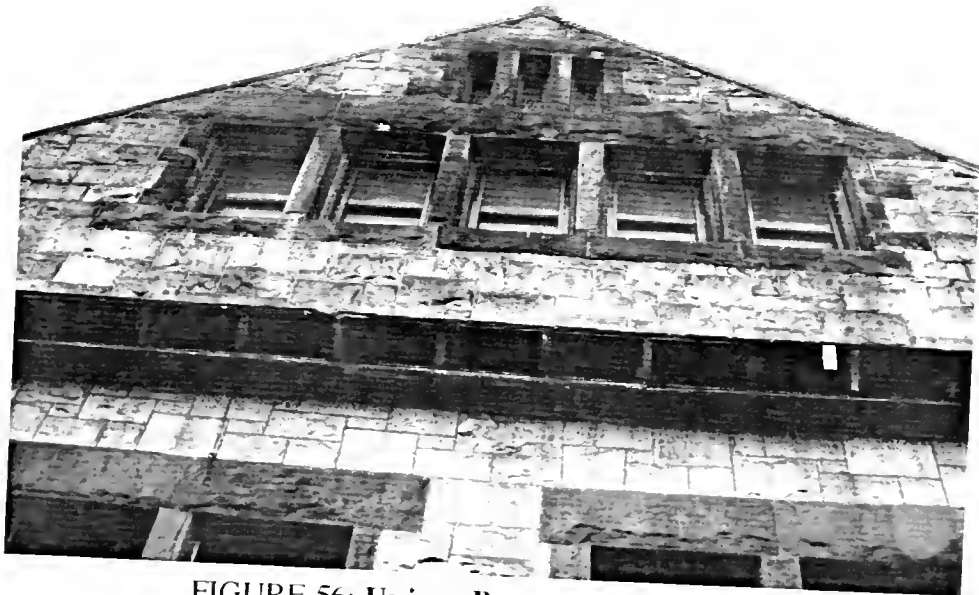
FIGURE 56: Union Passenger Station.
