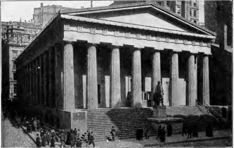
THE SUB-TREASURY AT WALL AND NASSAU STREETS, NEW YORK, BUILT ON THE SITE OF THE OLD FEDERAL HALL
