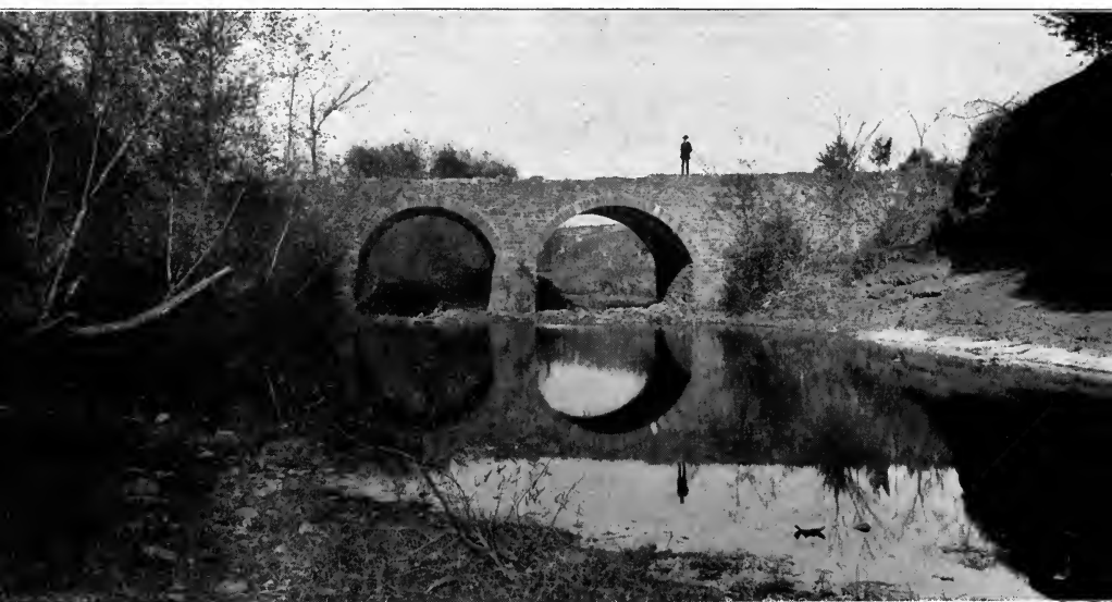
THE STONE BRIDGE AT BULL RUN
