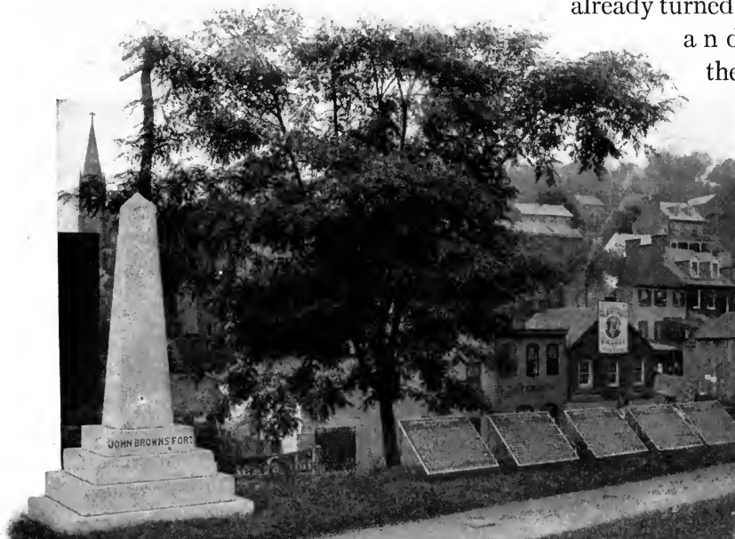
THE SITE OF JOHN BROWN'S FORT AT HARPER'S FERRY
