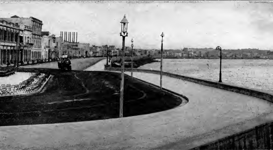
THE MALECON, HAVANA'S NEW SEA WALL, BUILT SINCE AMERICAN INTERVENTION
