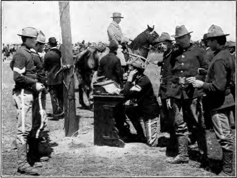
A TELEPHONE STATION IN THE FIELD AT SANTIAGO
