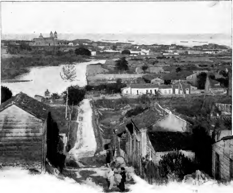
GENERAL VIEW OF MATANZAS AND HARBOR
