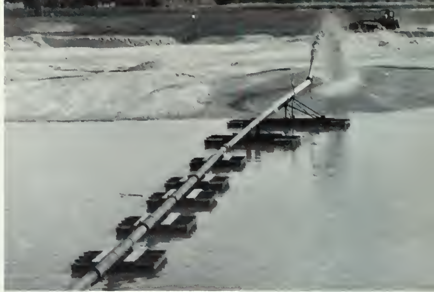
Figure 30—Desander being utilized in land forming
