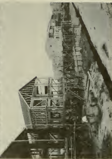
C-5. Upper left - CBS first floor, wood frame second floor; upper right - neighboring CBS both floors with concrete tie beams and tie columns - no failures of walls, but window and door failures; lower left - rebuild - replacing former wood frame second floor with CBS; lower right - new construction in Garden City, South Carolina. It should be noted that despite some "shoddy construction" in South Dade county, the great majority of the houses that were heavily damaged were still better built far better than the great majority of the homes along the Gulf of Mexico and Atlantic coasts from Texas through Maine.
