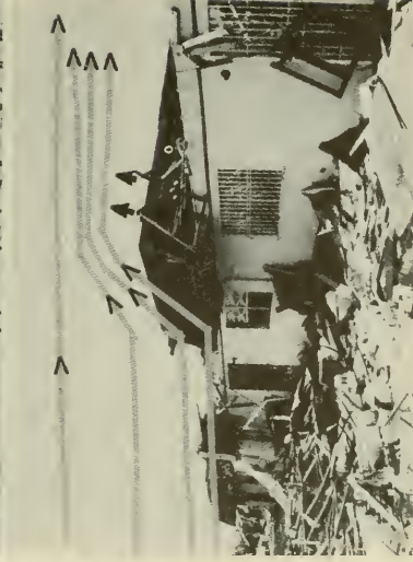
C-2. Upper left - Steel reinforced poured concrete tiebeam with steel roof straps exposed; upper right - streak of damage in senior citizen housing where tiebeams with roofs became airborne; lower left and lower right - Naranja Lakes complex where roofs acted similar to airplane wings lifting the roof and the tie beams off the buildings.
