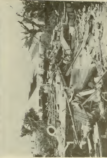
C-4. Upper left - Mobile home park with well built CBS community building where 17 people rode out the hurricane across from the Naranja Lakes development in figure 4; upper right - close up of senior citizen housing in background of picture to the left - note some shutters failed and others were not present, but building stood; lower right - Padeland Mobile Home park - some 31 people rode out the hurricane in the community building; lower right - floor of mobile home still tied down - failures were the structures, not the tie downs, even for those that had additional straps across the top of the mobile home - note conventional CBS structures still standing in the background.
