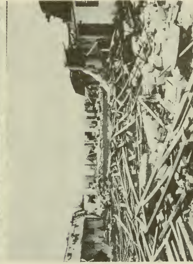
C-2. Upper left - Steel reinforced poured concrete tiebeam with steel roof straps exposed; upper right - streak of damage in senior citizen housing where tiebeams with roofs became airborne; lower left and lower right - Naranja Lakes complex where roofs acted similar to airplane wings lifting the roof and the tie beams off the buildings.
