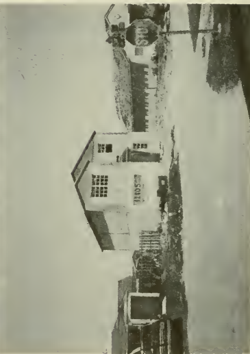
C-5. Upper left - CBS first floor, wood frame second floor; upper right - neighboring CBS both floors with concrete tie beams and tie columns - no failures of walls, but window and door failures; lower left - rebuild - replacing former wood frame second floor with CBS; lower right - new construction in Garden City, South Carolina. It should be noted that despite some "shoddy construction" in South Dade county, the great majority of the houses that were heavily damaged were still better built far better than the great majority of the homes along the Gulf of Mexico and Atlantic coasts from Texas through Maine.
