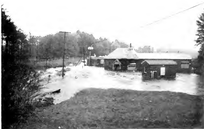
Receding floodwater at Water Treatment Plant - October, 1996
