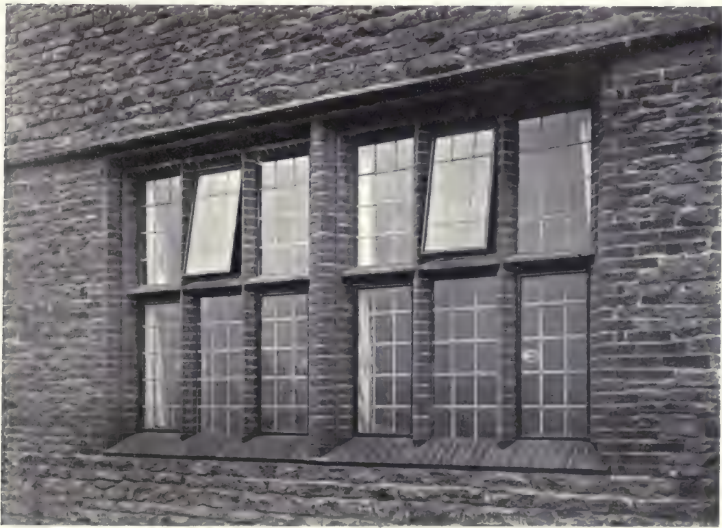
TUESLEY COURT, GODALMING, SURREY: EXTERIOR AND INTERIOR VIEWS OF DRAWING-ROOM WINDOW.
