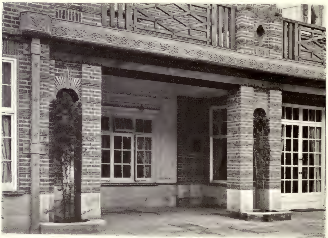
“EAST WEALD,” HAMPSTEAD : DETAIL OF SOUTH FRONT.
