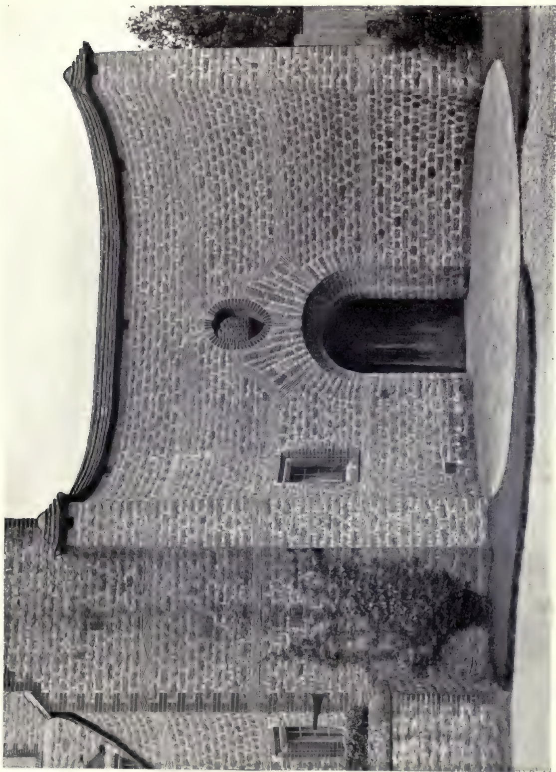
The walling is of Bargate stone, with creasing courses in tiles, and pieces of ironstone put in the mortar joints, following a local custom.
