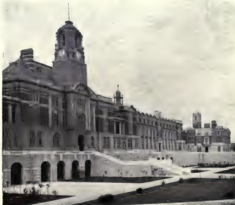
The Britannia Royal Naval College, Dartmouth. Expanded Metal Lathing used throughout for Plasterwork.
