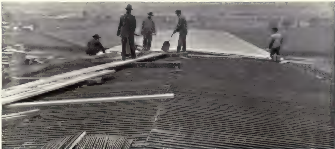
Hy-Rib Roof in course of construction.
