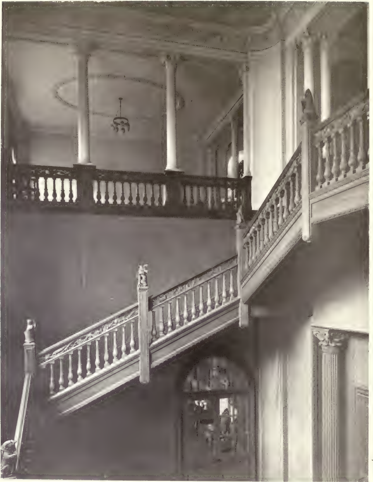
NEW STAIRCASE AT KINFAUNS CASTLE, PERTH.
