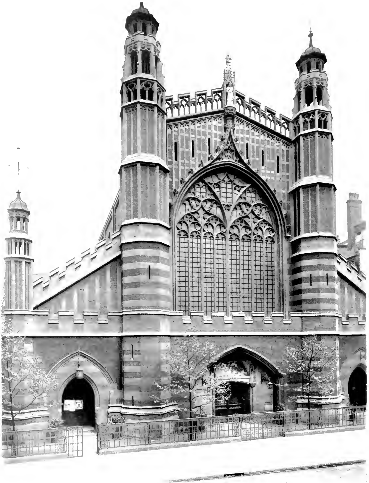
WEST FACADE, 10, LOANS STREET
