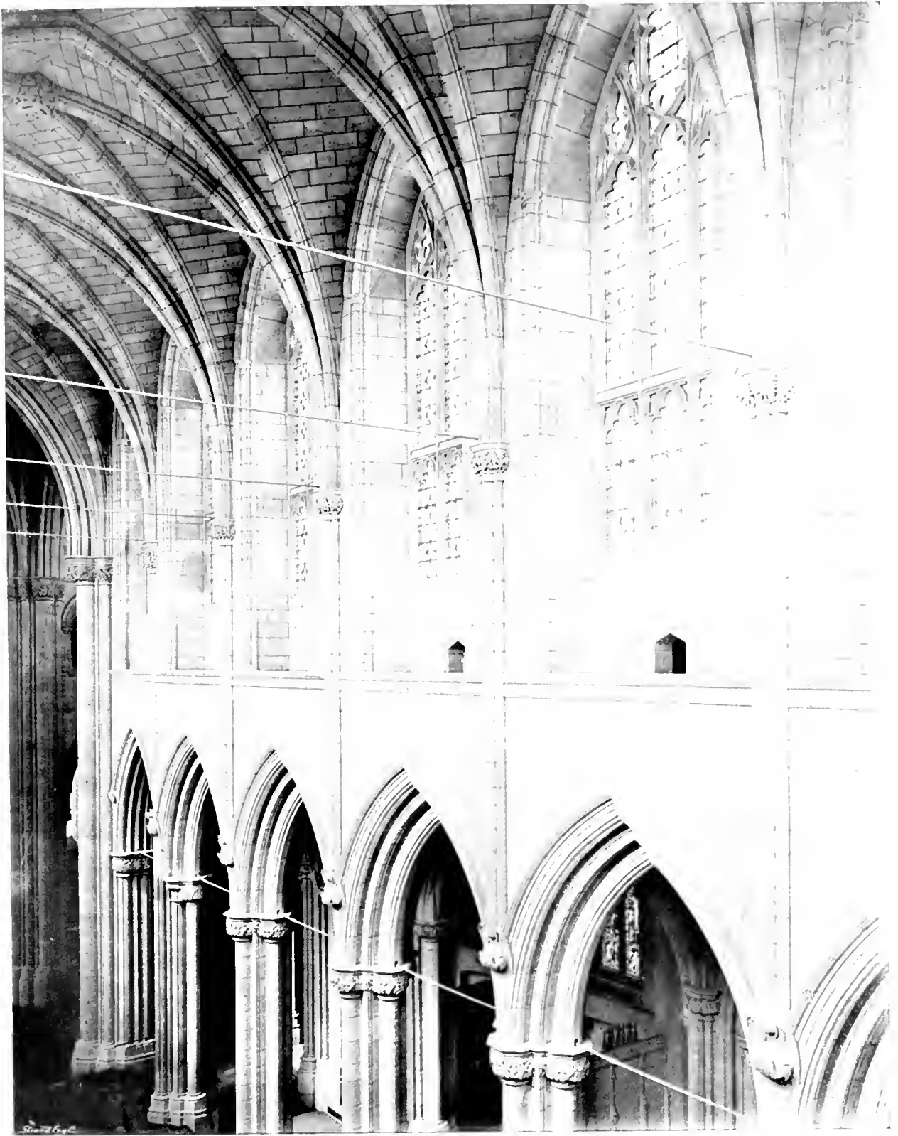
THE TRIFORIUM AND CLEARSTORY WINDOWS.
