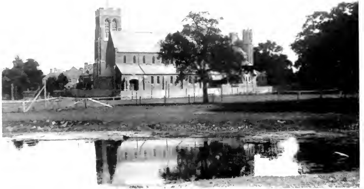
GENERAL VIEW FROM SOUTH-WEST.
