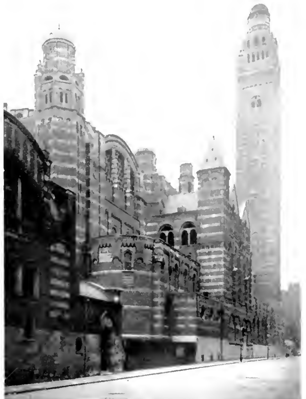
VIEW LOOKING NORTH-WEST.
