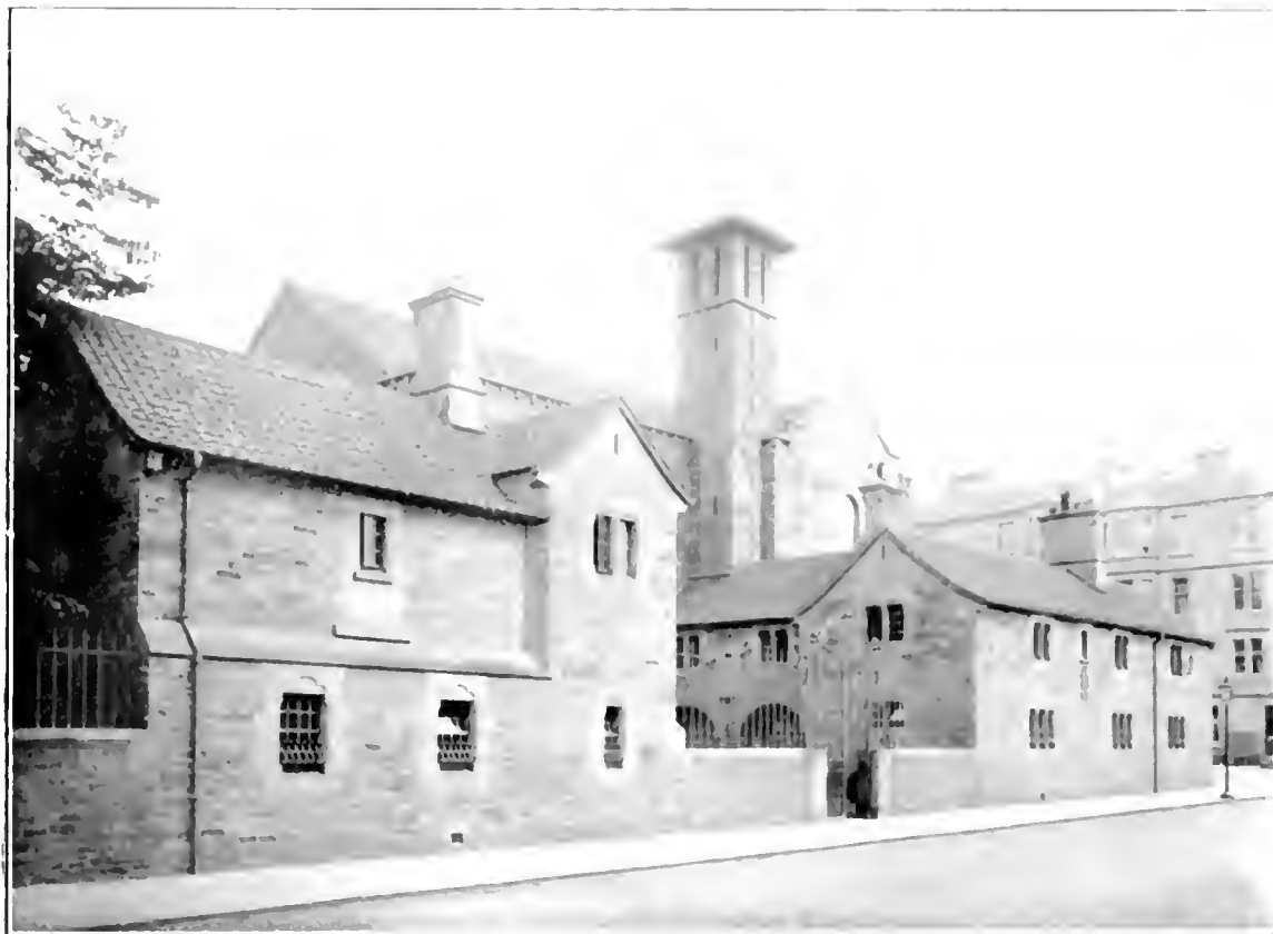
VIEW FROM NORTH EAST
