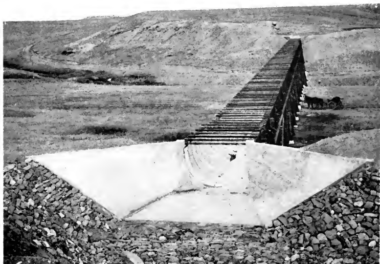
FLUME ON FISHER CANAL BLACKFEET PROJECT, MONTANA
