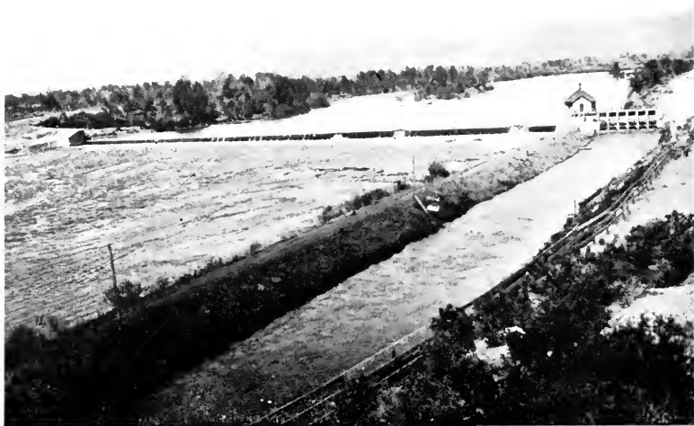
DIVERSION DAM IN YAKIMI RIVER, HEADGATES, AND GATE TENDER'S HOUSE ON THE SUNNYSIDE CANAL YAKIMA PROJECT, WASHINGTON
