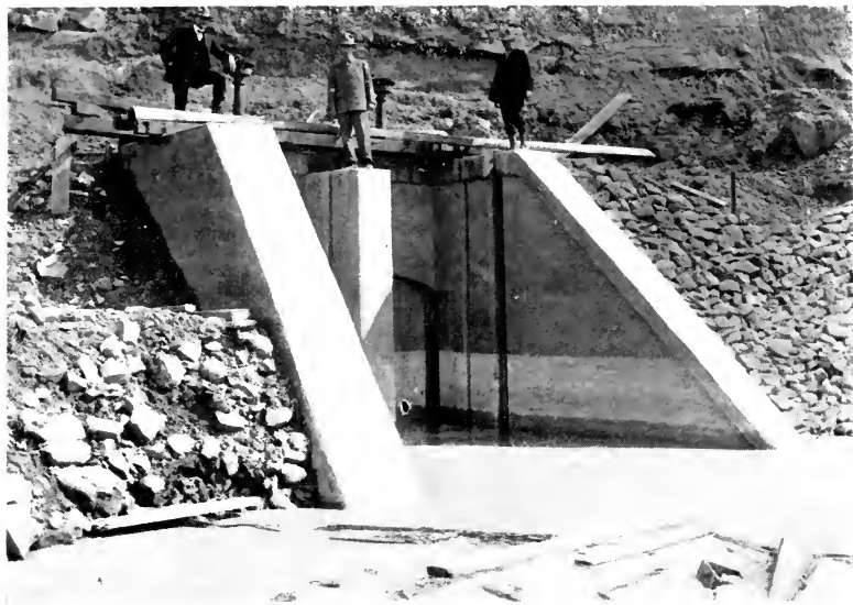
HEADGATE, SHOWING GATE STANDS, YELLOWSTONE RIVER HUNTLEY PROJECT, MONTANA
