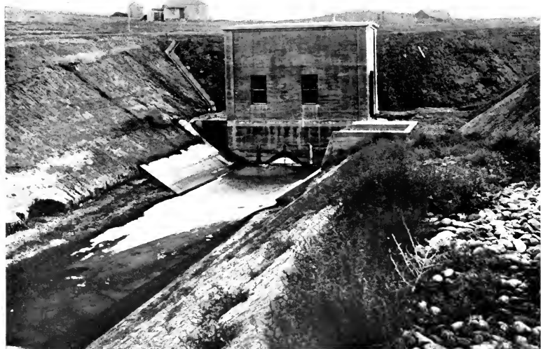
DIRECT PUMPING PLANT HUNTLEY PROJECT, MONTANA
