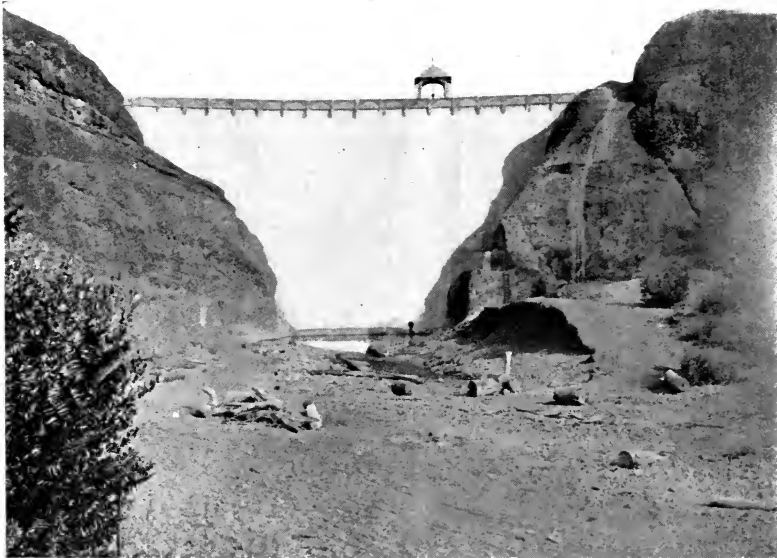
EAST PARK DAM, DOWNSTREAM FACE—HEIGHT 127 FEET, LENGTH OF CREST 220 FEET ORLAND PROJECT, CALIFORNIA
