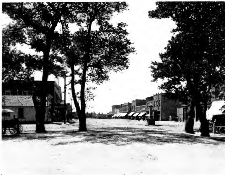
THE CITY OF FALLON ON WHAT WAS ONCE THE CARSON DESERT TRUCKEE-CARSON PROJECT, NEVADA
