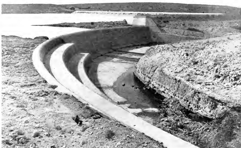
AVALON DAM AND SPILLWAY CARLSBAD PROJECT, NEW MEXICO
