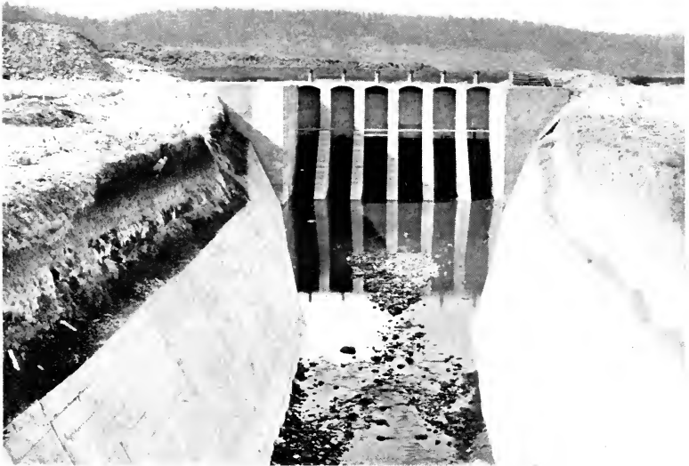
INTAKE GATES OF MAIN CANAL KLAMATH PROJECT, OREGON-CALIFORNIA
