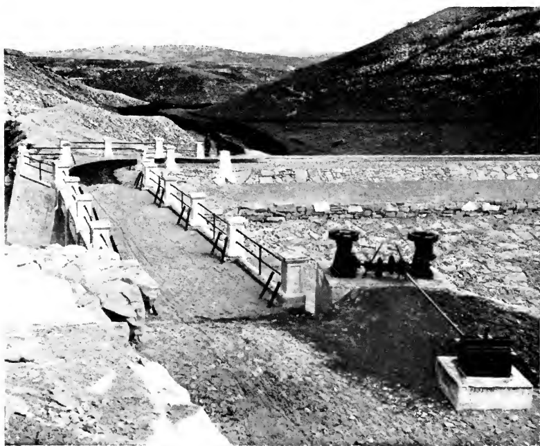
BRIDGE ACROSS WASTEWAY AT NORTH END OF STRAWBERRY DAM STRAWBERRY VALLEY PROJECT, UTAH
