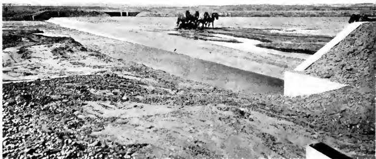
DAM ON POPLAR RIVER
