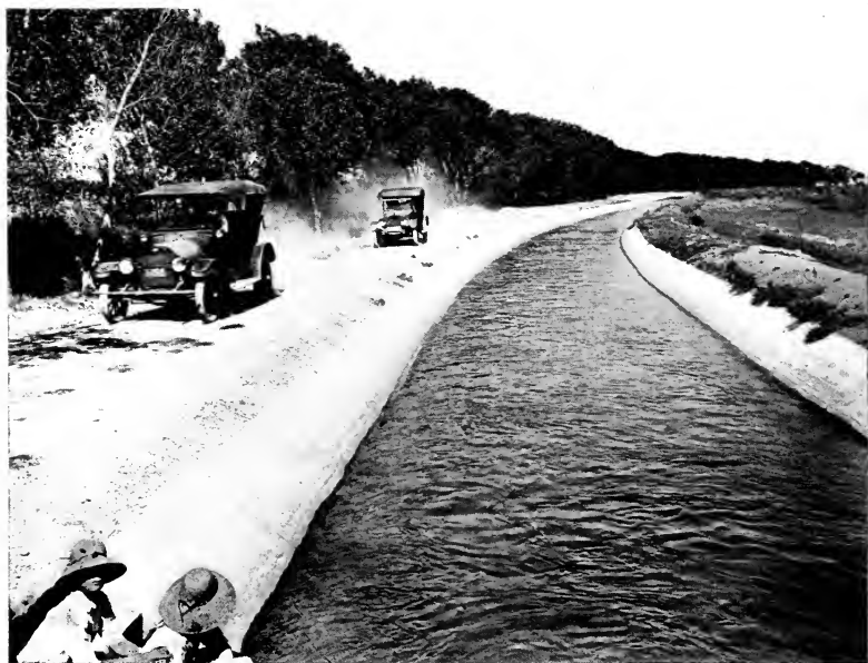
CEMENT LINED SECTION MAIN CANAL CARLSBAD PROJECT, NEW MEXICO
