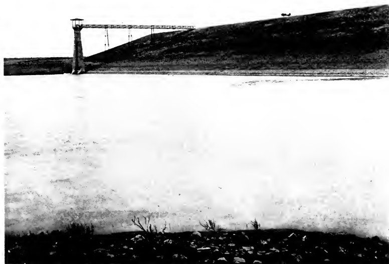
COLD SPRINGS DAM, RESERVOIR, AND OUTLET TOWER UMATILLA PROJECT, OREGON
