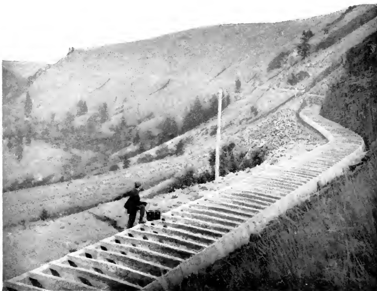
MAIN TIETON CANAL, TIETON CANYON, 600 FEET ABOVE THE STREAM YAKIMA PROJECT, WASHINGTON
