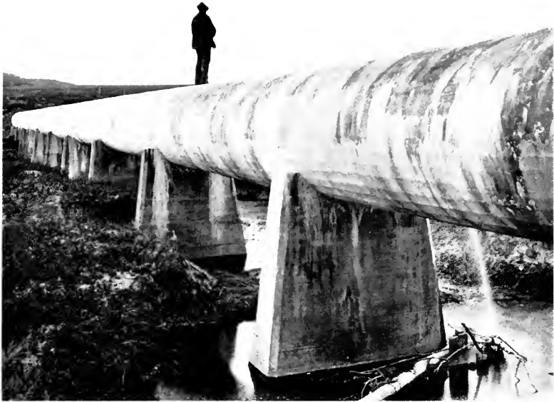
SIMM'S CREEK PRESSURE PIPE, FORT SHAW UNIT SUN RIVER PROJECT, MONTANA
