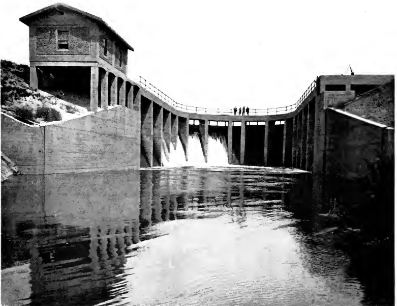
LOST RIVER DAM KLAMATH PROJECT, OREGON-CALIFORNIA
