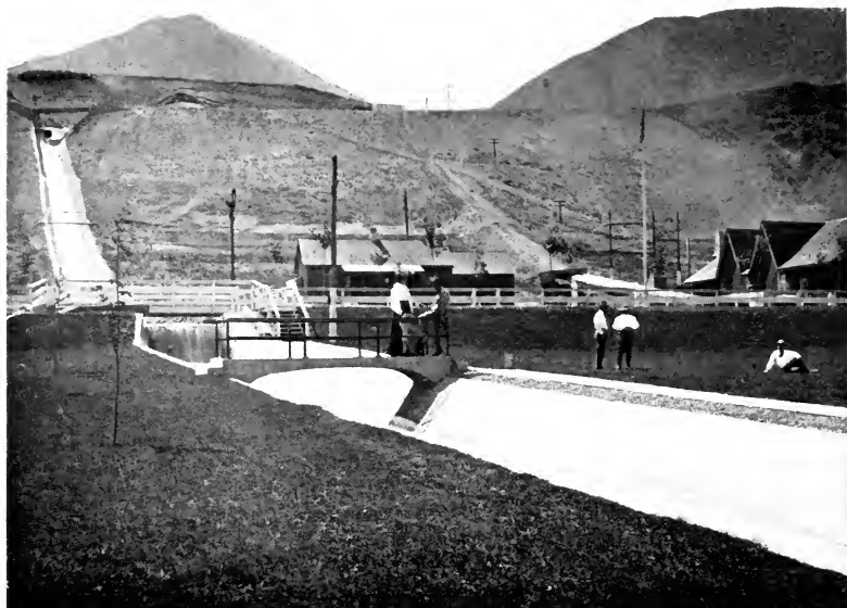
POWER-HOUSE AND WASTEWAY CHUTE STRAWBERRY VALLEY PROJECT, UTAH
