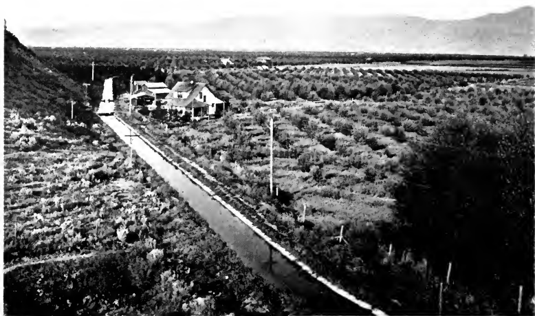
VISTA FROM ROUND TOP HILL BACK OF WHITE RANCH OKANOGAN PROJECT, WASHINGTON
