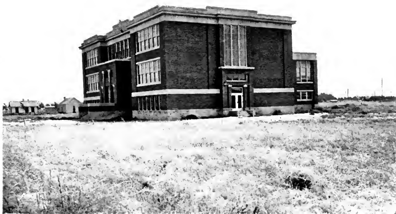
ELECTRICALLY HEATED HIGH SCHOOL AT RUPERT MINIDOKA PROJECT, IDAHO
