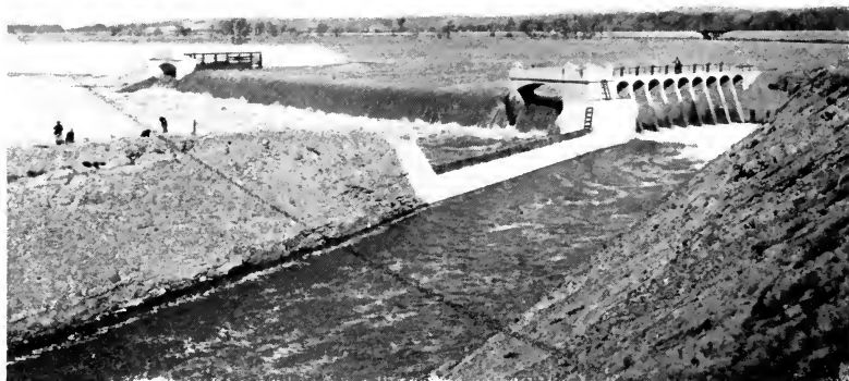
WILALEN DIVERSION DAM AND HEADWORKS NORTH PLATTE PROJECT, NEBRASKA-WYOMING
