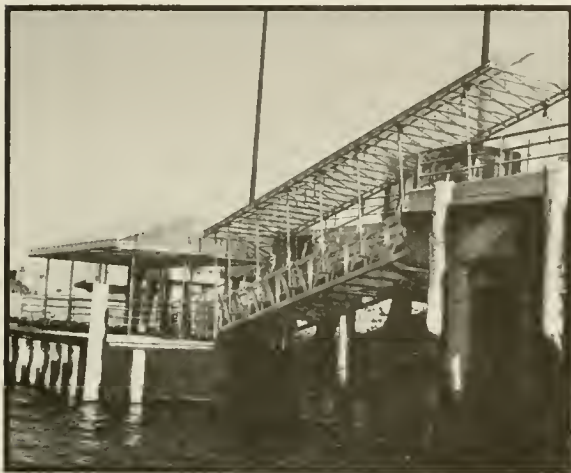
Gangway, Float, and Canopy
