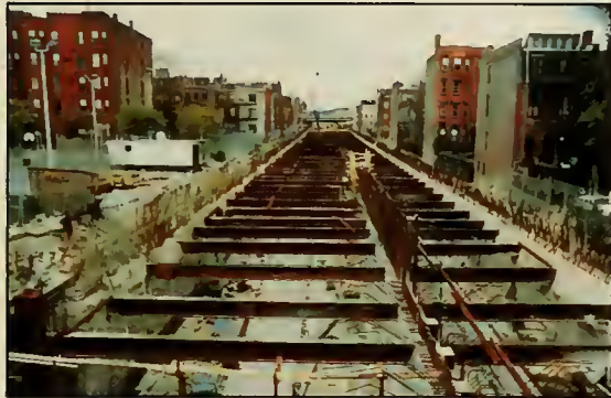
Temporary Bracing—Slurry Wall
