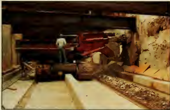
Slurry Wall Under Construction
