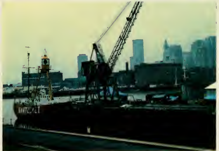
Existing Pier Features
