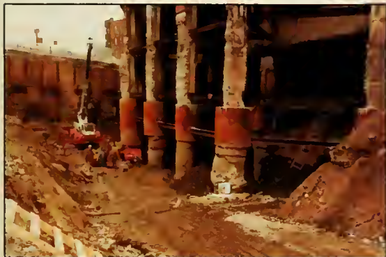
Heath Building Underpinning
