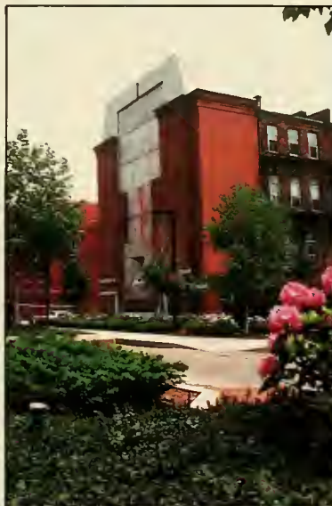
Yarmouth St. Ventilation Shaft
