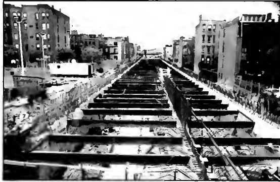
Temporary Bracing—Slurry Wall
