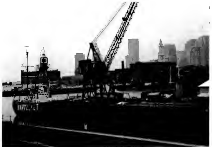
Existing Pier Features
