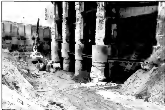
Heath Building Underpinning
