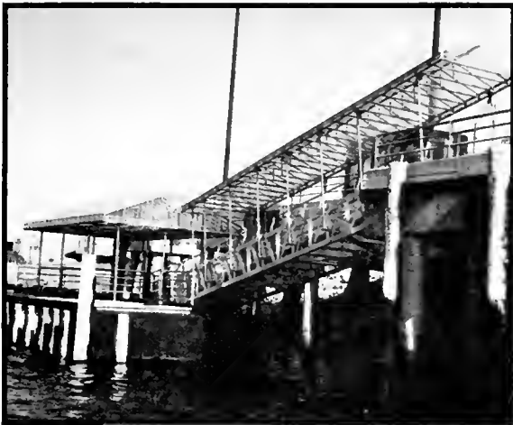
Gangway, Float, and Canopy
