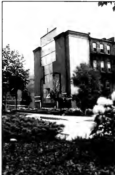
Yarmouth St. Ventilation Shaft
