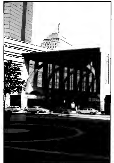
Back Bay Station
