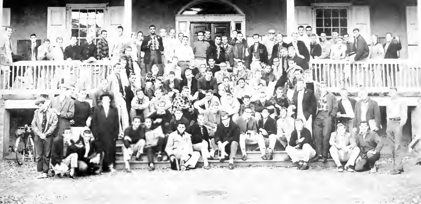
A study in disaster: The unsuspecting sophomore class was photographed just before the collapse of the Founders porch.
