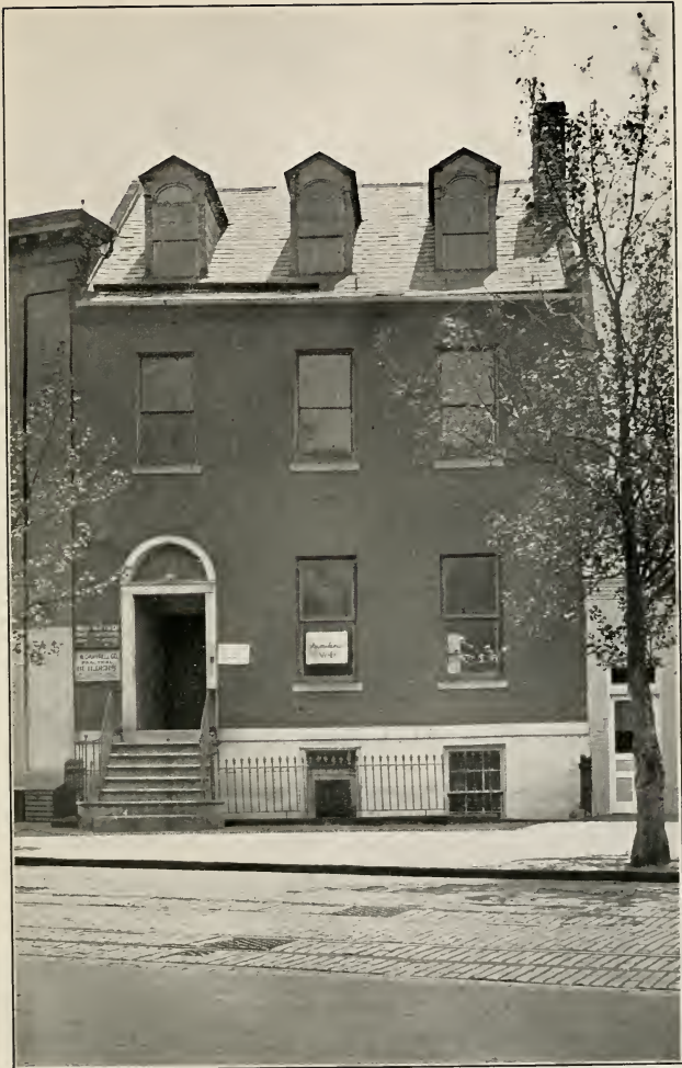
RESIDENCE OF RICHARD WALLACH, 456 LOUISIANA AVENUE.
