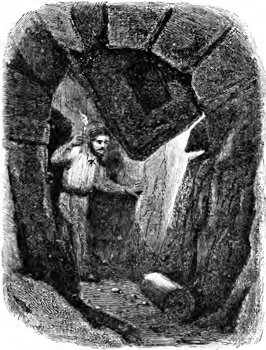
VOUSSOIR OF AN ARCH FALLEN THROUGH ROOF OF ROCK-CUT CANAL.
