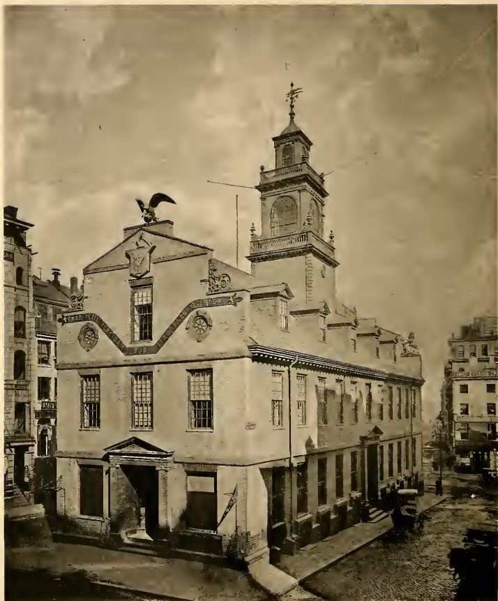
OLD STATE HOUSE. WEST END, 1883
